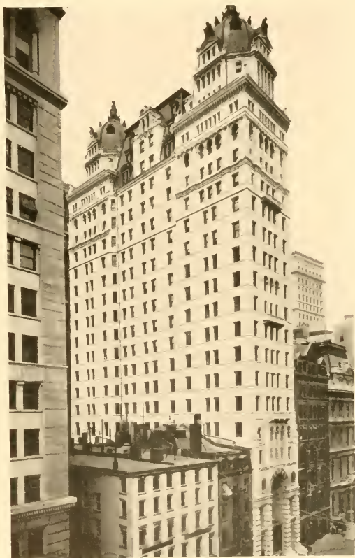
COMMERCIAL CABLE BUILDING. Adjoins the Stock Exchange at 20 Broad Street. An imposing office building given over to the business of the Commercial Cable system organized in 1884 by John W. Mackay and James Gordon Bennett. The offices of the Postal Telegraph-Cable, the German and Pacific cables are here.
