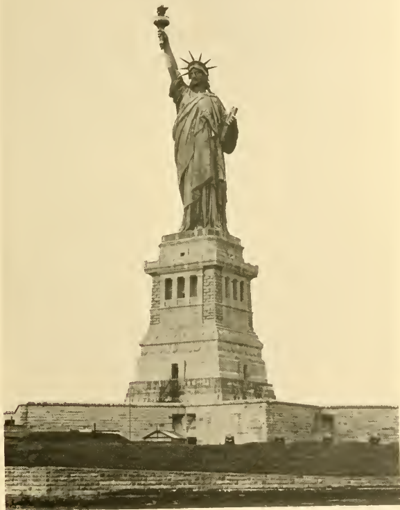
THE BARTHOLDI STATUE stands upon Bedloe's Island, almost two miles southeast of the Battery. This colossal figure, representing Liberty Enlightening the World was presented to the people of America by the great French sculptor, Auguste Bartholdi. It was erected in 1886. The torch is 306 feet above the sea.
