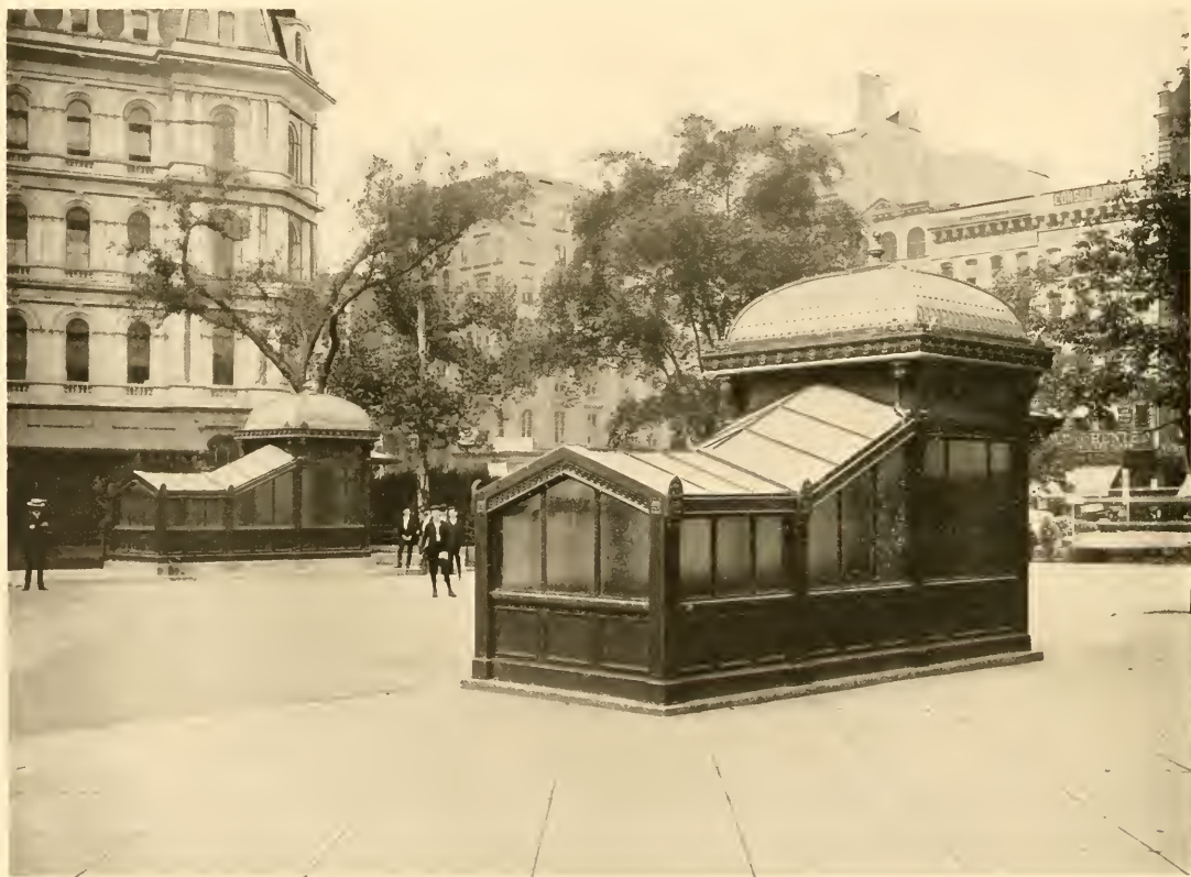
SUBWAY ENTRANCE, CITY HALL. The entrances and exits to the city's underground rapid transit system are a new feature of the streets of the metropolis. They are substantially built and of a pleasing design. The hereunto undertaking was completed in 1904. Ultimate cost, $21,000,000. Brooklyn Bridge is the terminal for all lines. Manhattan western section runs to Kingsbridge, eastern to Bronx Park. Brooklyn tunnel will pass under Broadway to South Ferry, thence under East River to Atlantic and Flatbush Avenues. Manhattan and Bronx lines reach Yonkers and Williamsbridge. Various branches and loop-lines connect the sections.
