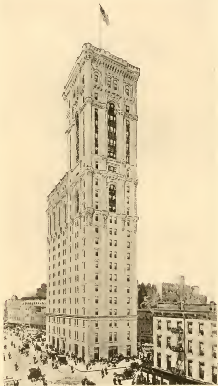
NEW YORK TIMES BUILDING. At Broadway, 7th Avenue and 43d Street. The new home of the great newspaper, built especially to meet the requirements of modern journalism. It is a stately structure of 22 stories; rises 375 feet above and extends 55 feet below the sidewalk. A Subway station is in the basement.
