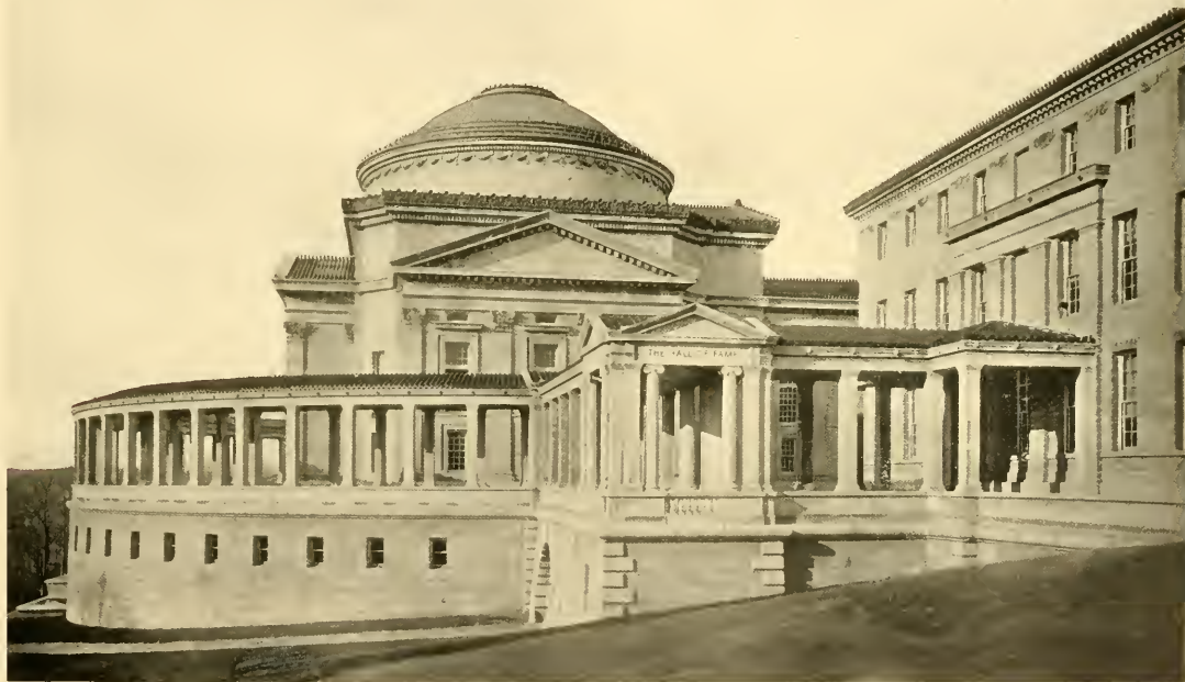
THE HALL OF FAME FOR GREAT AMERICANS, University Heights at Sedgwick, Aqueduct and University Avenues and East 181st Street. This semi-circular structure, over 500 feet long, is a striking feature of the New York University, the library of which institution it half-surrounds. It contains 150 eight-foot panels which will ultimately be inscribed with the names of departed great Americans. The first five names selected were: Washington, Lincoln, Webster, Franklin and Grant. The building cost $250,000 and was the gift of Miss Helen Gould to the University.
