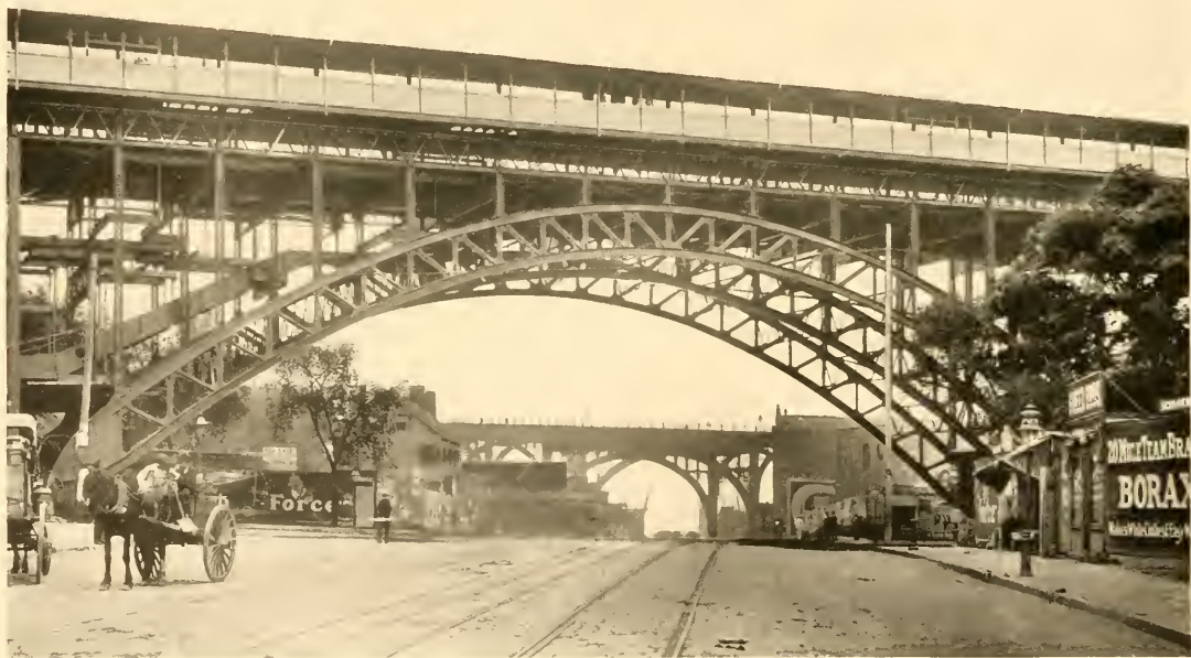
MANHATTAN VIADUCT, Manhattanville. At 125th Street the West Side line of the underground rapid transit system emerges from the subway and crosses the Manhattan valley on a great flying-arch-steel viaduct to 135th Street, where it again enters the tunnel, and at 190th Street is more than 100 feet below the surface. The Manhattan Viaduct is a splendid example of American bridgework, and in common with all sections of this greatest engineering feat of the new century, is built to last for all time under the severest strain.
