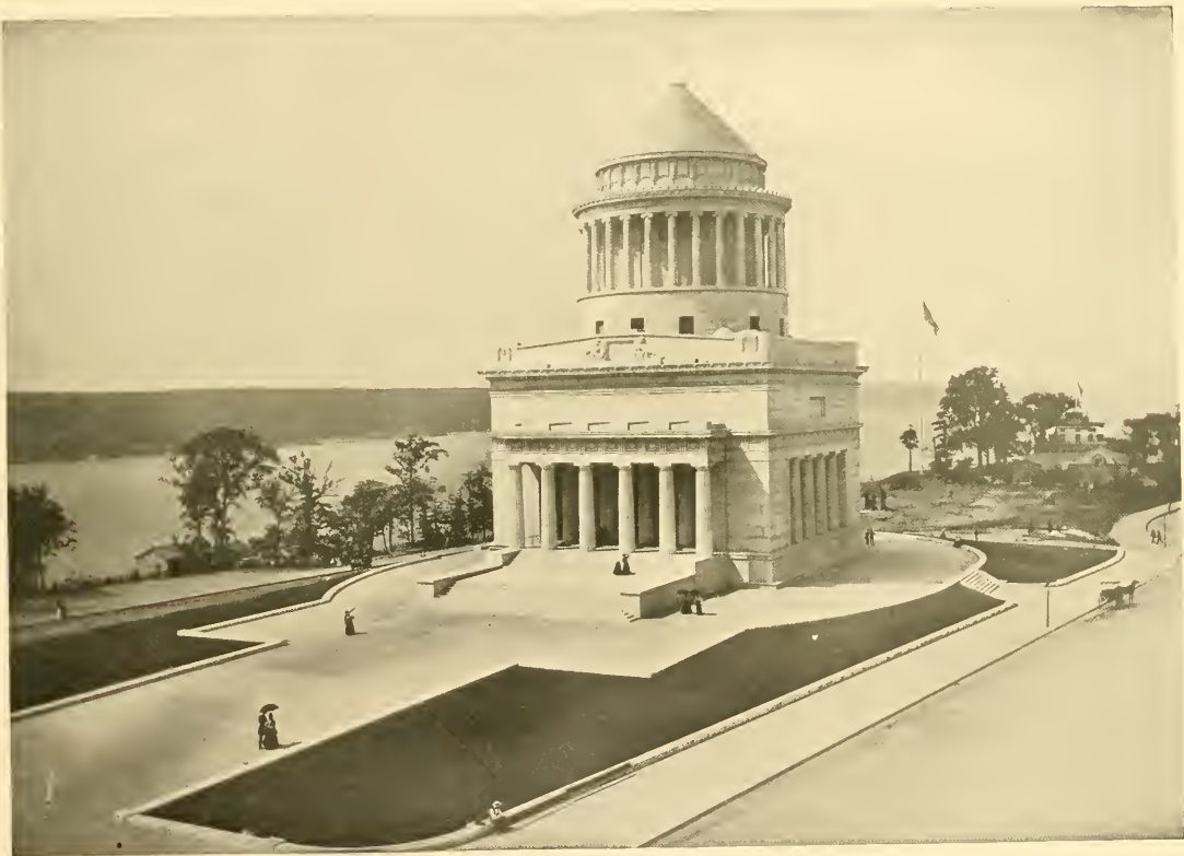
GRANT'S TOMB. Claremont Heights, Riverside Drive, near 123d Street. This beautiful edifice, one of the largest monuments in the world, is 150 feet high and covers an area of 10,000 square feet, and is built of Maine white granite. The cost, $600,000, was raised by the Grant Monument Association by voluntary contributions from over 30,000 people. The memorial was dedicated by President McKinley in 1897. Over the portico are statues of "Peace" and "Victory" by J. Massey Rhind. The remains of the great soldier and his wife lie in two red porphyry sarcophagi in a crypt under the dome.
