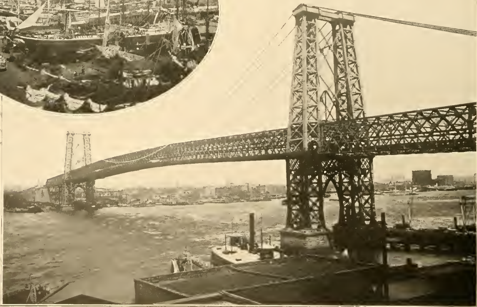
THE WILLIAMSBURG BRIDGE, the greatest suspension bridge in the world, crosses the East River at the Grand Street Ferry to Broadway (Williamsburg) Brooklyn. It is a steel-towered suspension-cantilever structure with a length of 7,300 feet between terminals. The towers are 335 feet high. The central span is 1,000 feet long and 135 feet above the middle of the river. The bridgeway is 118 feet wide, and carries four trolley and two cable tracks, two roadways, two foot-paths, and two bicycle paths. Estimated cost, about $21,000,000.
