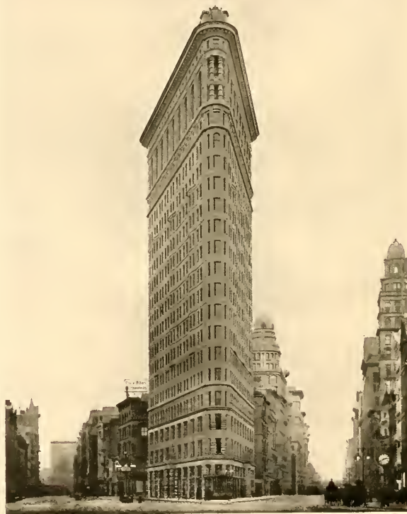
THE FULLER BUILDING, known popularly as "the "Flat-iron," is located on Broadway at the intersection of 23d Street and 5th Avenue. It has 20 stories and is 286 feet high. Its remarkable shape and conspicuous position have made it one of the best known buildings in the country.
