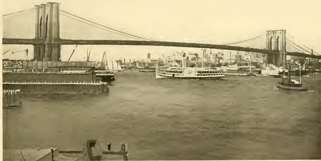
THE BROOKLYN BRIDGE. Stretches from opposite City Hall Park to Fulton and Sand Streets, Brooklyn. This magnificent bridge was begun in 1870 and opened to the public in 1883. Cost, $21,000,000. It consists of a central river span 1,595 feet long and two land spans, with a total length between terminals of 7,580 feet. The bridgeway carries two cable and two trolley car tracks, two wagon ways and a footpath. 4,000 cars and 2,000 vehicles pass east and west every day. The average number of passengers in twenty-four hours is 300,000. It is estimated that about 5,000,000,000 people have used this bridge since its opening.
