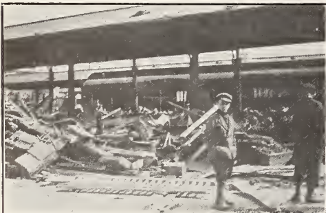
Depot Union Station, Dayton.
