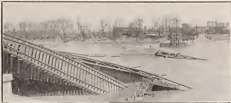
Wreck of Modern Bridge in Dayton.
