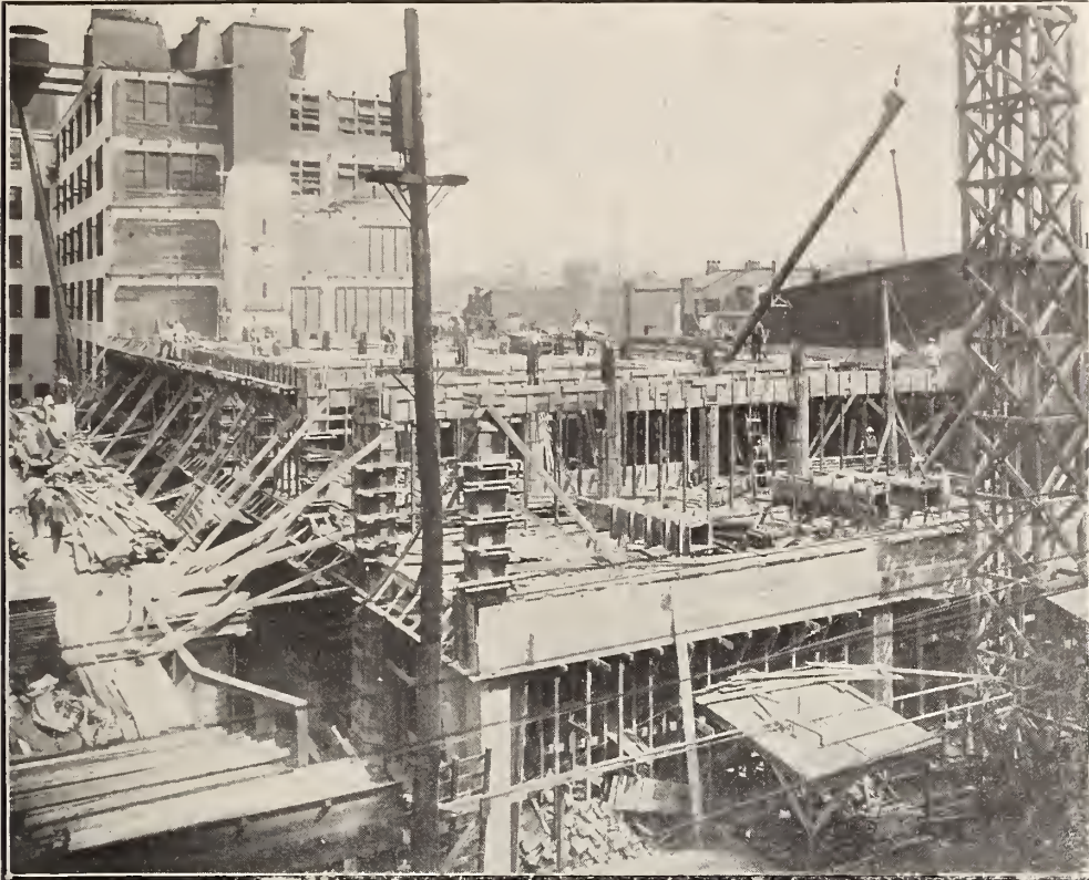
Progress of Work on Addition to Victor Factories.
