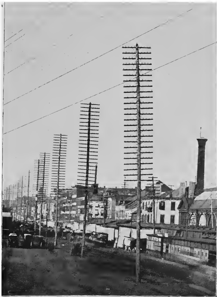
HEAVY POLE LINE CONSTRUCTION, WEST STREET, NEW YORK.
