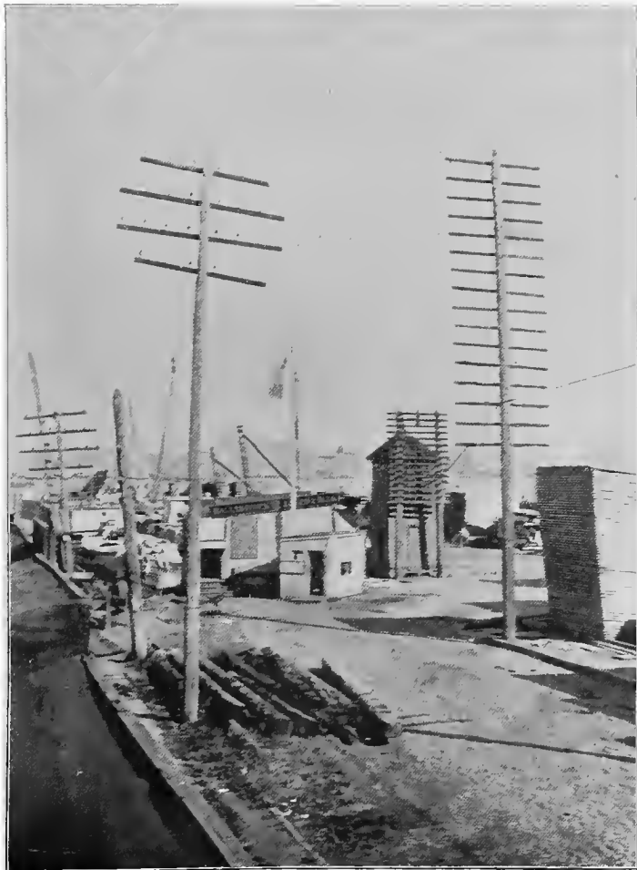
NORTH RIVER CABLE TERMINAL, NEW YORK END.
