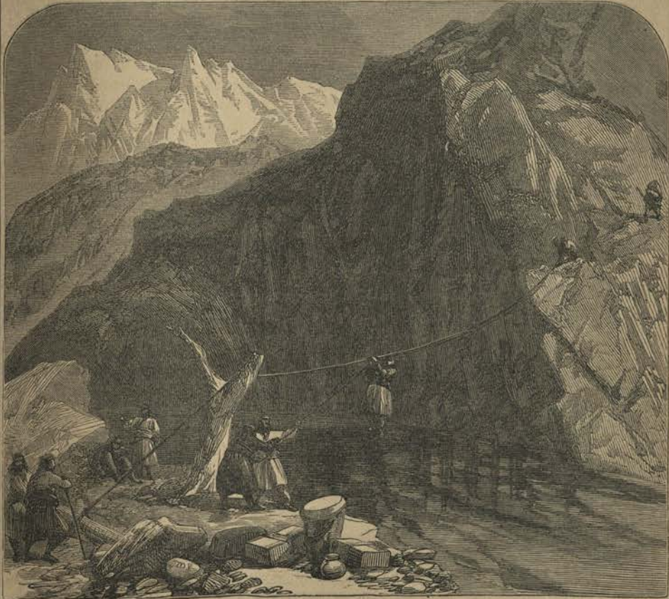
Rope Bridge over the Spiti Torrent.
