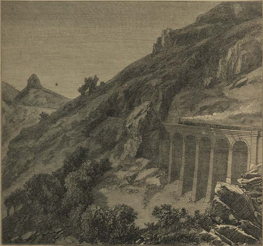
Viaduct on the Bhor Ghaut Incline.
