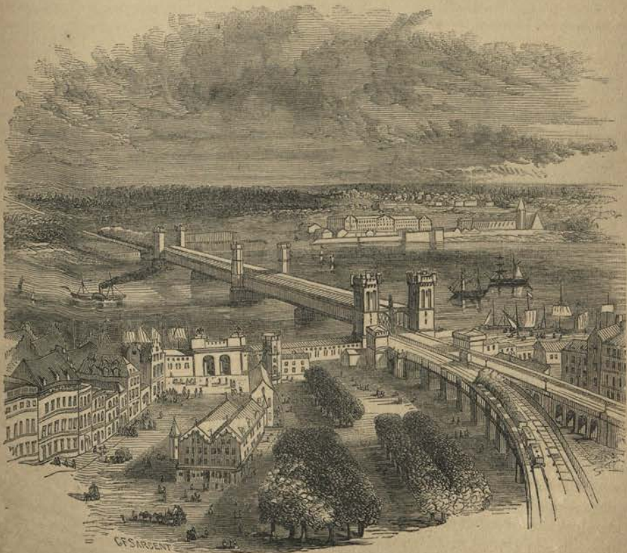
Railway Bridge at Cologne.
