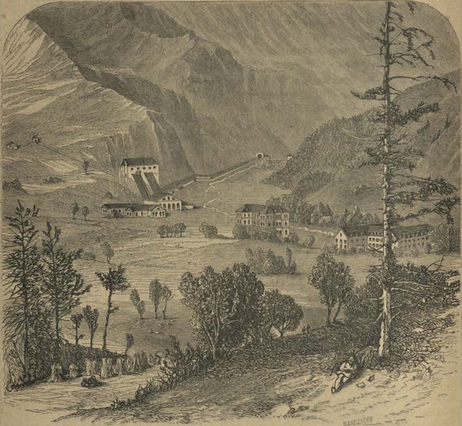
Bardonnèche Mouth of the Mount Cenis Tunnel.
