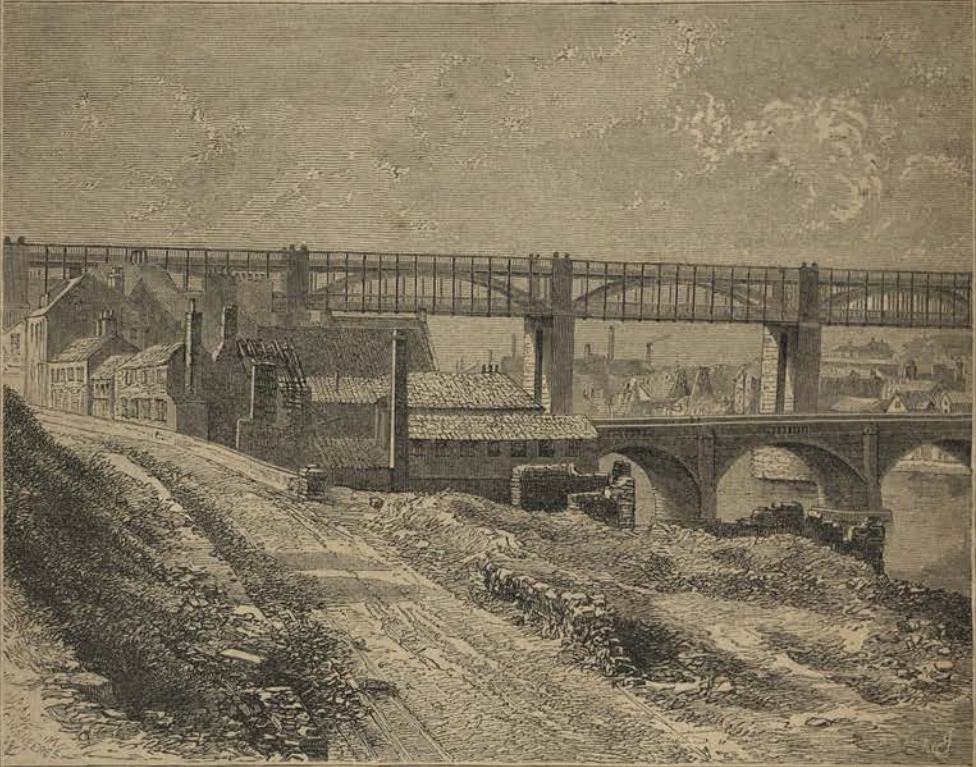
High and Low Level Bridges,
