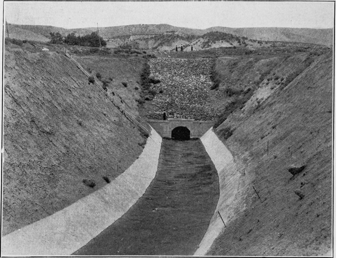
DOWN STREAM END OF SIX-MILE TUNNEL IN UNCOMPAGRE VALLEY
