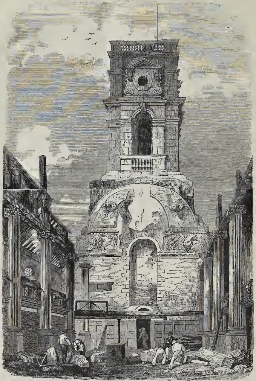
INTERIOR VIEW OF ST. OLAVE'S CHURCH, SOUTHWARK, AFTER THE LATE FIRE.
