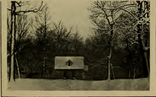
FIRST BUILDING OF THE SEABURY MISSION
