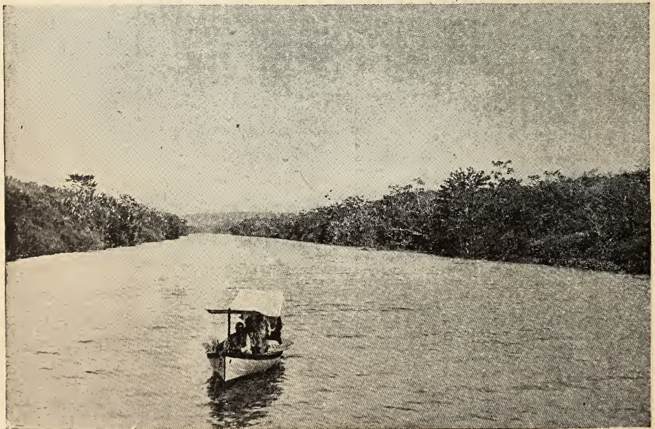
PANAMA CANAL. 9 MILES FROM COLCN.
