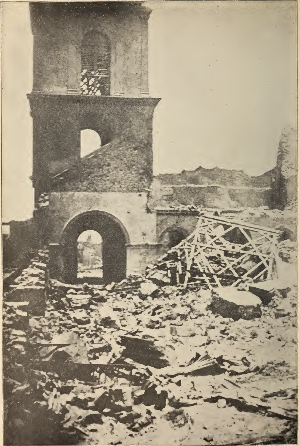
INTERIOR OF CATHEDRAL AT ST. PIERRE, Showing Wreckage of Bell and Frame-work on the Ground. Remainder of Church Entirely Destroyed.—(Copyright, May 21, 1902, by The Press Publishing Company—New York World.)
