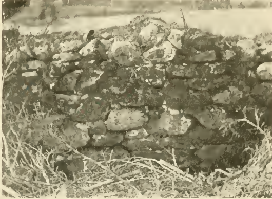
OLD WALL IN A CELLAR IN FORT WILLIAM HENRY, MAINE.
