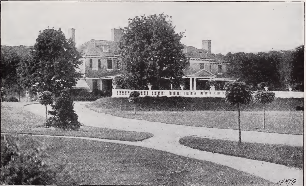
Large Norway Maples moved by Hicks Patent Tree-Mover to the residence of the late Charles Albert Stevens, Wheatley Hills, L. I. We can supply trees of this type for immediate effect. Catalpa Bungei in the foreground.
