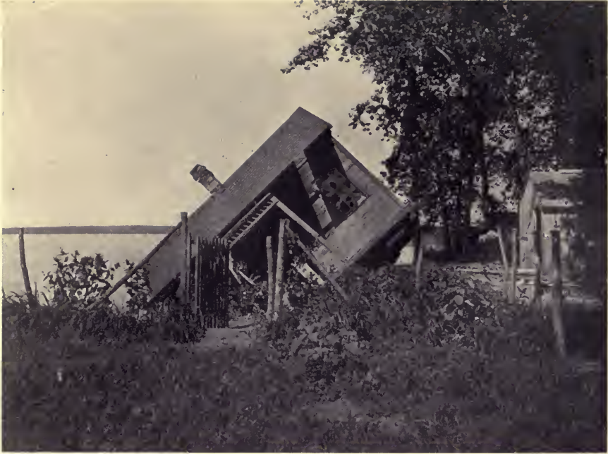
No. 5. Next Morning—the Remainder of the House Falls in.
