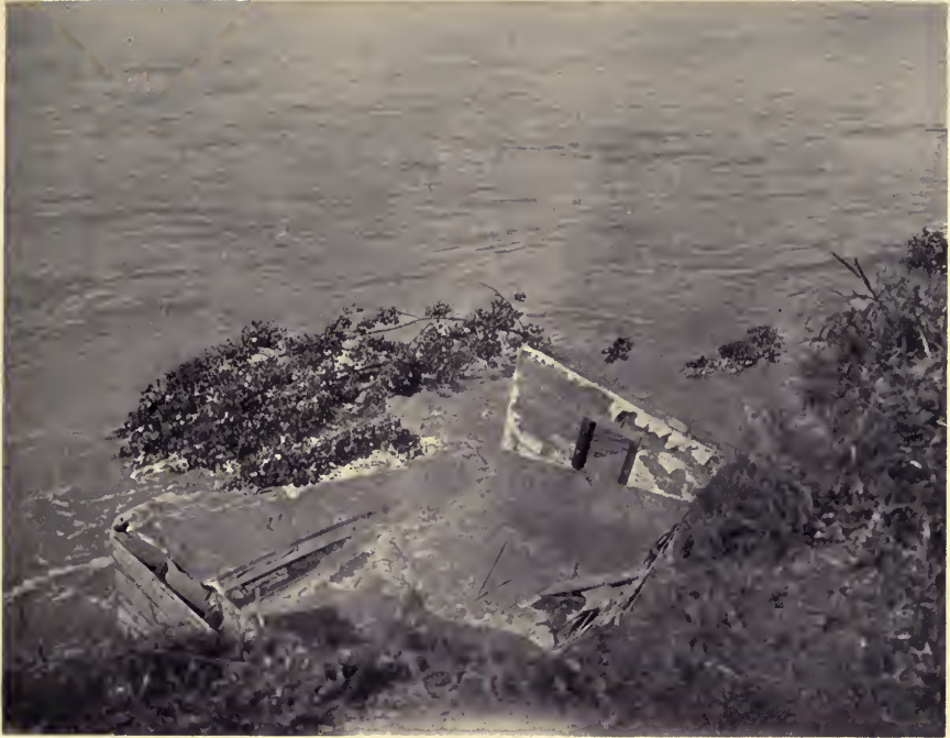
No. 3. The Undermined Wing Falls into the Stream.
