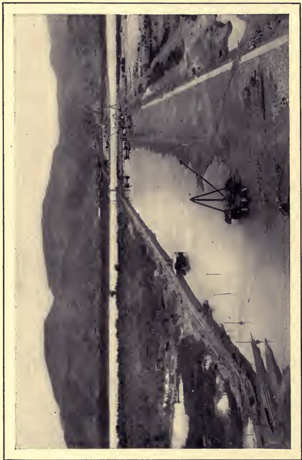
Work on Laguna Dam, Yuma Irrigation Project, Arizona and California.
