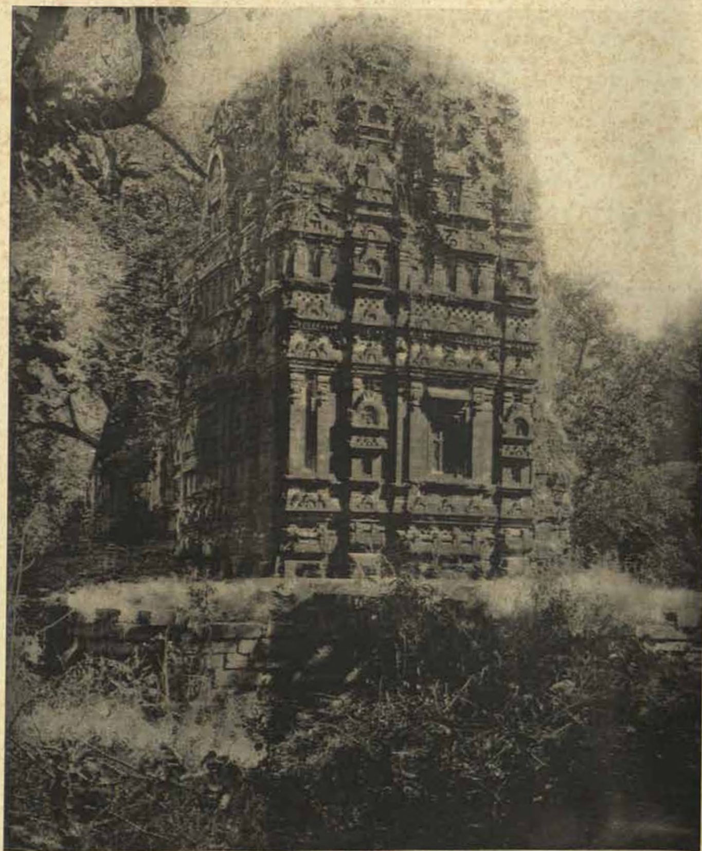
TEMPLE OF LAKSHMANA AT SIRPUR. SIDE VIEW FROM NORTH-WEST, BEFORE REPAIRS.
