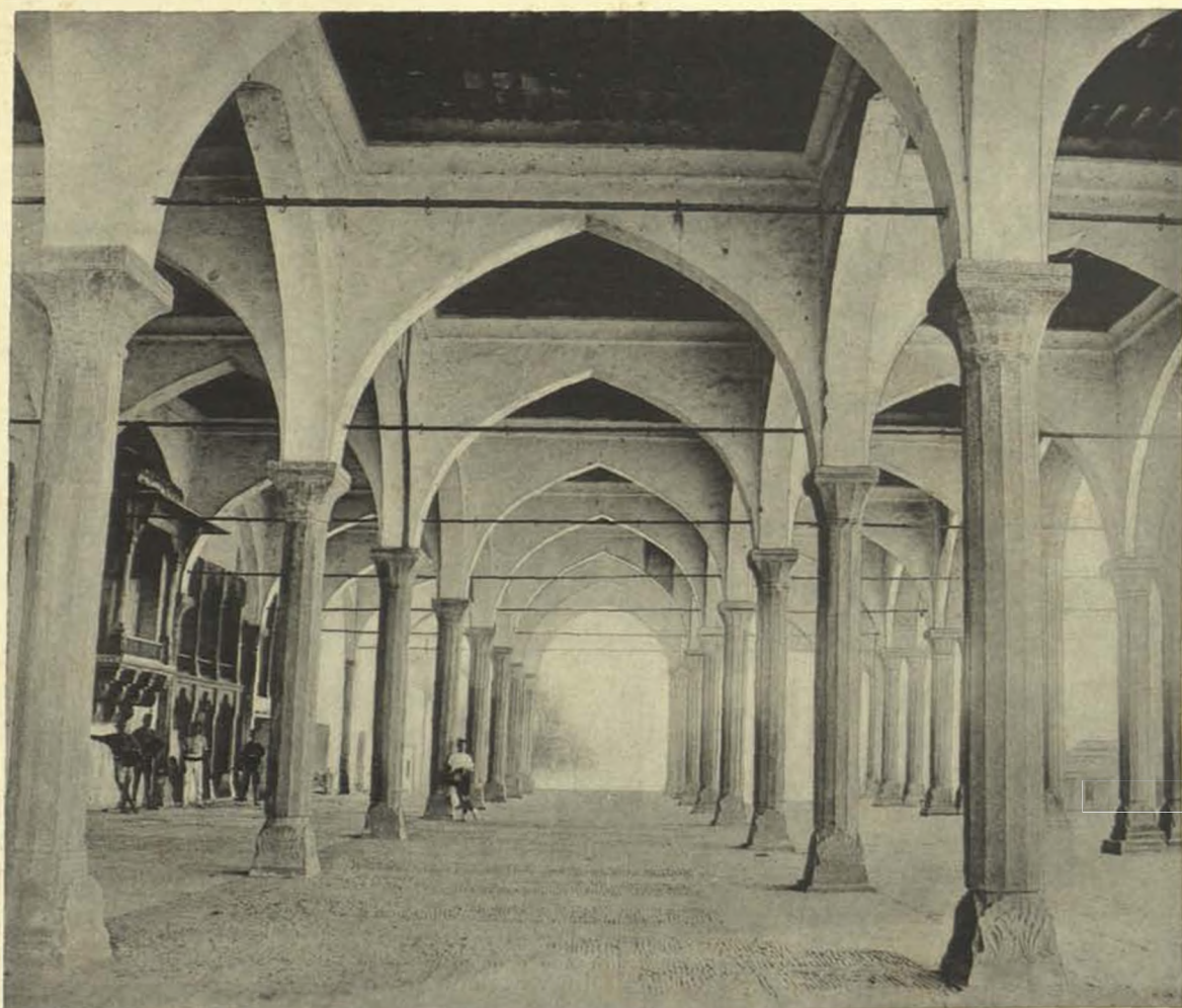
(b) VIEW FROM WEST; AFTER REMOVAL OF MODERN ADDITIONS FROM THE THRONE AND PILLARS.
