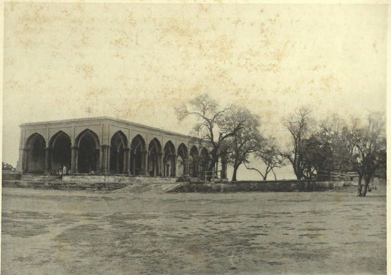
(b) VIEW FROM WEST; AFTER REMOVAL OF MODERN ADDITIONS.
