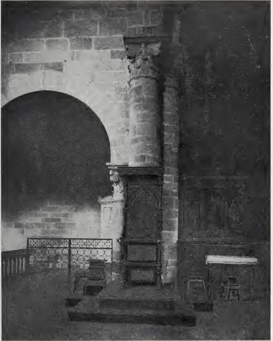
FIG. 4.—A PIER IN THE CATHEDRAL OF FIESOLE. Showing the entasis in profile.
