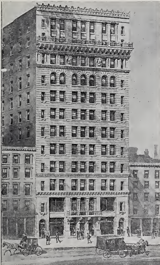
THE FRANKLIN BUILDING. Nos. 11 to 15 Murray Street, New York City. Clinton & Russell, Architects.
