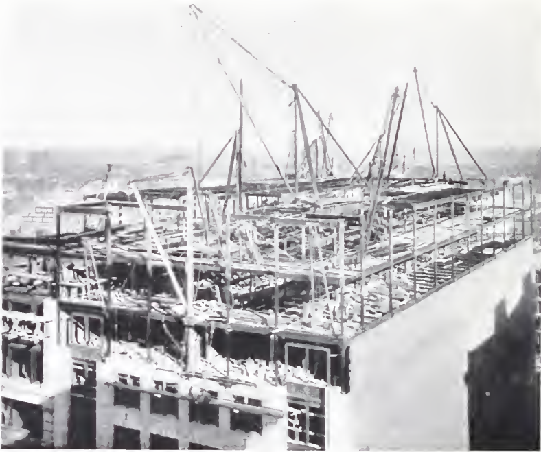
BIRD'S-EYE VIEW NEW TWELVE STORY BUILDINGS, 594-596 BROADWAY, SHOWING ERECTING PLANT.
