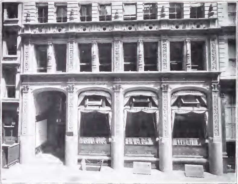
ENTRANCE OF FAHYS BUILDING.
