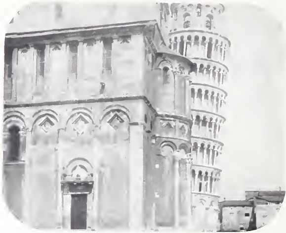
FIG. 2.—THE LEANING TOWER OF PISA.
