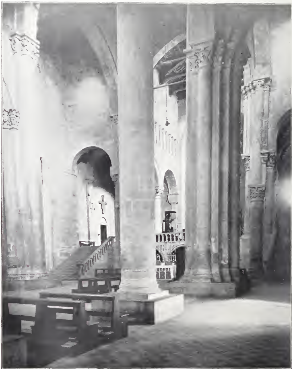
FIG. II. THE LEANING PIERS OF S. MARIA DELLA PIEVE AT AREZZO. Accurately photographed. Compare Figs. 10, 12.
