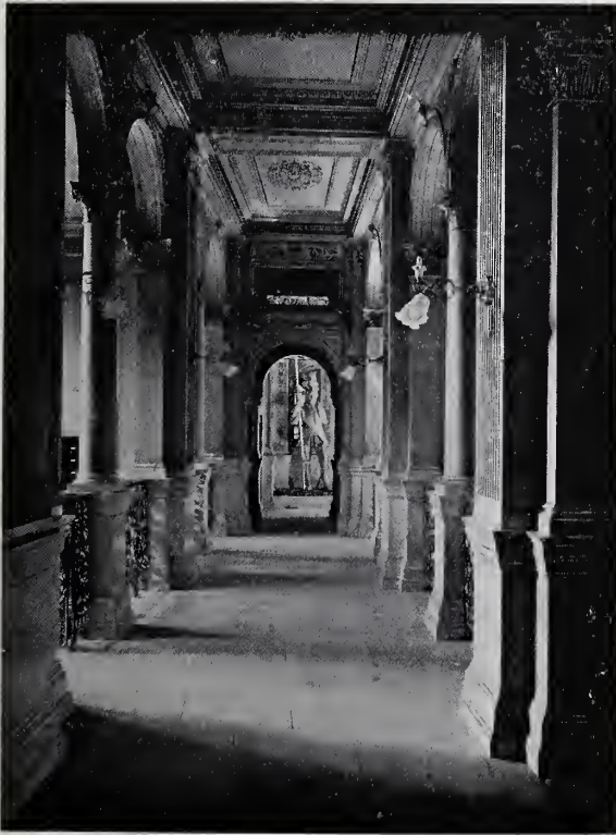
CORRIDOR, MUTUAL LIFE INSURANCE BUILDING.
