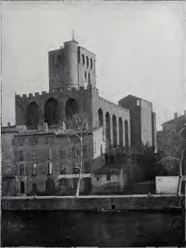
AGDE CATHEDRAL—VIEW FROM THE SOUTHWEST.
