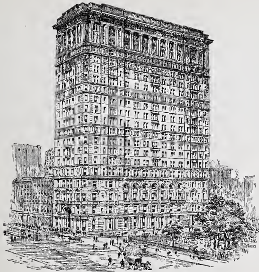
EMPIRE BUILDING, Broadway and Rector Street. Kimball & Thompson, Architects.
