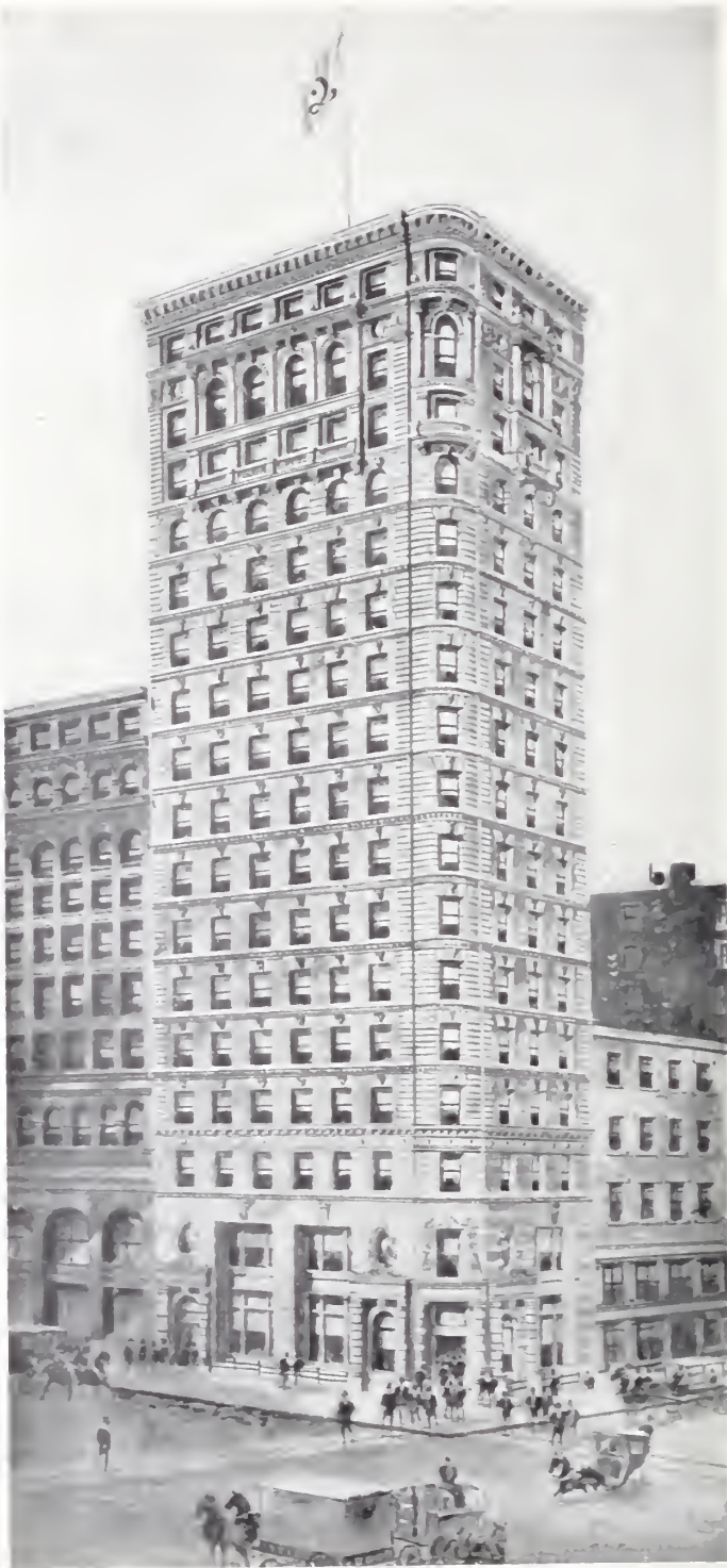
QUEENS INSURANCE CO.'S BUILDING.
