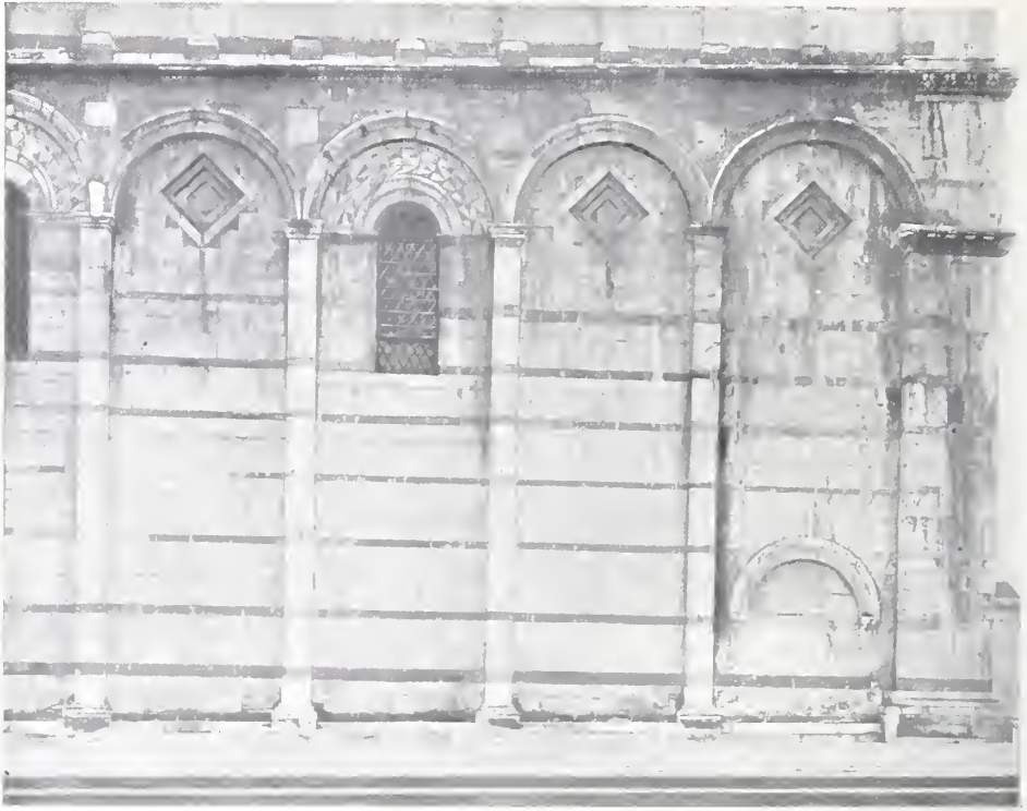
FIG. 9.—PISA CATHEDRAL NORTH WALL AND LEANING FACADE.
