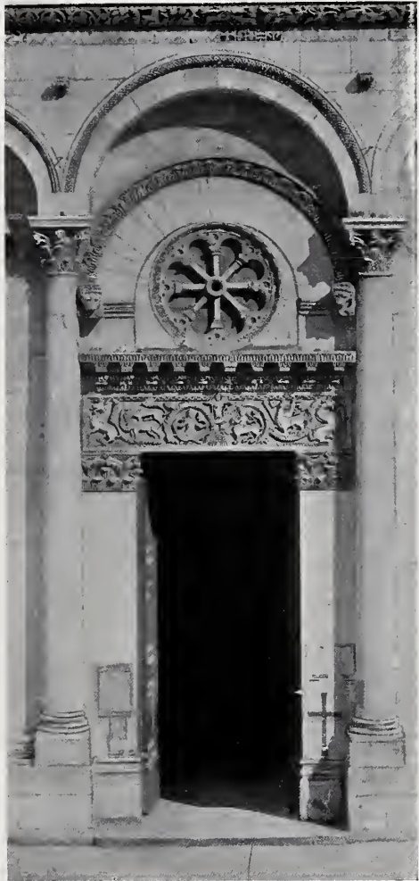
FIG. 3.—DETAIL OF FACADE, S. MICHELE, LUCCA. The engaged mediaeval columns have an entasis.
