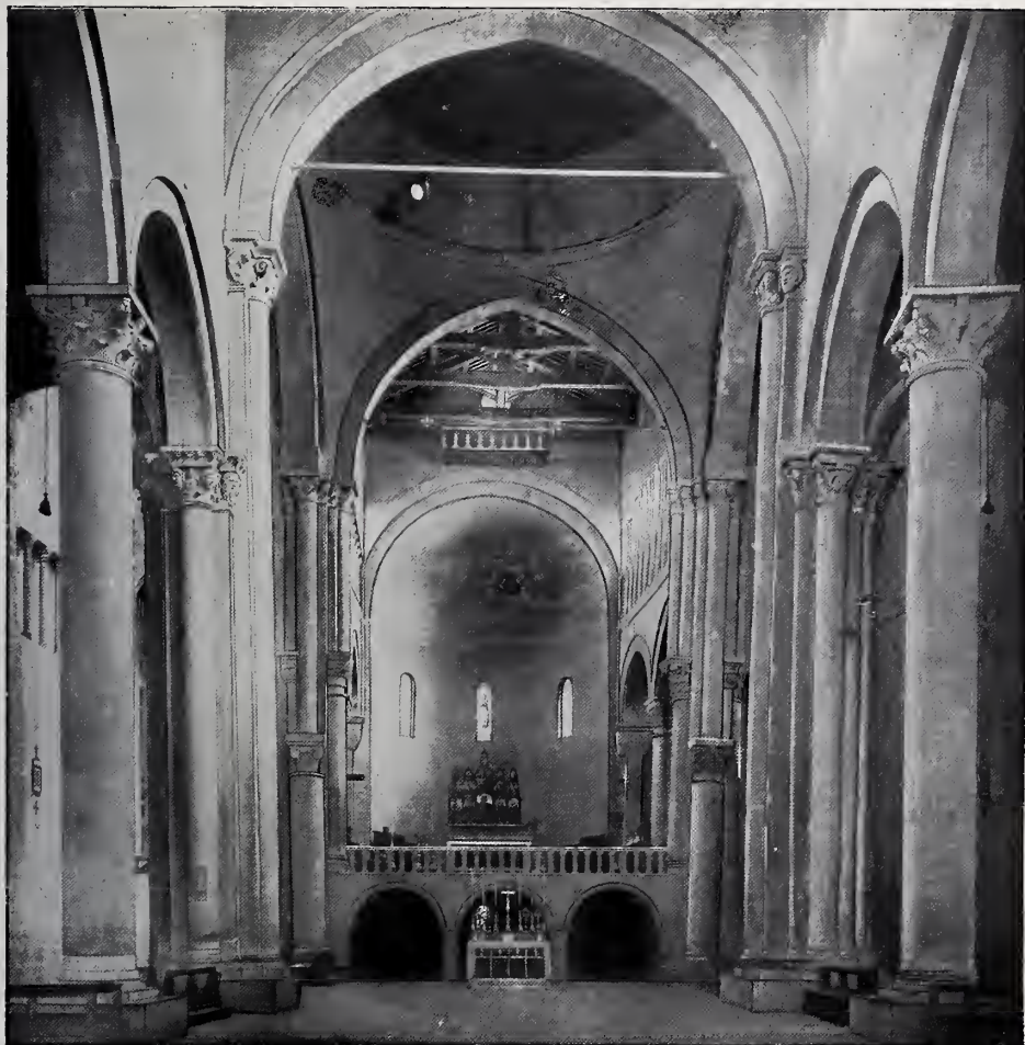
FIG. 10. THE LEANING PIERS OF S. MARIA DELLA PIEVE AT AREZZO. Accurately photographed. Compare Figs. 11, 12.
