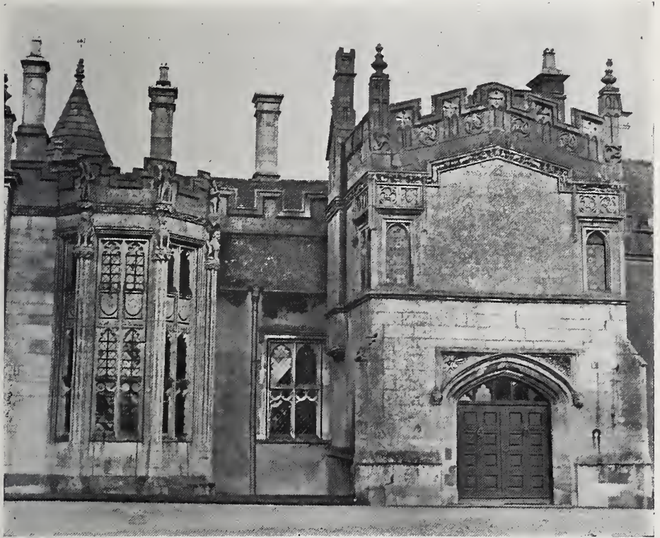
FRONT DOOR AND OLD STONE WINDOW.
