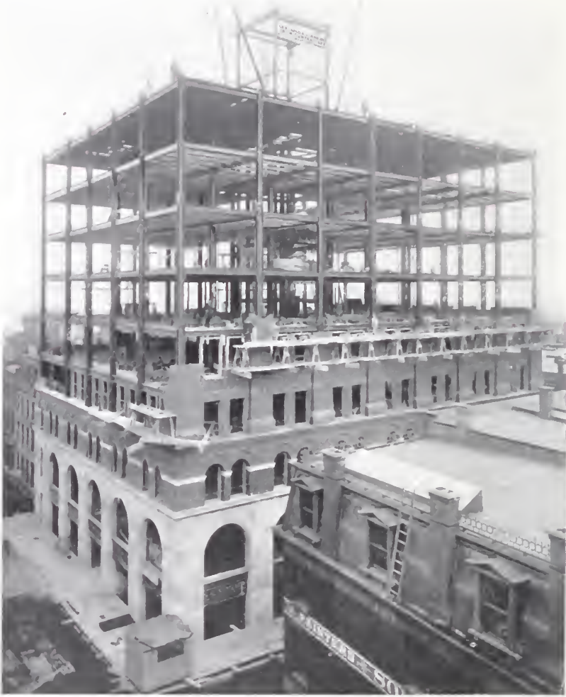
THE WOODBRIDGE BUILDING IN PROCESS OF CONSTRUCTION.
