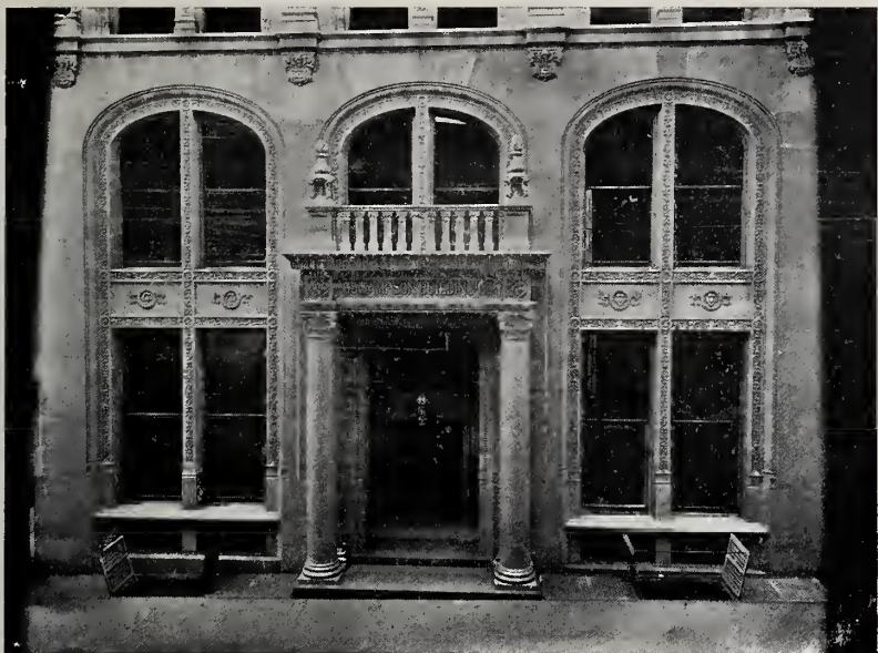
DETAIL OF THE SAMPSON BUILDING.
