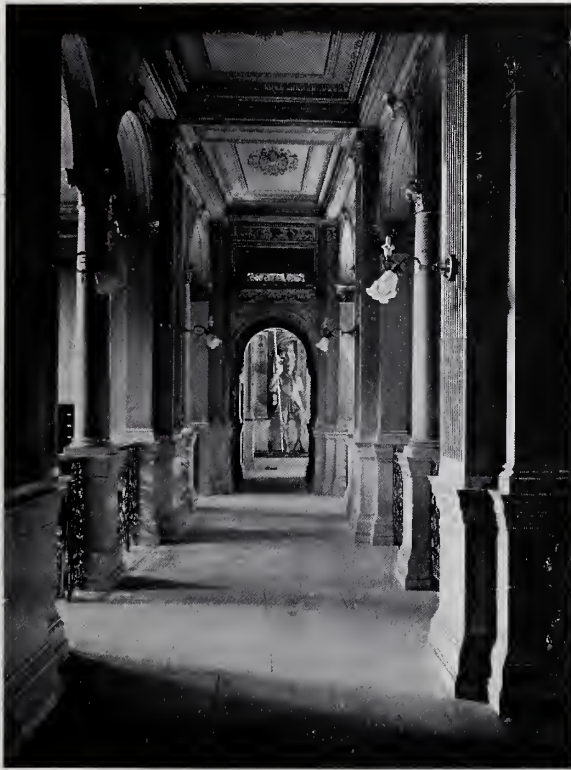
CORRIDOR, MUTUAL LIFE INSURANCE BUILDING.
