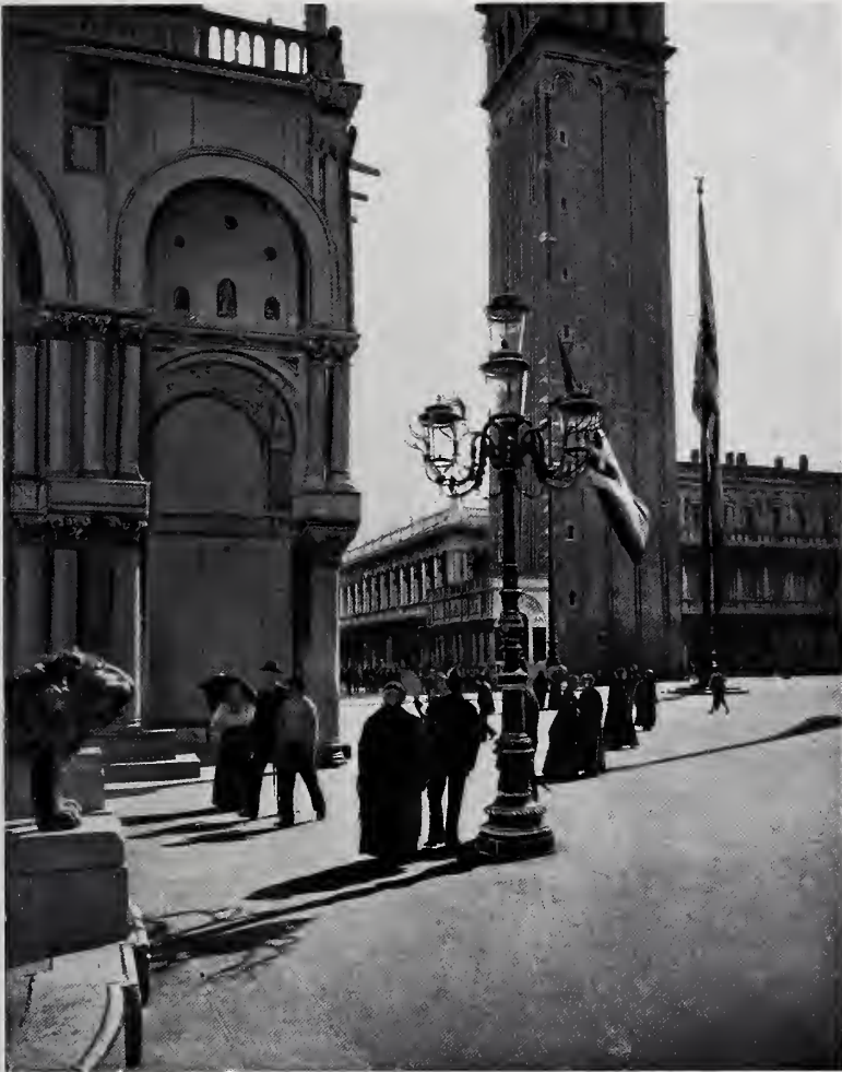
FIG. 16.—NORTHWEST ANGLE OF S. MARK'S, VENICE. Showing a delicate forward lean and return bend.
