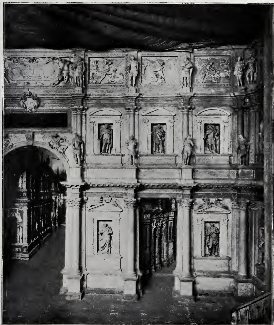
FIG. 16.—PORTION OF THE STAGE SETTING, TEATRO OLIMPICO, VICENZA. Showing Palladio's use of the entasis in all columns and pilasters. Compare Fig. 15.
