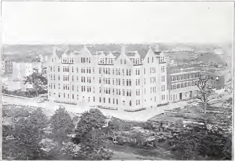
FIG. 8.—SCHOOL AT EDGEComb AVENUE BETWEEN 140TH AND 141ST STREETS.
