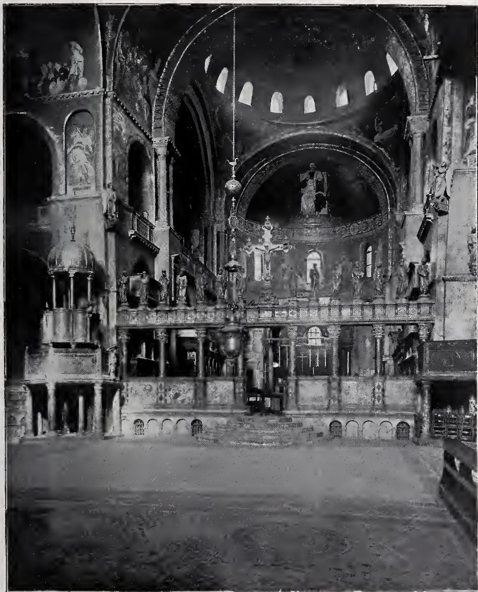
FIG. 4. NAVE OF S. MARK'S AT VENICE. Showing outward lean of the right pier.
