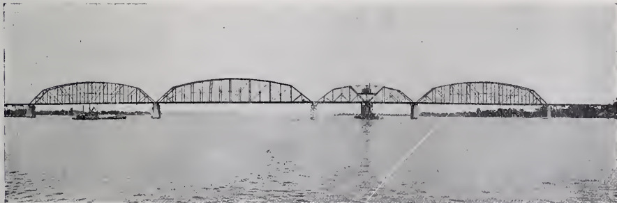
DELAWARE RIVER BRIDGE. Pennsylvania Railroad, Crossing the Delaware River at Frankford, Philadelphia, Pa.
