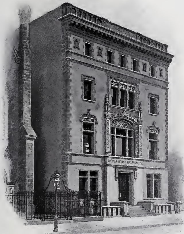
AMERICAN SOCIETY OF CIVIL ENGINEERS, Cyrus L. W. Edlitz, Architect. 220 West 57th Street, New York City.
