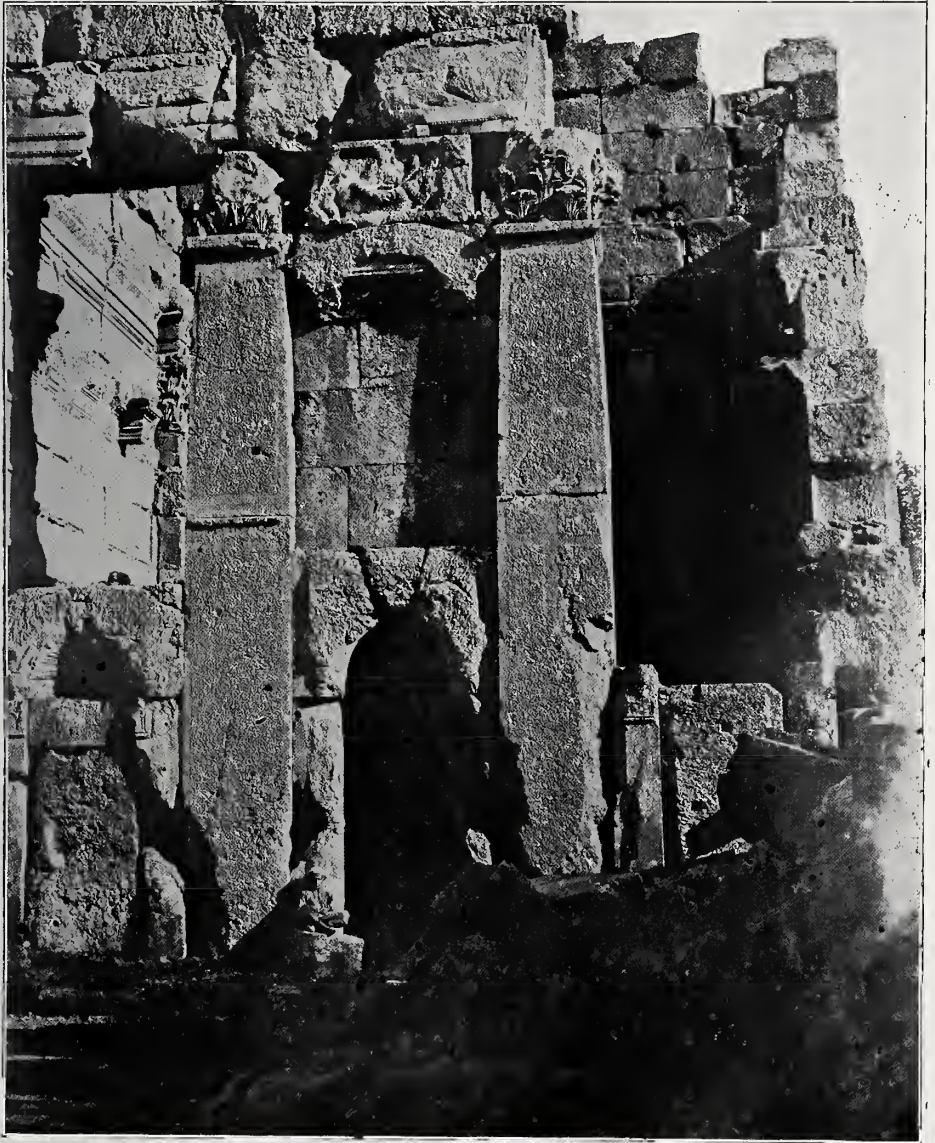
FIG. 17.—THE ENTASIS IN ROMAN PILASTERS AT BAALBEK, SYRIA. The date is second century of our era.
