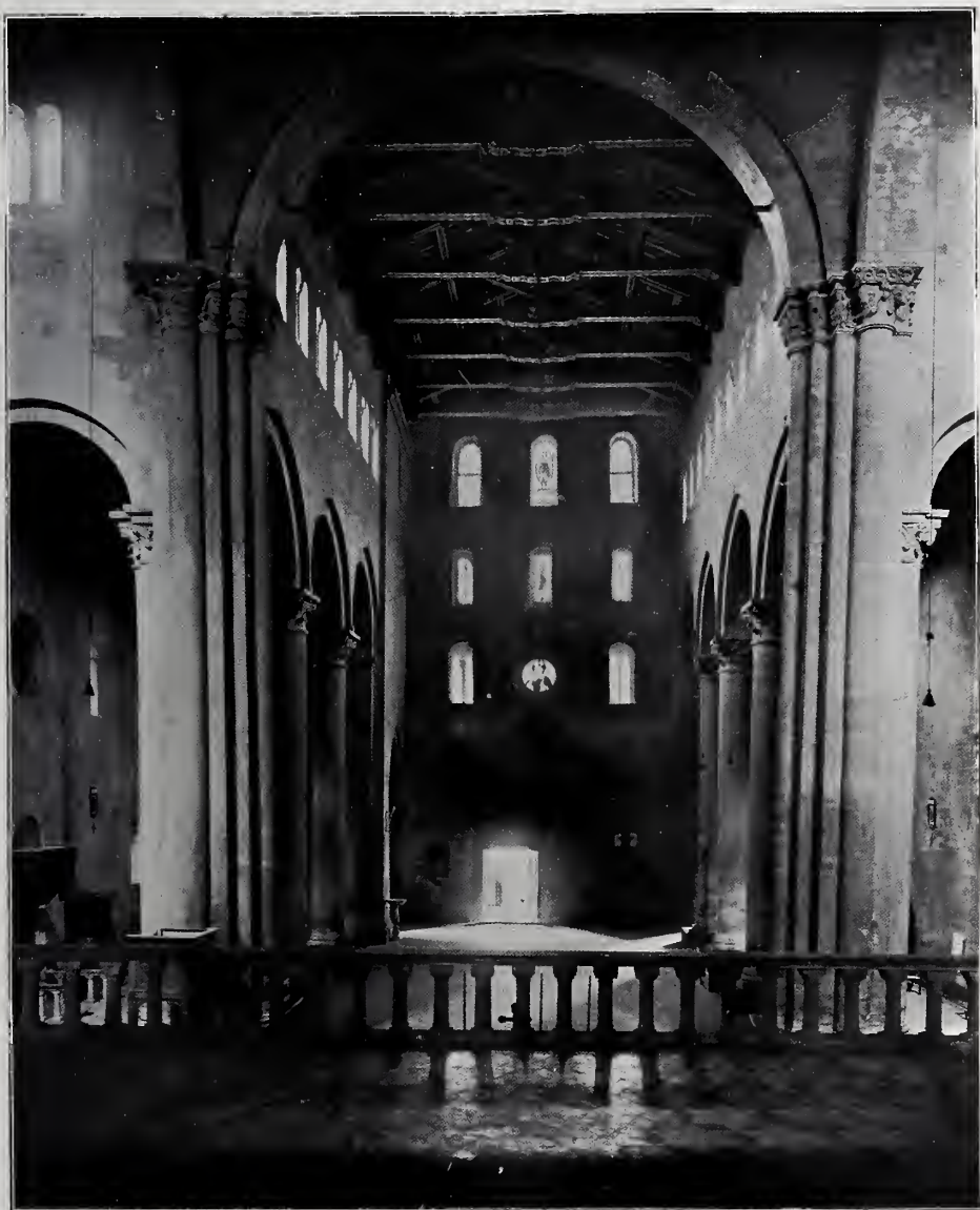
FIG. 12. THE LEANING PIERS OF S. MARIA DELLA PIEVE AT AREZZO. Accurately photographed. Compare Figs. 10, 11.
