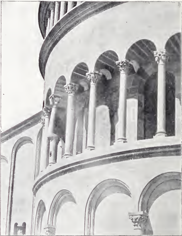
FIG. 19. CHOIR GALLERY OF S. MARIA DELLA PIEVE, AREZZO. Showing a bent column.
