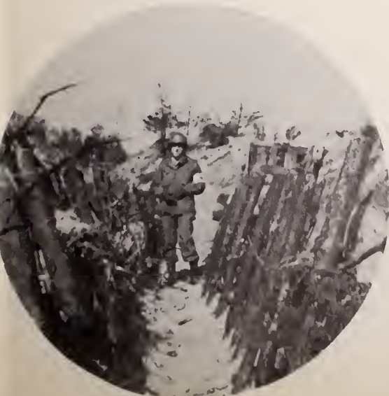
Trench—Frankfurt Race Track
