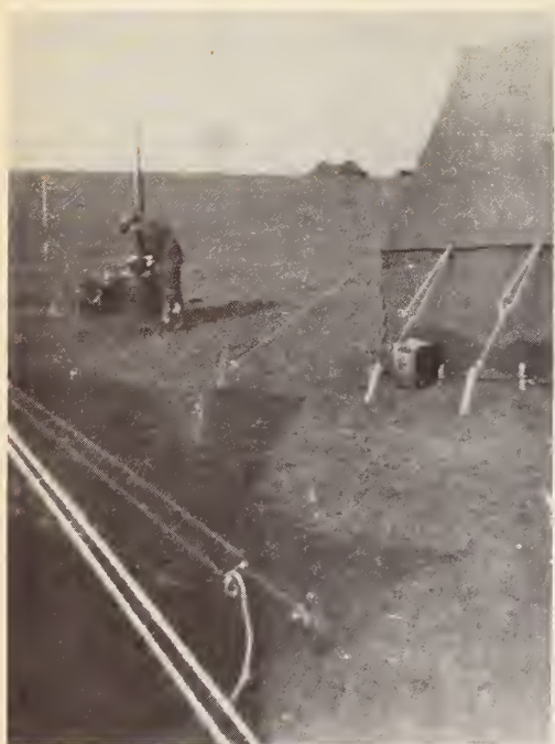
Hot water supply
