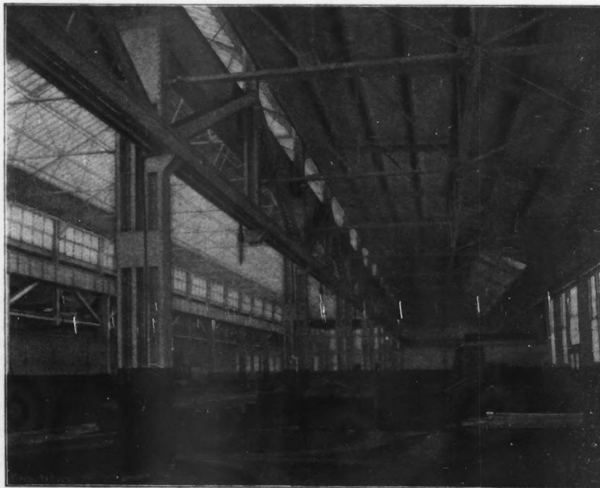
FIG. 2.—INTERIOR OF NEW IRON FOUNDRY, GENERAL ELECTRIC CO., SCHENECTADY, N. Y.
