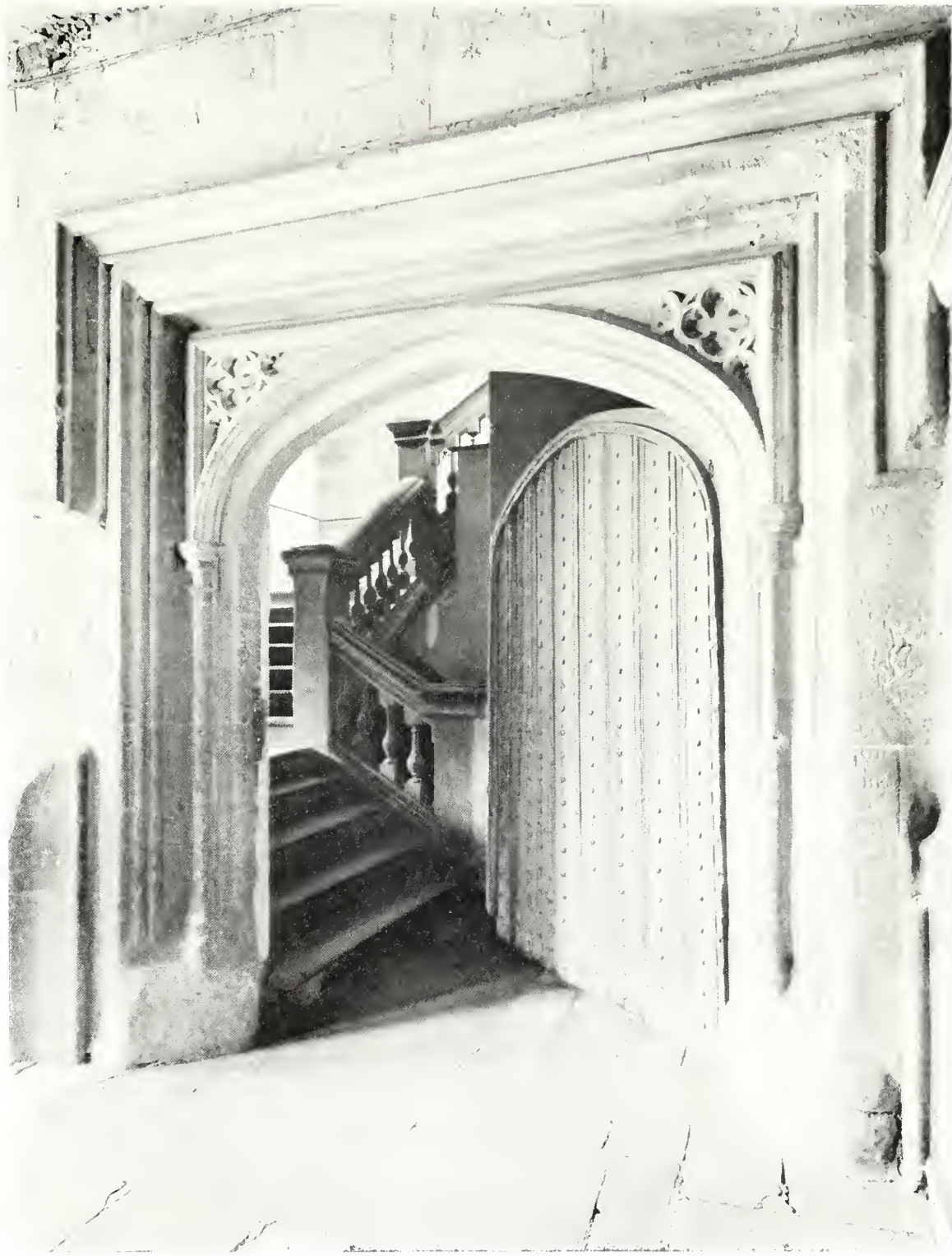
WAYNFLETE'S NORTH DOOR, WITH THE SEVENTEENTH-CENTURY STAIRS TO UPPER SCHOOL AND ANTECHAPEL.
