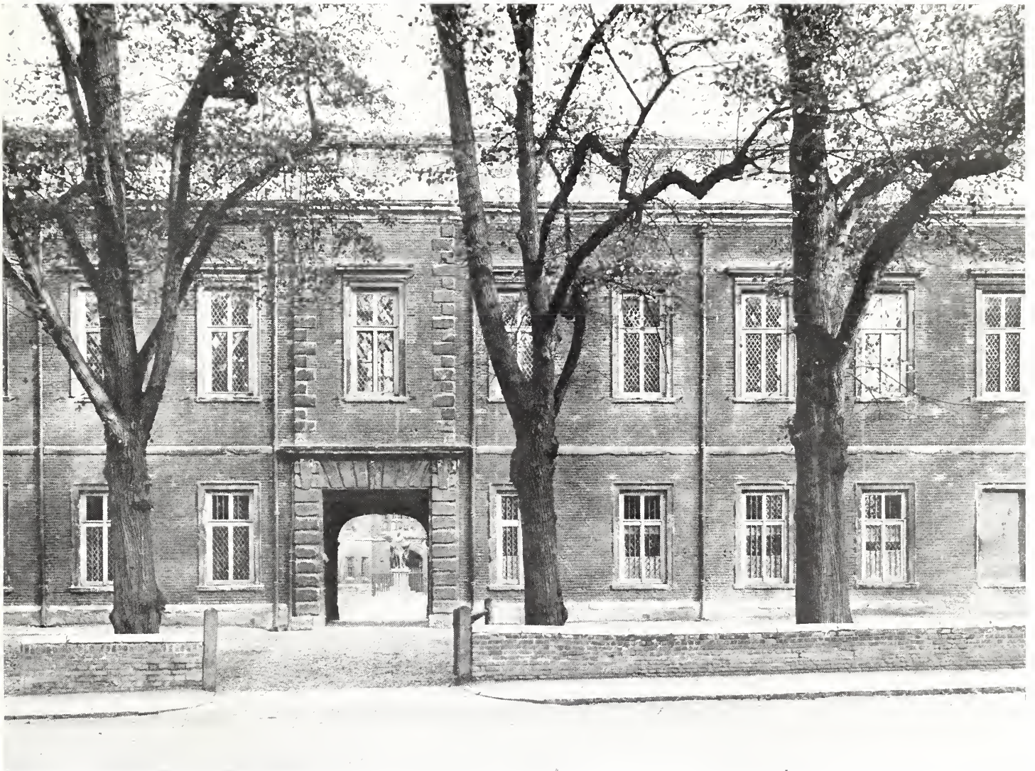
UPPER SCHOOL, LOOKING THROUGH INTO SCHOOL YARD.
