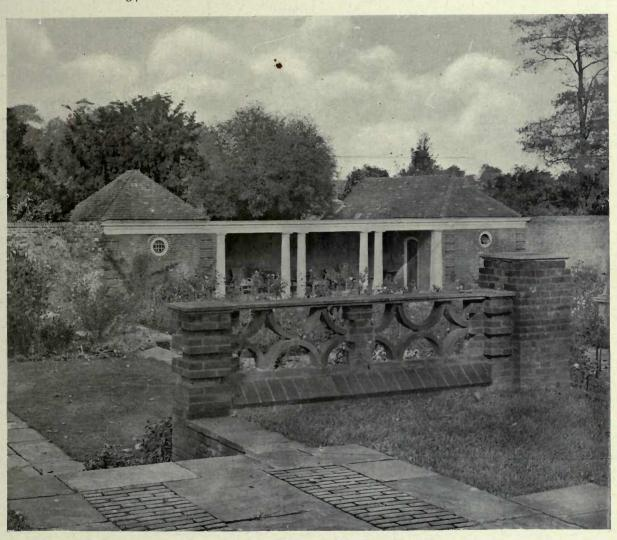
FIG 135.—OPEN PARAPET OF CURVED TILES.
