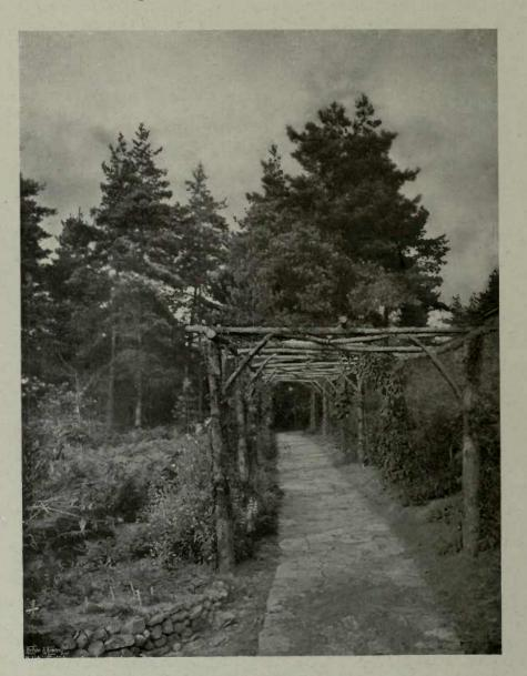
FIG. 258.—OF LARCH POLES WITH WELL-SHAPED BRACES.
