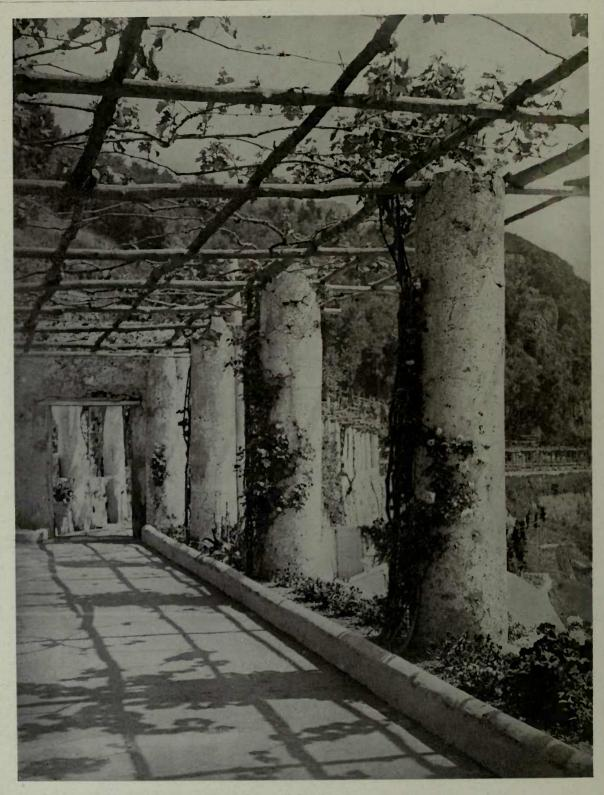
FIG. 256.—PIERS OF RUBBLE, PLASTERED, AT AMALFI.
