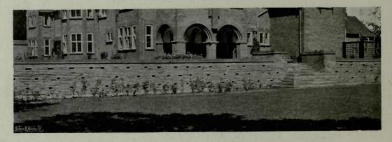
FIG. 162.—BRICK WALL WITH SPACES LEFT FOR PLANTS.
