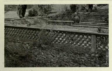
FIG. 134.—IN MOULDED BRICK.
