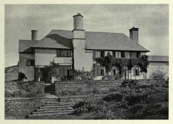
FIG. 155.—THIN SLATE STONES LAID LEVEL.
