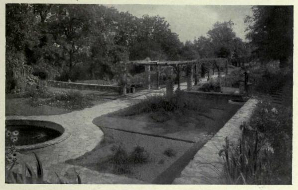
FIG. 244.—STONE PAVING WITH "RANDOM" JOINTS.
