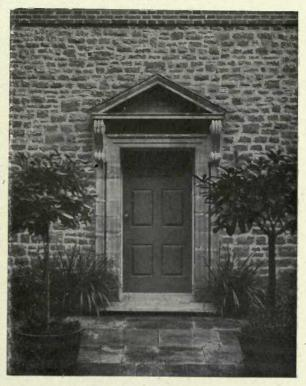
FIG. 243.—PAVEMENT OF RECTANGULAR FLAGS OF PORTLAND STONE.
