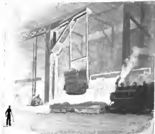
LADLE CONTAINING FIFTY TONS OF MOLTEN STEEL BEING PLACED ON A CONVEYING-CAR.
