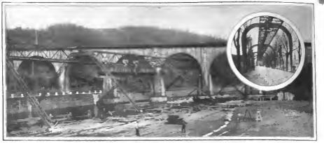
THE NEW ELECTRIC SUSPENSION RAILWAY AT BARMEN, GERMANY. The car can be suspended on two heavy bogies 97 feet in length. The frame surrounds the car across a span that the wheels cannot rise from the rails, and the car is raised up over a strong bridge of 15 feet or more in height. The current is fed by a contact shoe below the rail. The inventor lives in Vienna, Austria.
