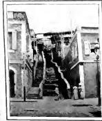
A TYPICAL HILL-SIDE STREET, WITH WATER-COURSE DOWN THE MIDDLE.
