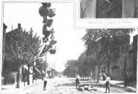
ACTUAL CONDITION OF MOST OF THE TROLLEY WIRES IN THE CITY.
