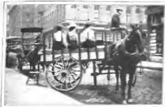
THROUGHOUT STREET CONDUITS
