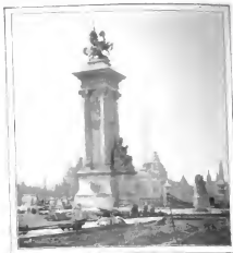
THE ENTRANCE TO THE NEW ALEXANDER III BRIDGE.
