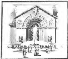
ENTRANCE TO THE HORTICULTURE BUILDING.
