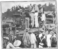
LOADING WAGONS FOR THE FRONT.
