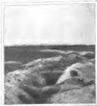
A PORTION OF GENERAL CRONJES' ENTRENCHMENTS.
