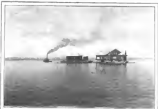
MOVING A HOUSE BY WATER
