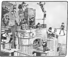
Skilled Labor at Work on a Boston Municipal Building.
