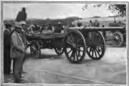
A NAVY 48-POUNDER, MOUNTED FOR SERVICE AS A FIELD-GUN
