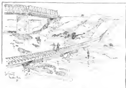
THE BRIDGES OVER MODDER RIVER. In the Background is the Railroad Bridge that was blown up by the Boers. The Trestle Bridge in the Foreground was constructed by the Royal Engineers.
