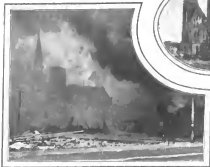
THE BEGINNING OF THE FIRE.
