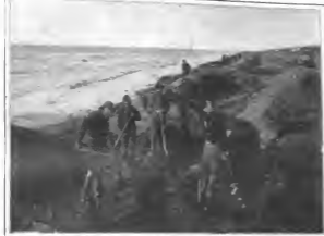
DRAINING ON THE BEACH AT CAPE NOME
