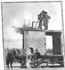
FREIGHT-CAR USED AS A MOVABLE OBSERVATION TOWER
