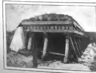
CASEMATE IN THE REDOUBT "EL MAZO."
