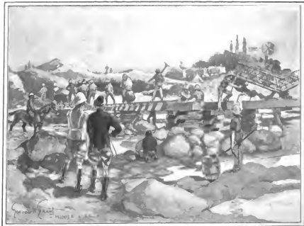
THE ROYAL ENGINEERS BUILDING A RAILWAY BRIDGE ACROSS THE MODDER RIVER DRAWN ON THE FIELD BY GORDON H. GRANT, SPECIAL ARTIST FOR "HARPER'S WEEKLY" The Iron Structure Moves up by the Bars & to be seen in the Background. The crossed Train is on the Embankment.
