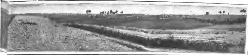
SECTION OF THE LAND DEFENCES OF HAVANA on the Pampas are for Machine guns. This is a striking example of a defunct Exterior Ditch.
