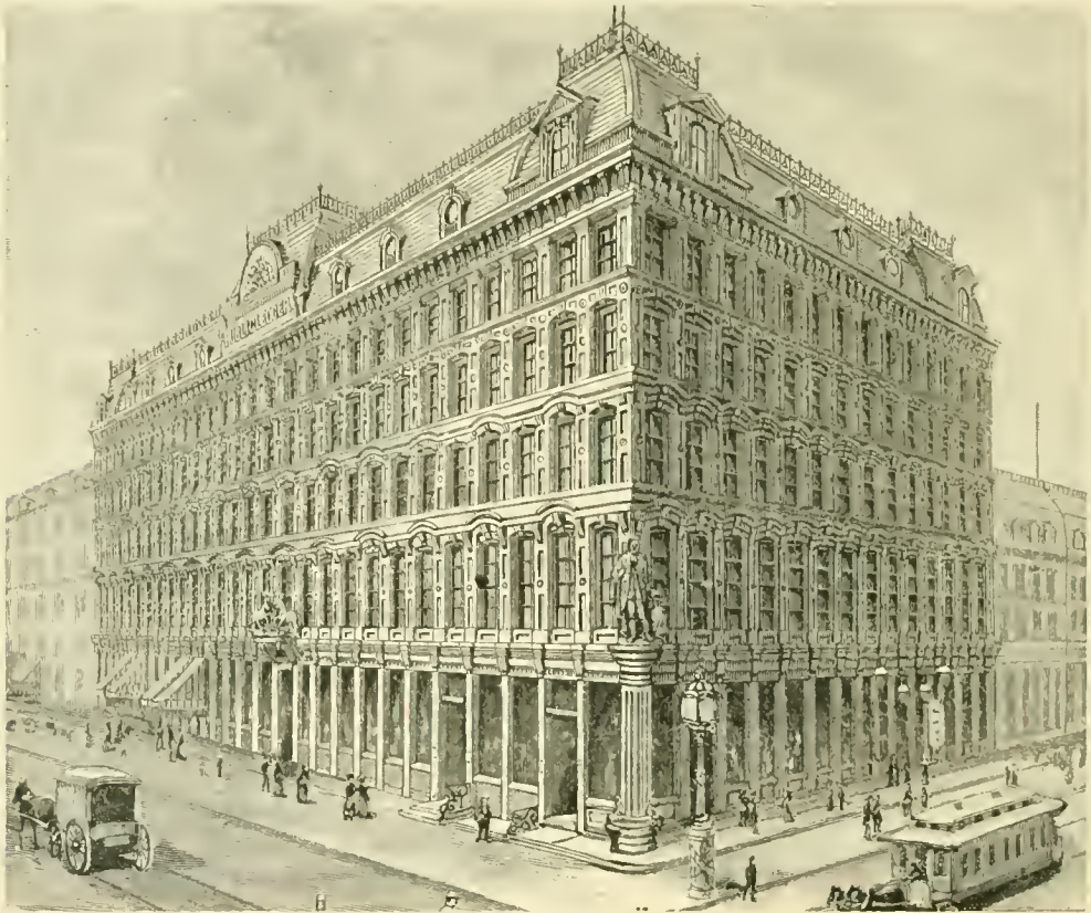
PUBLIC LEDGER BUILDING.
