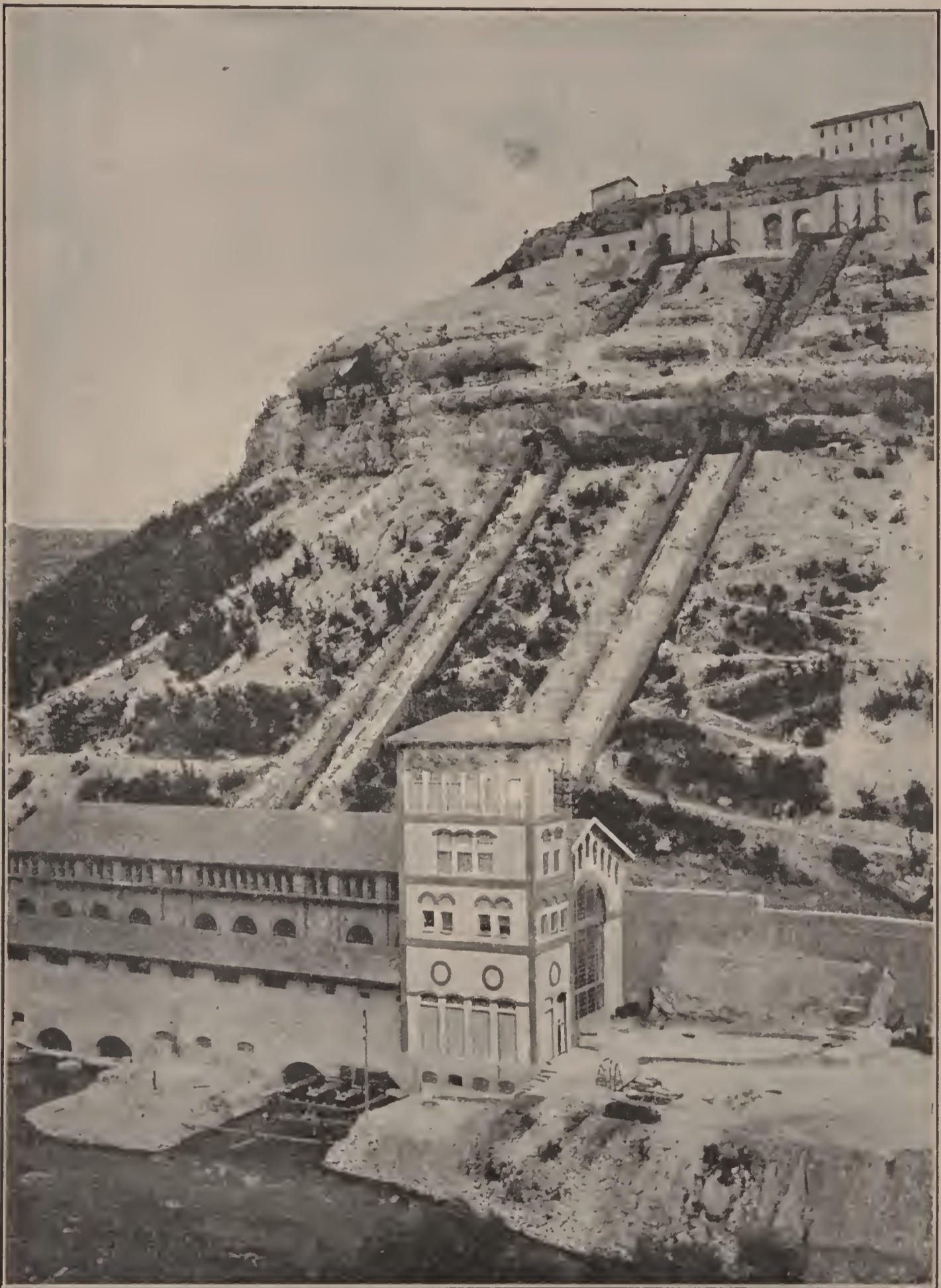
FIG. 15.—The electric power installation in Manojlovac (Ganz), Dalmatia; water head, 330 feet, 24,000 horsepower.
