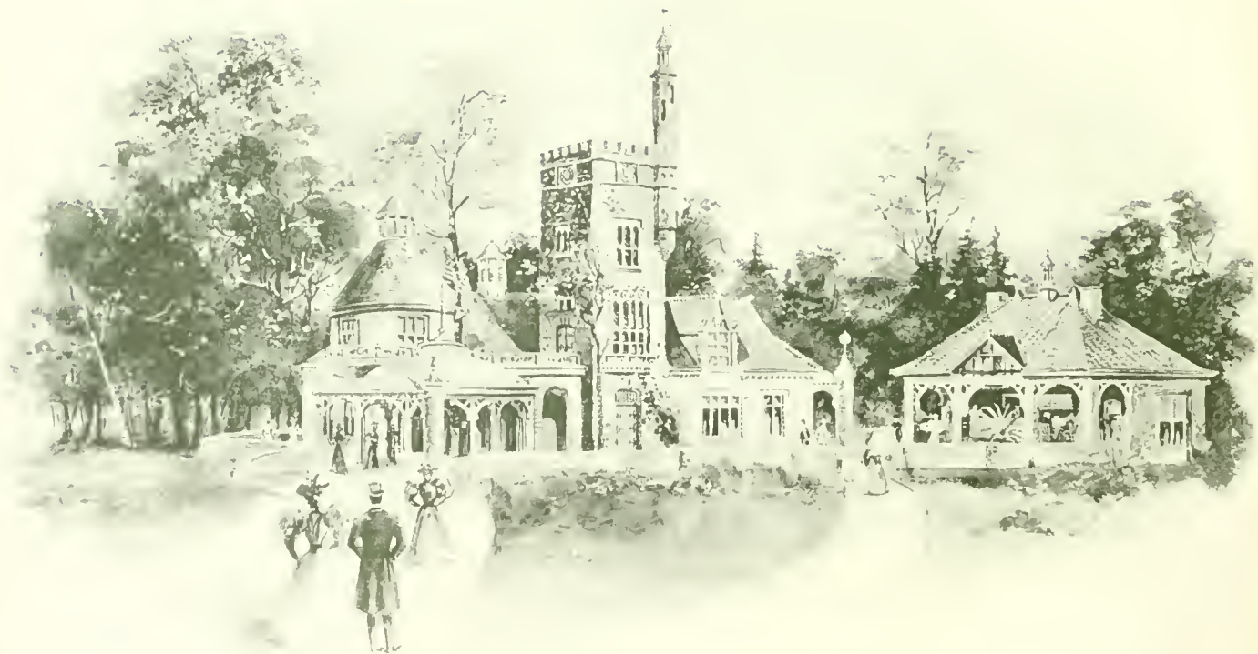
THE SPRING HOUSE OF THE FUTURE (IN COURSE OF CONSTRUCTION).
