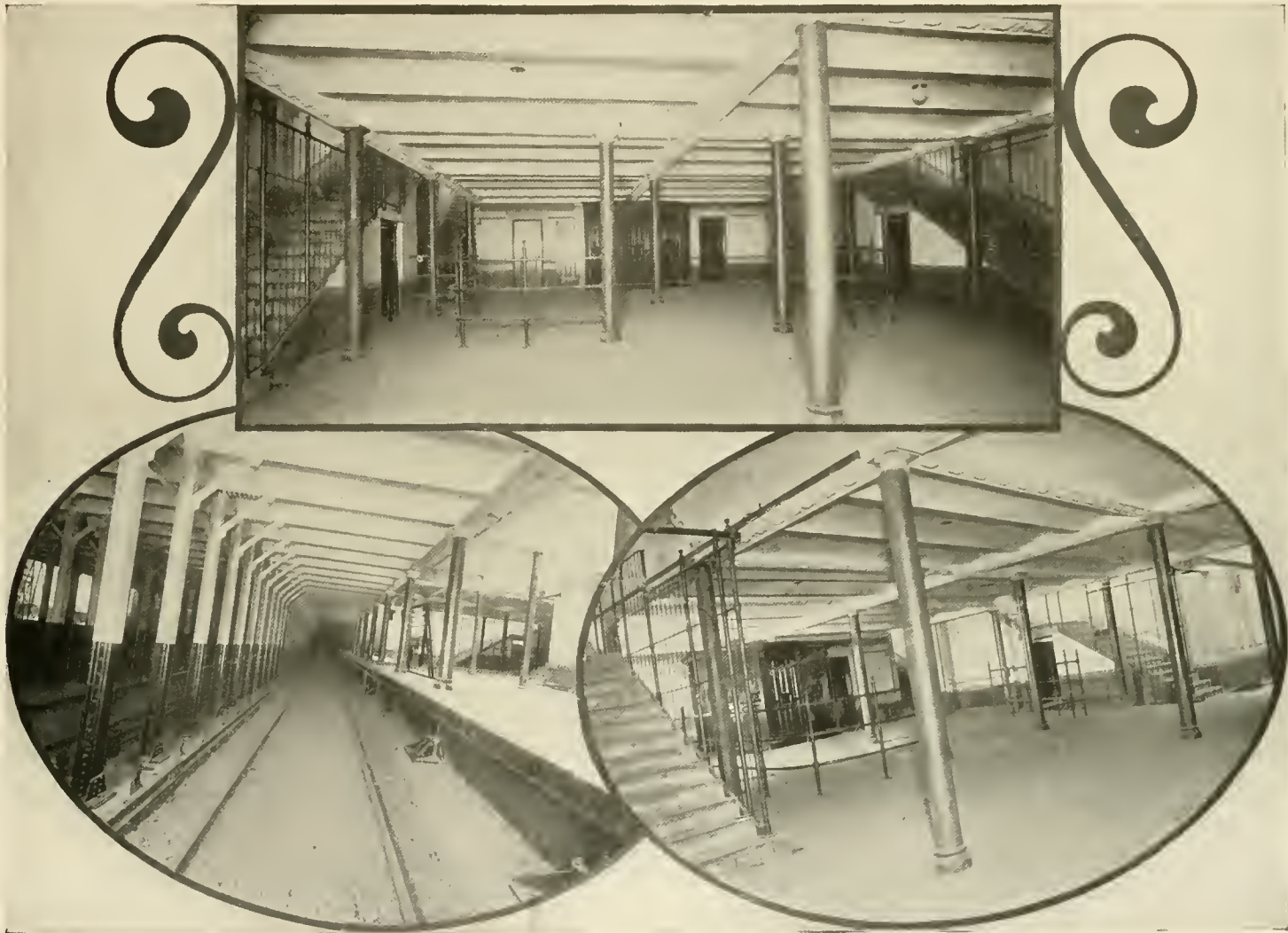
INTERIOR OF SUBWAY. The Subway is rectangular, 13 feet high and 25 feet wide for 2-track sections, 50 feet wide for 4-track sections. The bed is of concrete, with steel frame construction, concrete walls and roof, lined with asphalt and roofing-felt. It is mostly near the surface, but at certain points drops lower, notably at Columbus Avenue and 104th Street, where the cars pass at a depth of 80 feet. At 169th and 181st streets are elevators to stations 110 feet below the surface. The motive power is electricity, using the third rail system. City Hall Park to 96th Street in 13 minutes.
