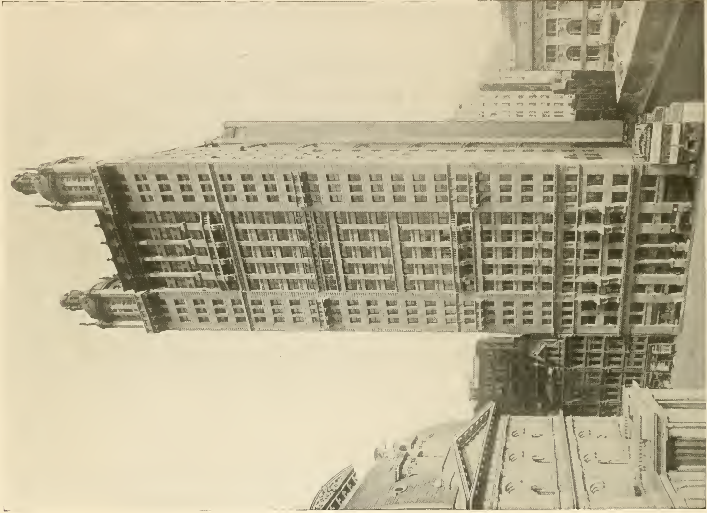
PARK ROW BUILDING, Park Row, opposite Post Office. This is the highest of New York's many skyscrapers, and surpasses anything of its kind in the world for height. It measures 390 feet from the sidewalk to top of towers, which afford a panoramic view of the great city. The 32 floors house more than 6,000 persons. Four letter carriers are required to distribute their mail.
