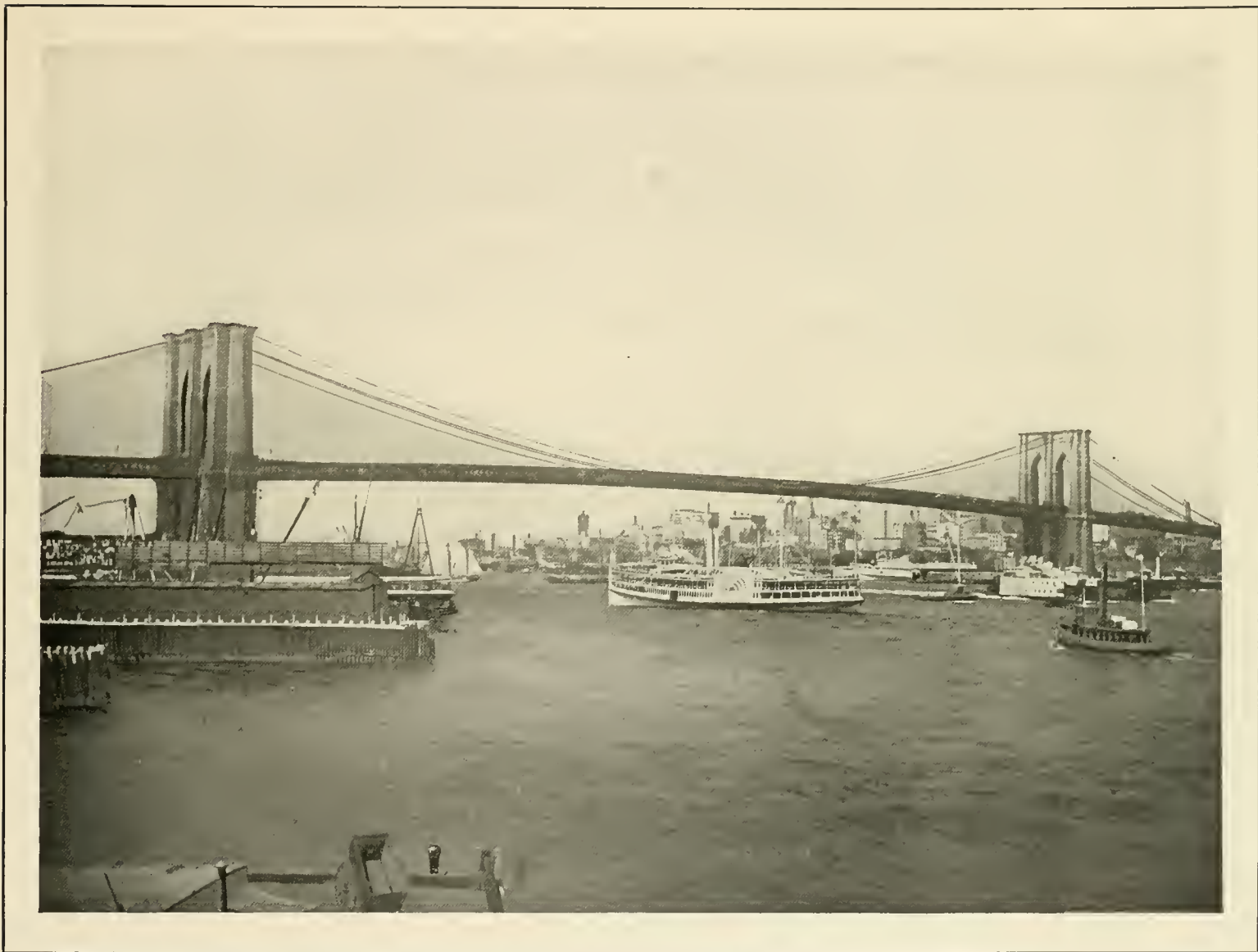
THE BROOKLYN BRIDGE. Stretches from opposite City Hall Park to Fulton and Sand streets, Brooklyn. This magnificent bridge was begun in 1870 and opened to the public in 1883. Cost $21,000,000. It consists of a central river span 1,595 feet long and two land spans, with a total length between terminals of 7,580 feet. The bridgeway carries two cable and two trolley car tracks, two wagon ways and a footpath. 4,000 cars and 2,000 vehicles pass east and west every day. The average number of passengers in twenty-four hours is 300,000. It is estimated that about 5,000,000,000 people have used this bridge since its opening.
