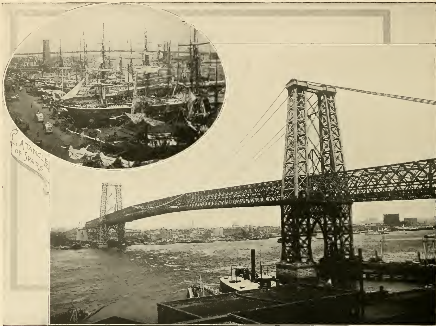
THE WILLIAMSBURG BRIDGE, the greatest suspension bridge in the world, crosses the East River at the Grand Street Ferry to Broadway (Williamsburg) Brooklyn. It is a steel-towered suspension-cantilever structure with a length of 7,200 feet between terminals. The towers are 335 feet high. The central span is 1,600 feet long and 135 feet above the middle of the river. The bridgeway is 118 feet wide, and carries four trolley and two cable tracks, two roadways, two foot-paths, and two bicycle paths. Estimated cost, about $21,000,000.
