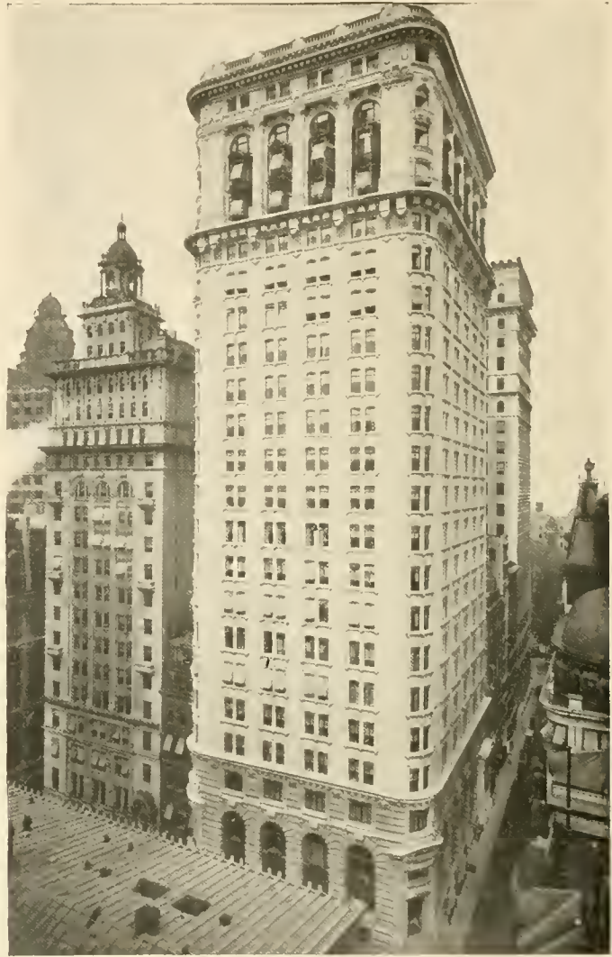
HANOVER BANK BUILDING. Located on the southwest corner of Nassau and Pine streets. This 22-story building, completed in 1901, is justly considered one of the finest office structures in the world. From an artistic standpoint it is a most pleasing example of sky-scraping architecture.
