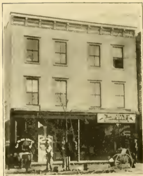
Building and Flats owned by Rev. W. L. Taylor.
