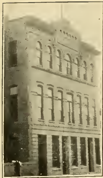
New Hall and former site of the bank of the I. O. O. St. Luke
