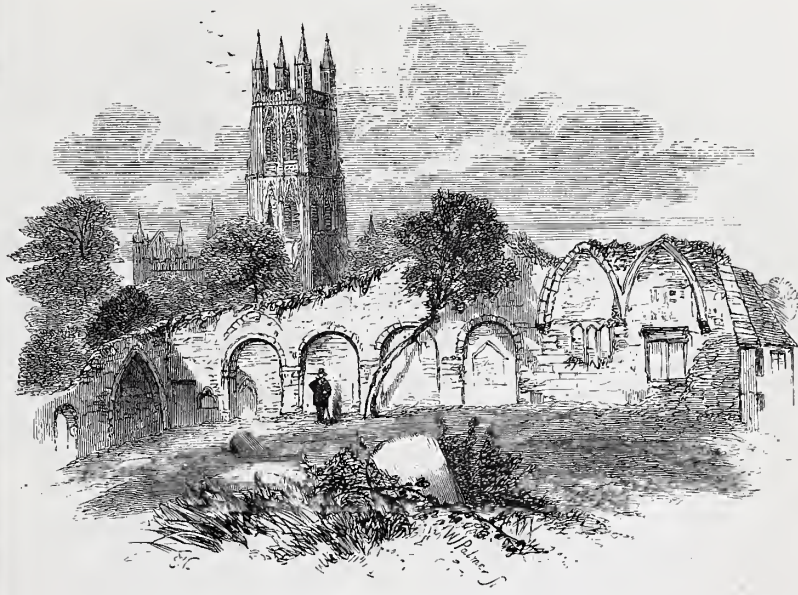
GLOUCESTER CATHEDRAL: ST. OSWALD'S PRIORY.
