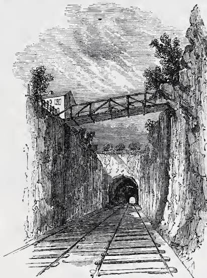
NEW HAMBURG TUNNEL.
