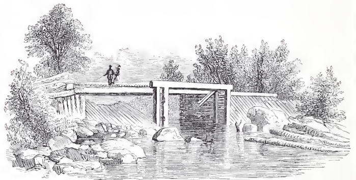
LUMBER DAM AND SLUICE.
