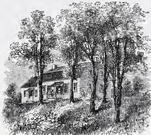
THE REIDSEL HOUSE.
