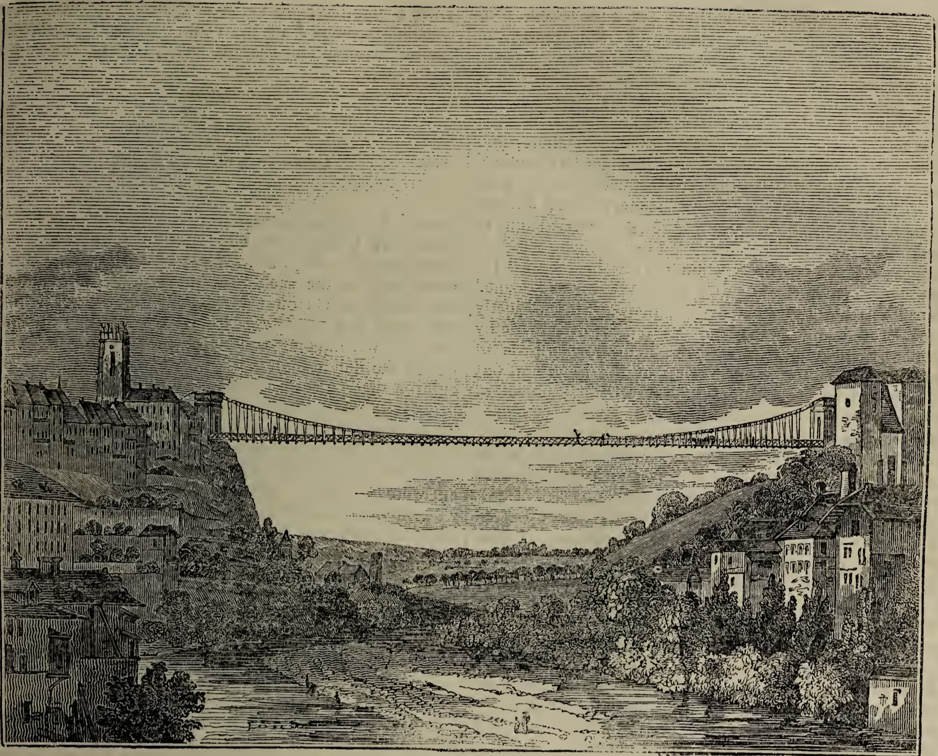
[Fribourg Suspension Bridge.]
