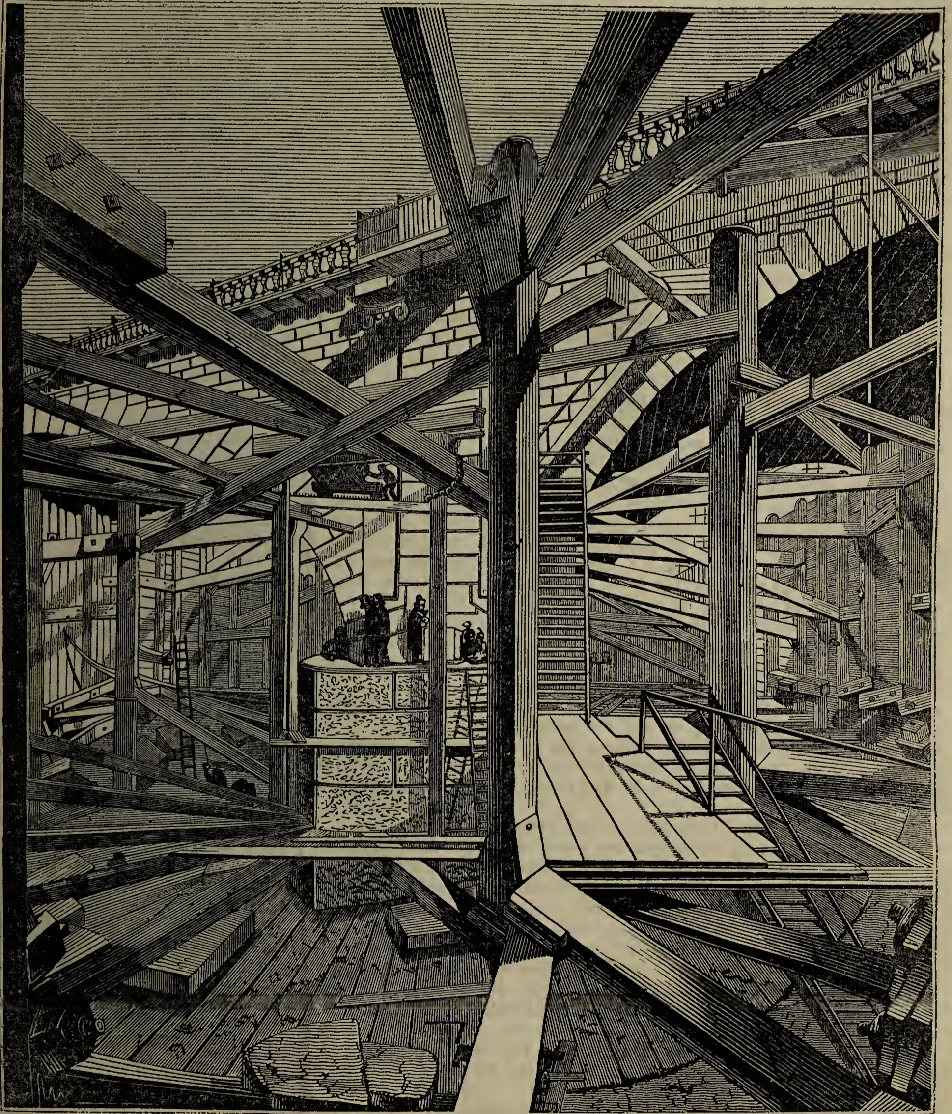
[Coffer-dam for carrying on the repair of Blackfriars' Bridge.]
