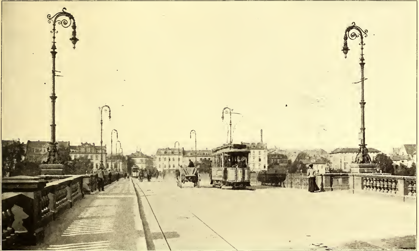
ORNAMENTAL SIDE TROLLEY POLES WITH ARC LIGHTS IN USE IN FRANKFORT
