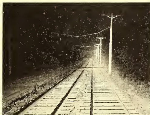
FIG. 2.—SHOWING EFFECTIVE TRACK ILLUMINATION
