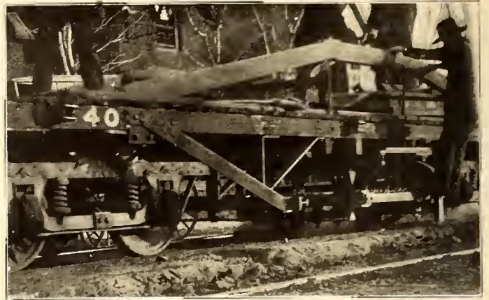
TRACK PLOW, WITH PLOW LOWERED, DENVER CITY TRAMWAY
