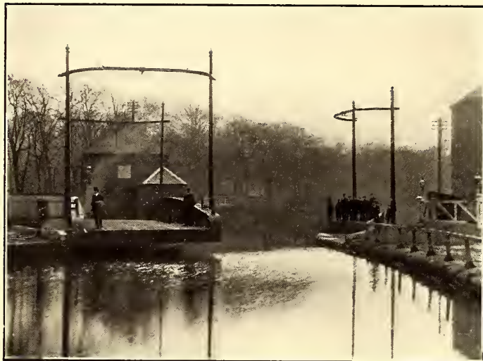
THE CAMELON SWING BRIDGE OPEN
