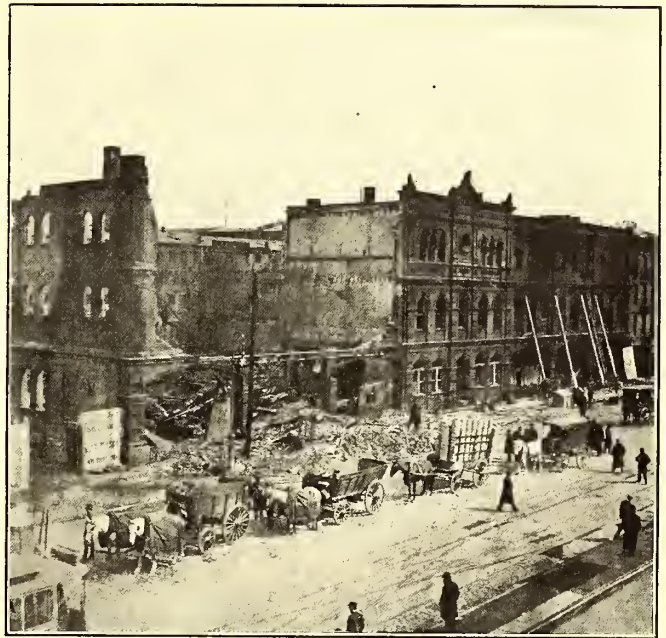
VIEW SHOWING ALL THAT REMAINED OF THE NEW YORK CITY RAILWAY CAR HOUSE AFTER THE FIRE, NAMELY, THE THREE-STORY OFFICE SECTION AND A PORTION OF THE WALLS
