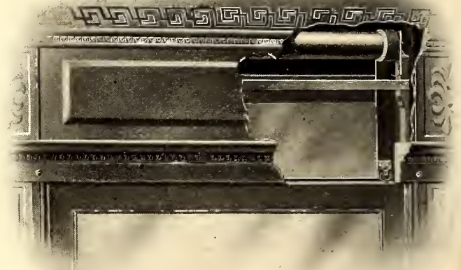
CUT-AWAY VIEW, SHOWING SASH BALANCE
