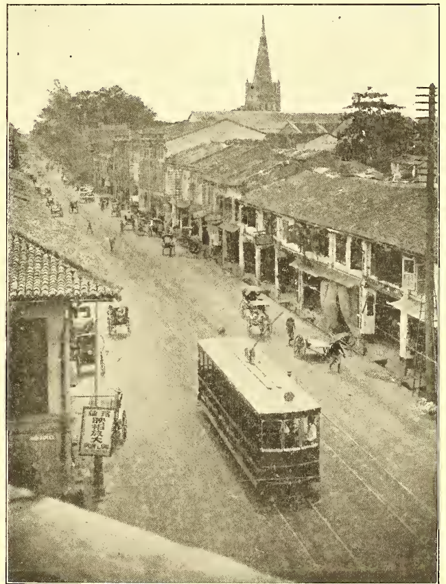
TYPICAL STREET VIEW, SHOWING ATTACHMENT OF SPAN WIRES TO HOUSES
