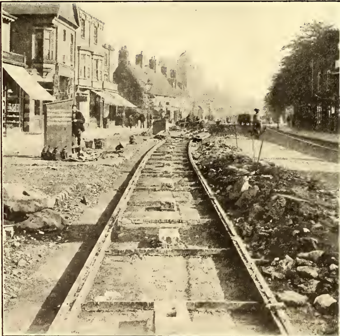
CONDITION OF TRACK WHEN PAVING
