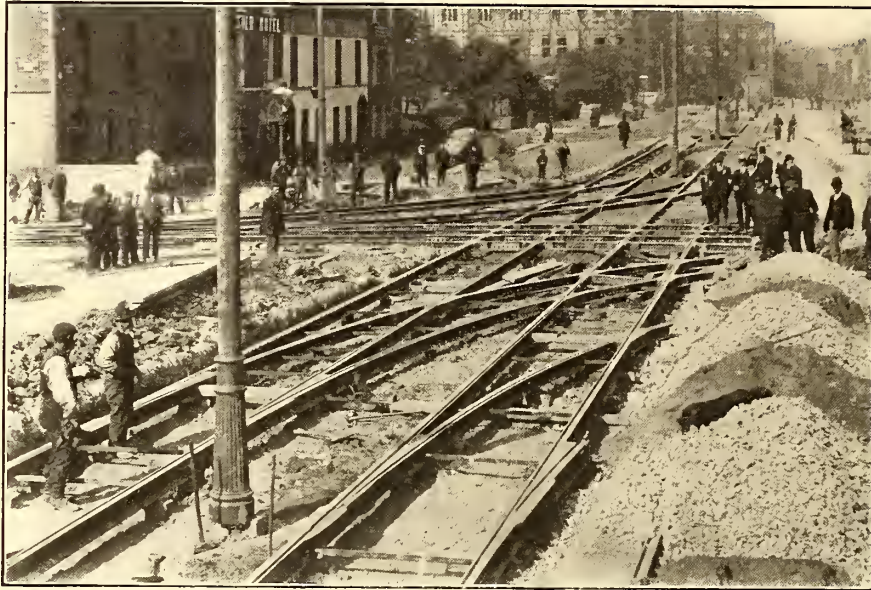
VIEW OF THE TRACK LAYOUT AT FISHERWICK PLACE AND GROSVENOR ROAD
