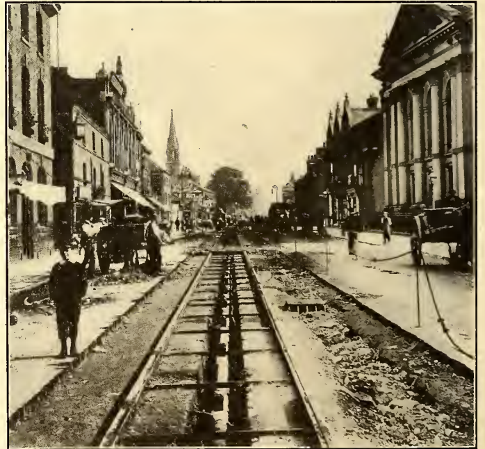
COMPLETED CONDUIT BEFORE FILLING WITH CONCRETE
