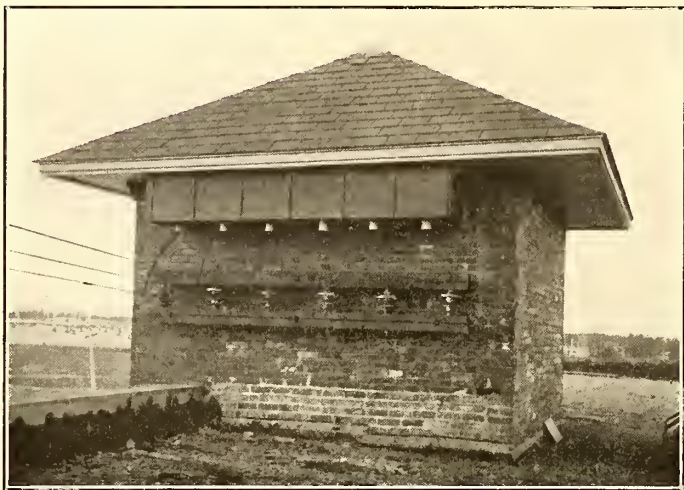
TOWER OF SUB-STATION
