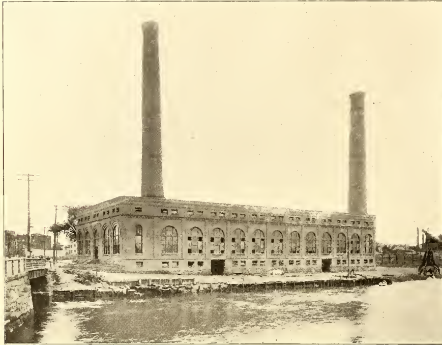
FIG. 1.—THE GRAND AVENUE STATION OF THE CONSOLIDATED RAILWAY AT NEW HAVEN, CONN., TAKEN BEFORE INSTALLATION OF COAL-HANDLING APPARATUS
