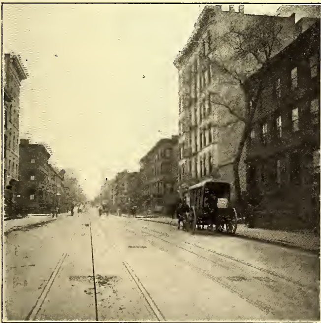
ALONG LEXINGTON AVENUE, NEW YORK, WHICH IS PAVED WITH CREO-RESINATE WOOD BLOCKS
