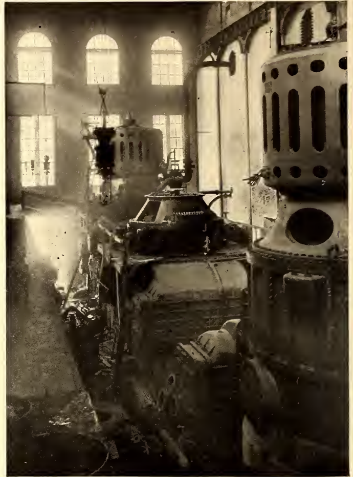
VIEW IN TURBINE ROOM, MARION STATION DURING CONSTRUCTION
