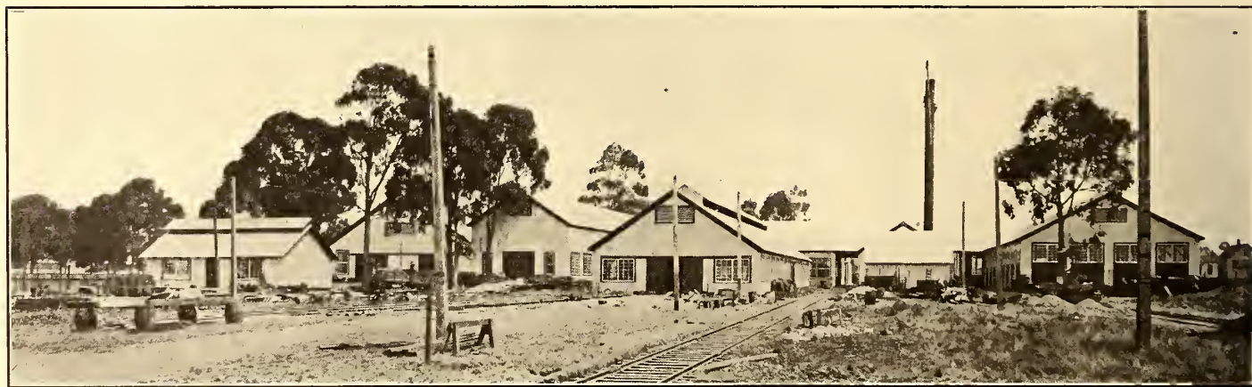
GENERAL VIEW, OAKLAND TRACTION SHOPS
