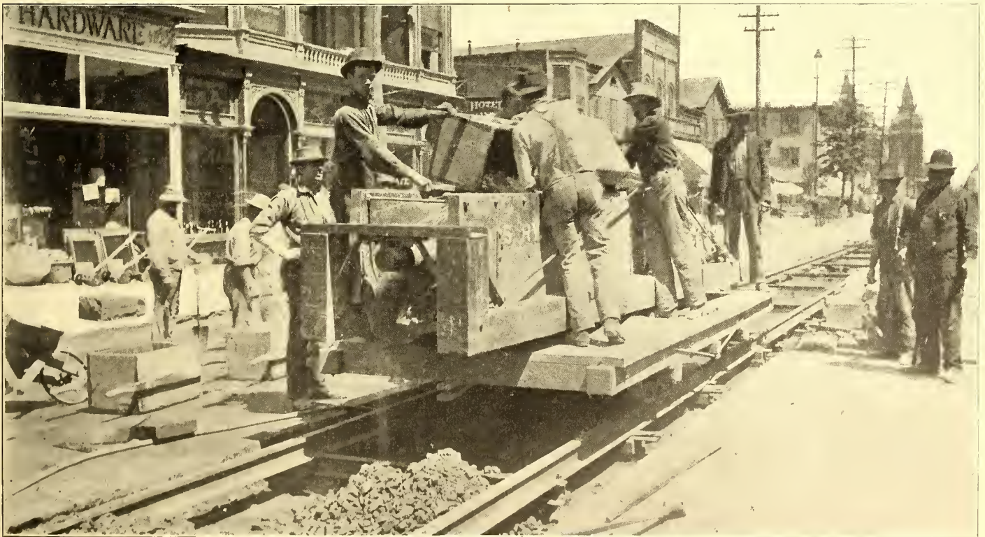
PORTABLE CONCRETE MIXER, SCRANTON RAILWAY
