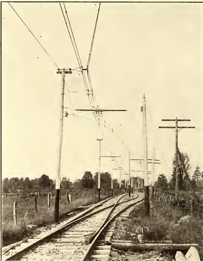
TURN-OUT SHOWING CATENARY OVERHEAD CONSTRUCTION
