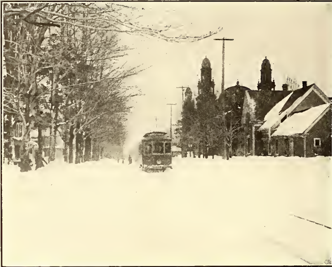
TYPICAL STREET SCENE IN MARQUETTE DURING WINTER
