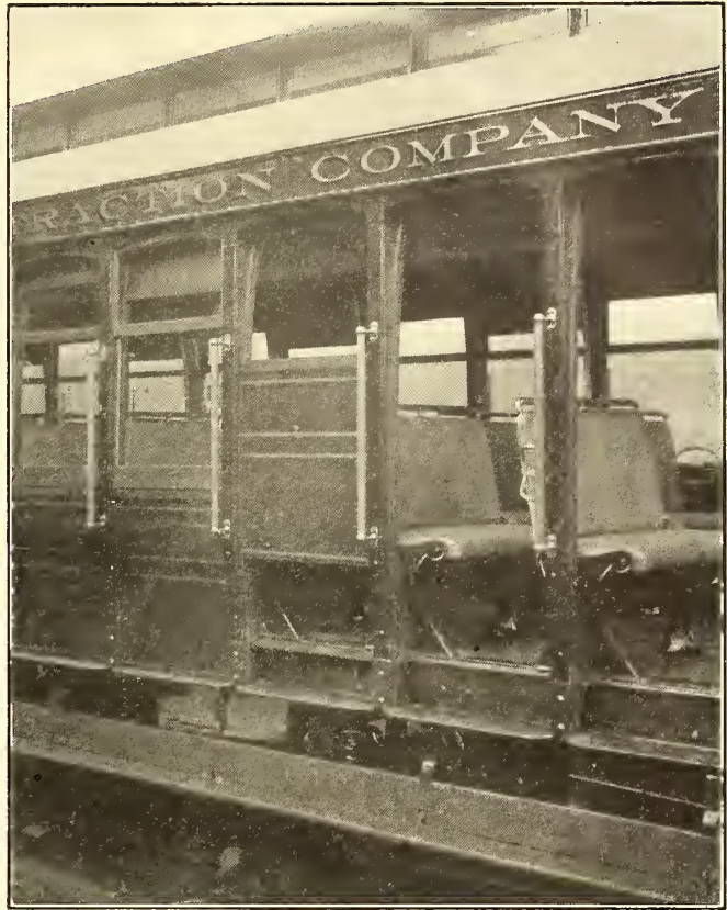
VIEW OF PART OF ONE SIDE OF THE KANAWHA CAR, ILLUSTRATING Z-BAR SILL CONSTRUCTION
