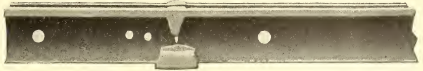
THE JOINT AFTER WELDING
