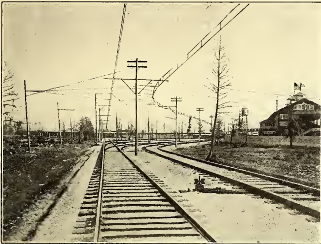
DIRECT-CURRENT CATENARY AT NEW ORLEANS
