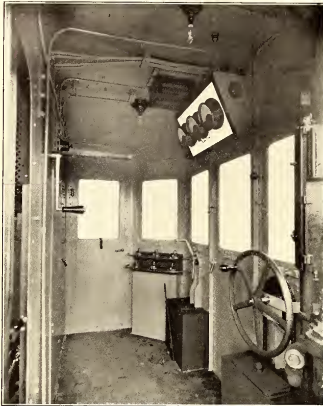
MOTORMAN'S CAB OF 15,000-VOLT, SINGLE-PHASE LOCOMOTIVE
