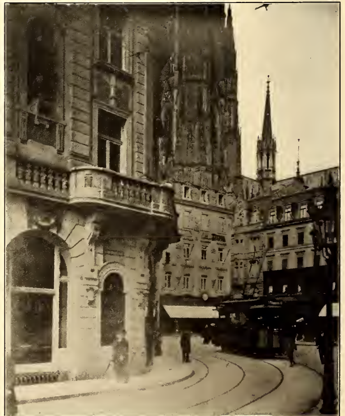
SPAN WIRES ATTACHED TO BUILDINGS IN COLOGNE NEAR THE CATHEDRAL
