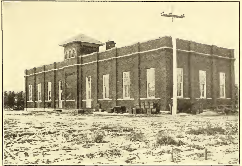
EXTERIOR OF NEW SUB-STATION
