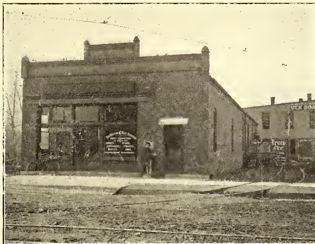
EXTERIOR OF TROY FREIGHT AND PASSENGER STATION
