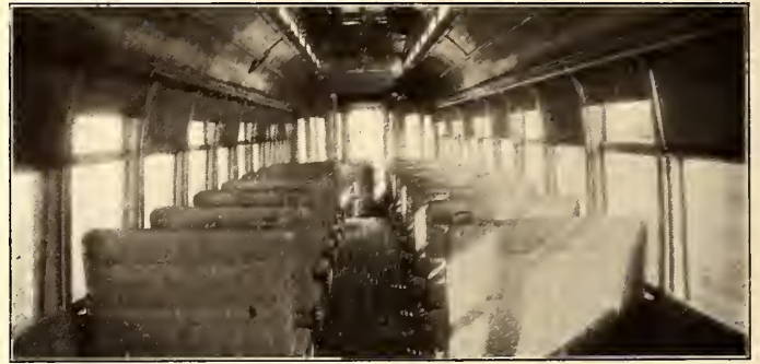
INTERIOR OF CAR, WITH ROOF POCKETS FOR THE PANELS
