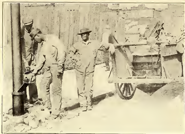
Illustration No. 2 Pouring the Sulphur—Wagon for Melting Sulphur at right.
