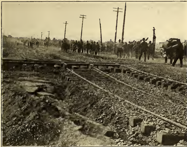
TWO SCENES ALONG THE LINES OF THE OAKLAND CONSOLIDATED TRACTION COMPANY, SHOWING THE UPHEAVAL OF THE ROADBED AND TWISTING AND BREAKING OF THE RAILS
