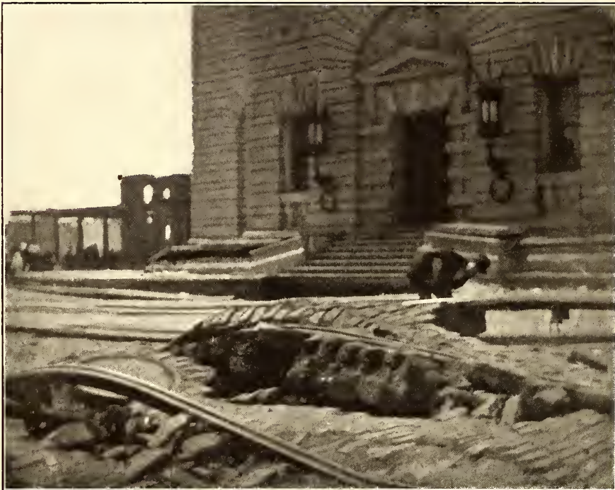
WHAT THE EARTHQUAKE DID TO THE TRACK AND ROADBED OF THE CABLE SYSTEM IN FRONT OF THE SAN FRANCISCO POST OFFICE
