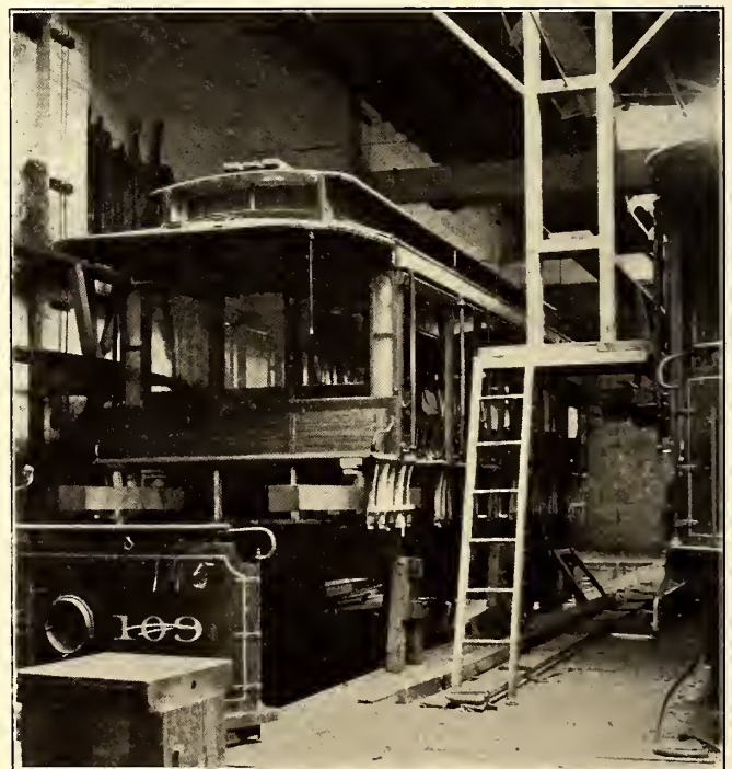
FIG. 5.—ELEVATED PLATFORMS IN CARPENTER SHOP, ST. JOSEPH, MO.
