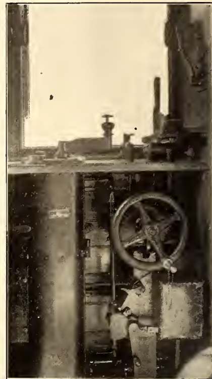
SINGLE-PHASE MASTER CONTROLLER IN CAB OF HAMBURG CAR
