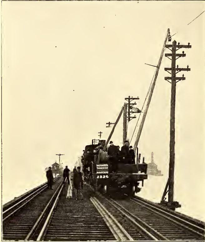
FIG. 18.—STRINGING CABLE ON JAMAICA BAY TRESTLE
