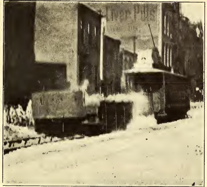
VIEW ON OLIVE STREET, TAKEN DURING EXPLOSION
