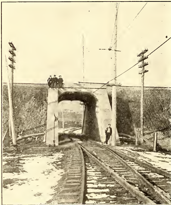
VIADUCT UNDER VANDALIA RAILWAY, ST. MARY'S LINE
