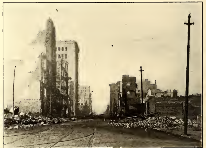
LOOKING DOWN MISSION STREET, SAN FRANCISCO
