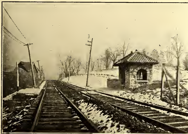
PRIVATE WAITING STATIONS ON THE FLORISSANT-FERGUSON DIVISION OF THE ST. LOUIS & SUBURBAN RAILWAY
