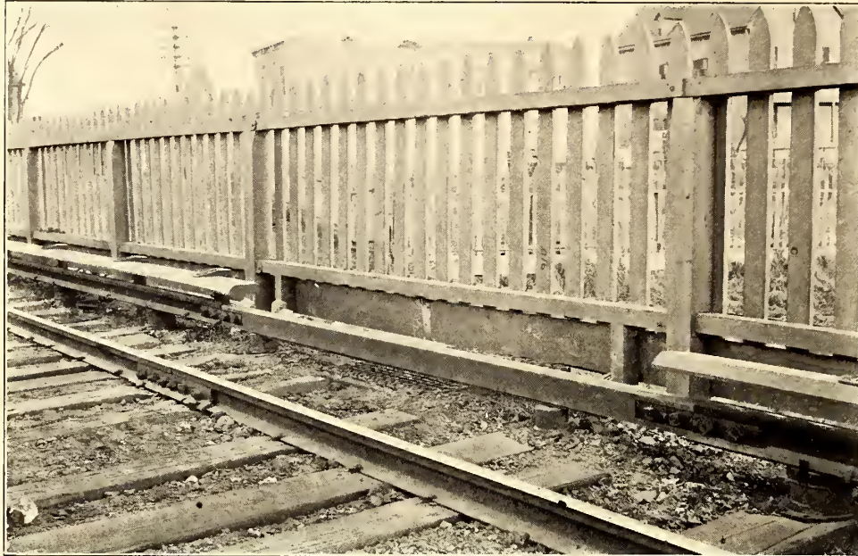
FIG. 25.—10-FT. BREAK IN THIRD RAIL OVER MANHOLE COVERS ON ATLANTIC AVENUE
