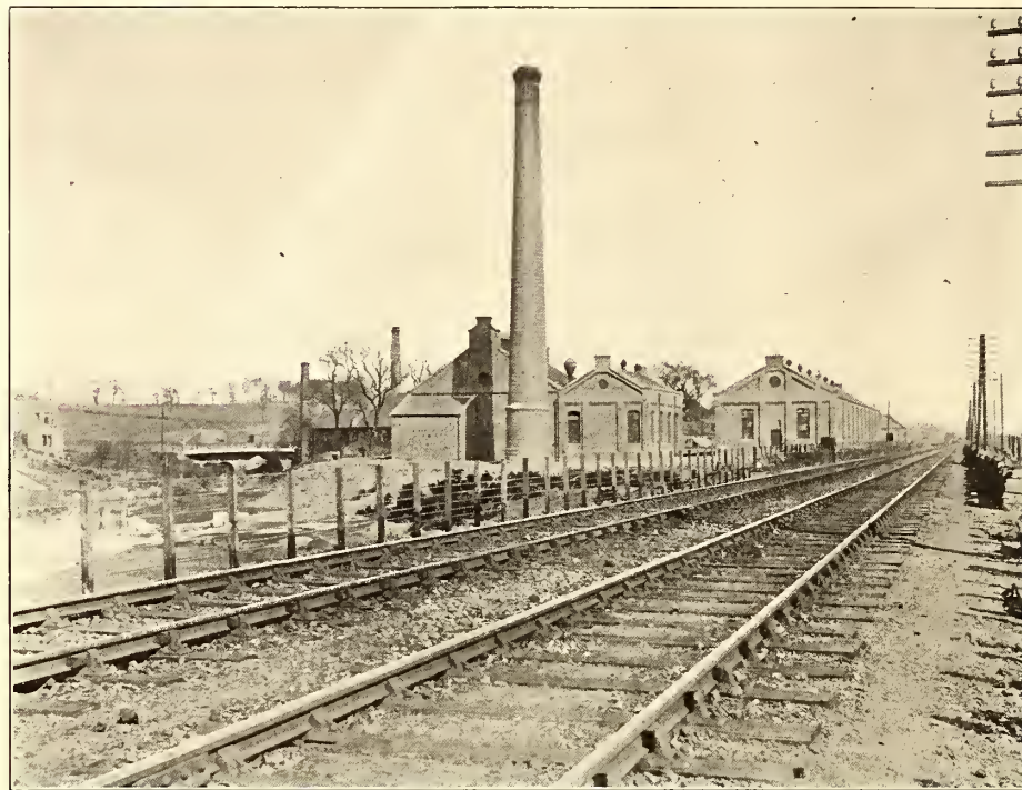
EXTERIOR OF POWER STATION AND CAR HOUSE, DUNDEE & MONIFIETH INTERURBAN RAILWAY
