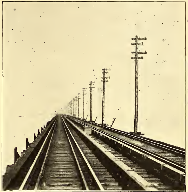
FIG. 13.—WOODEN-POLE CONSTRUCTION ON JAMAICA BAY TRESTLE
