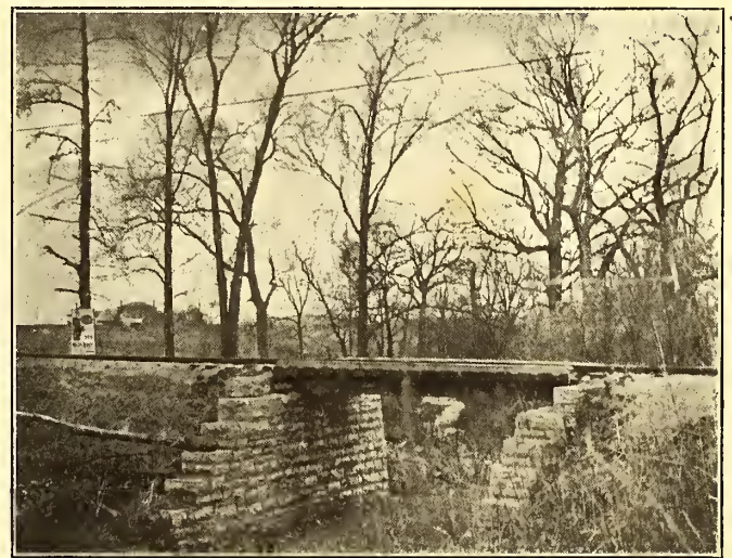
A 15-FT. SPAN WITH STONE BUTTRESSES
