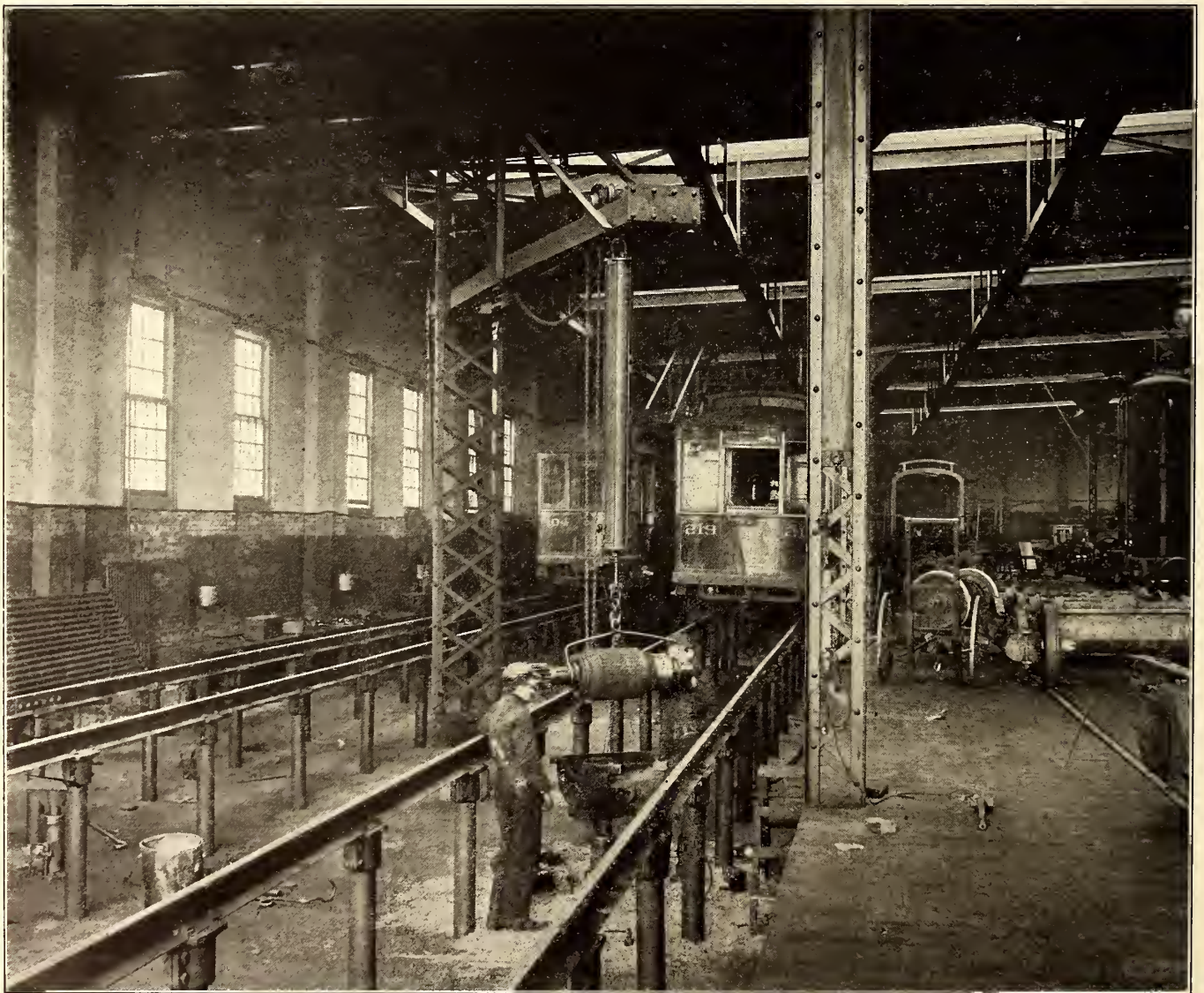
A PORTION OF THE REPAIR SHOPS AT BIRMINGHAM, SHOWING METHOD OF SUPPORTING RAILS OVER PITS, AND CONVENIENT ARRANGEMENT OF JIB CRANE AND JACKS FOR EXPEDITING TRUCK AND MOTOR REPAIR WORK
