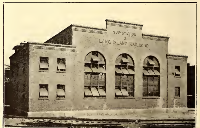
FIG. 6.—THE EAST NEW YORK SUB-STATION
