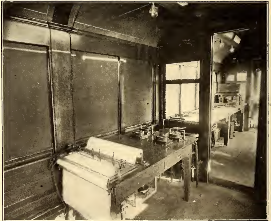
INTERIOR, SHOWING TABLE ON WHICH ARE RECORDED SPEED ACCELERATION AND CURVE
