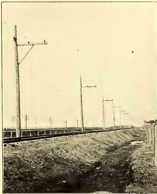
FIG. 1.—OVERHEAD CONSTRUCTION ON STRAIGHT TRACK
