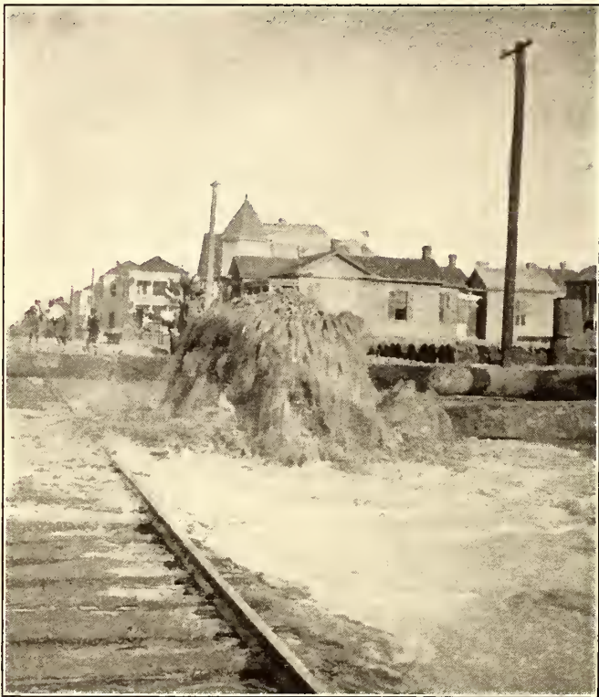
VIEW SHOWING END OF 42-IN. PIPE DISCHARGING SAND AND WATER IN THE GRADE-RAISING OPERATIONS AT GALVESTON
