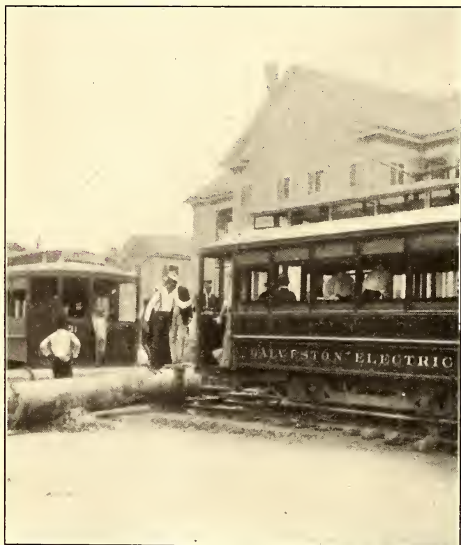
OPERATING UNDER DIFFICULTIES. THE VIEWS SHOW 42-IN. PIPES ACROSS THE TRACKS OF THE GALVESTON ELECTRIC COMPANY DURING THE GRADE-RAISING OPERATIONS
