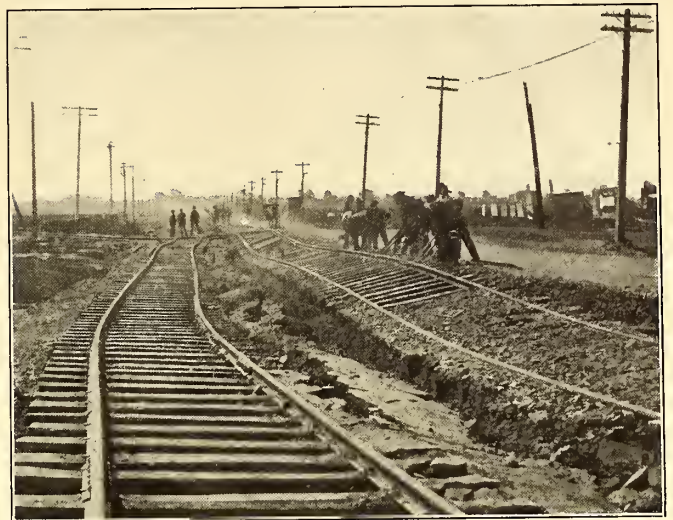
TWO SCENES ALONG THE LINES OF THE OAKLAND CONSOLIDATED TRACTION COMPANY, SHOWING THE UPHEAVAL OF THE ROADBED AND TWISTING AND BREAKING OF THE RAILS
