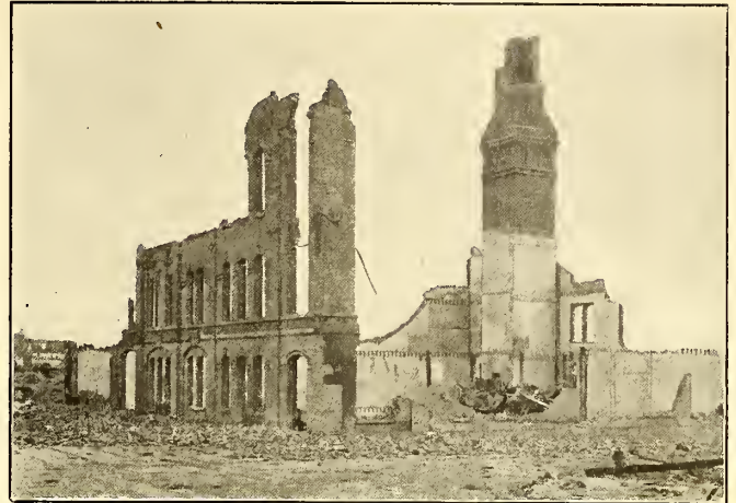
RUINS OF THE SUTTER STREET CABLE POWER HOUSE, UNITED RAILROADS, OF SAN FRANCISCO
