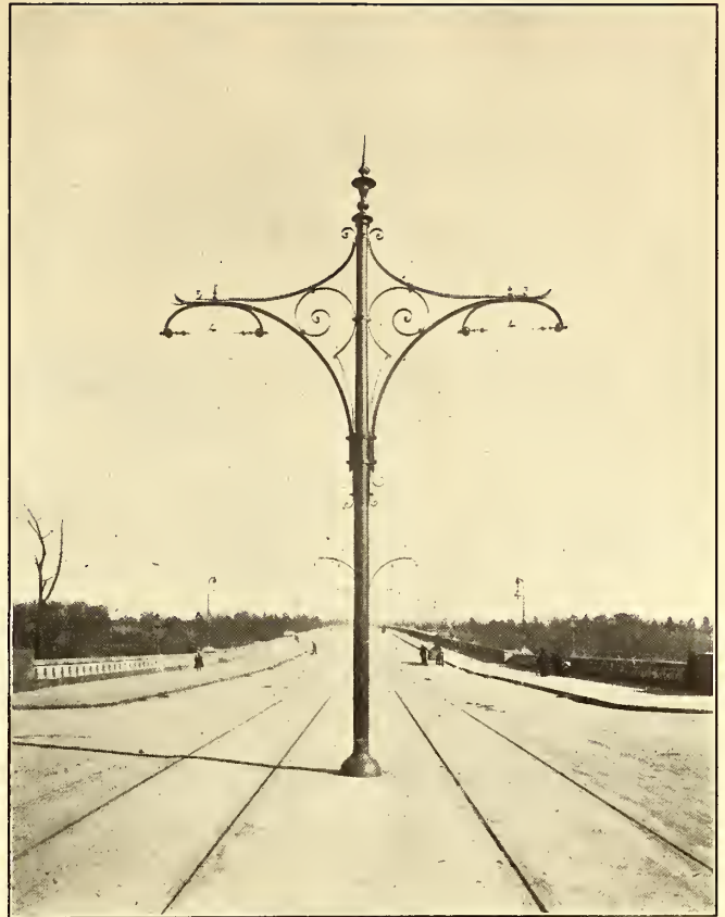
ARTISTIC OVERHEAD CONSTRUCTION ON WASHINGTON BRIDGE
