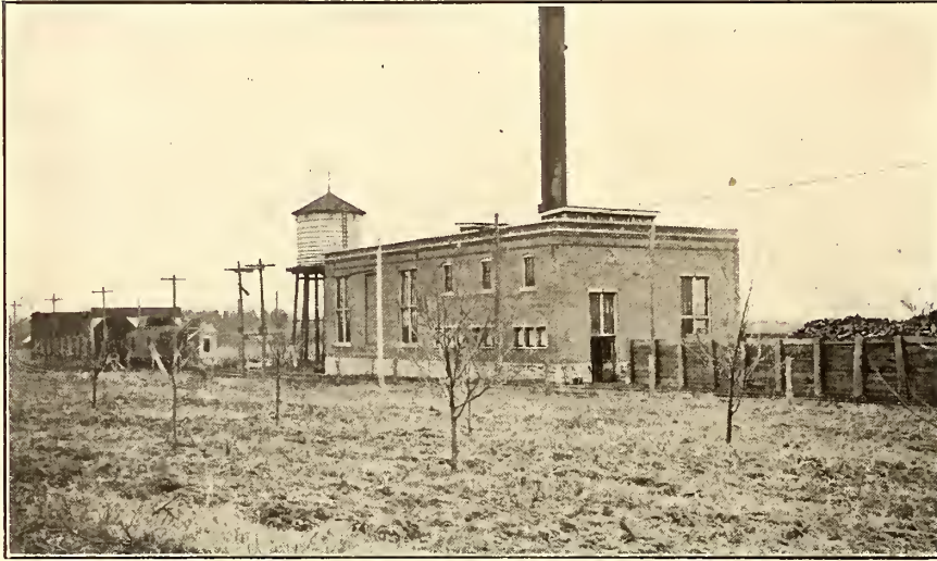
POWER HOUSE, WITH REPAIR SHOPS ON THE LEFT
