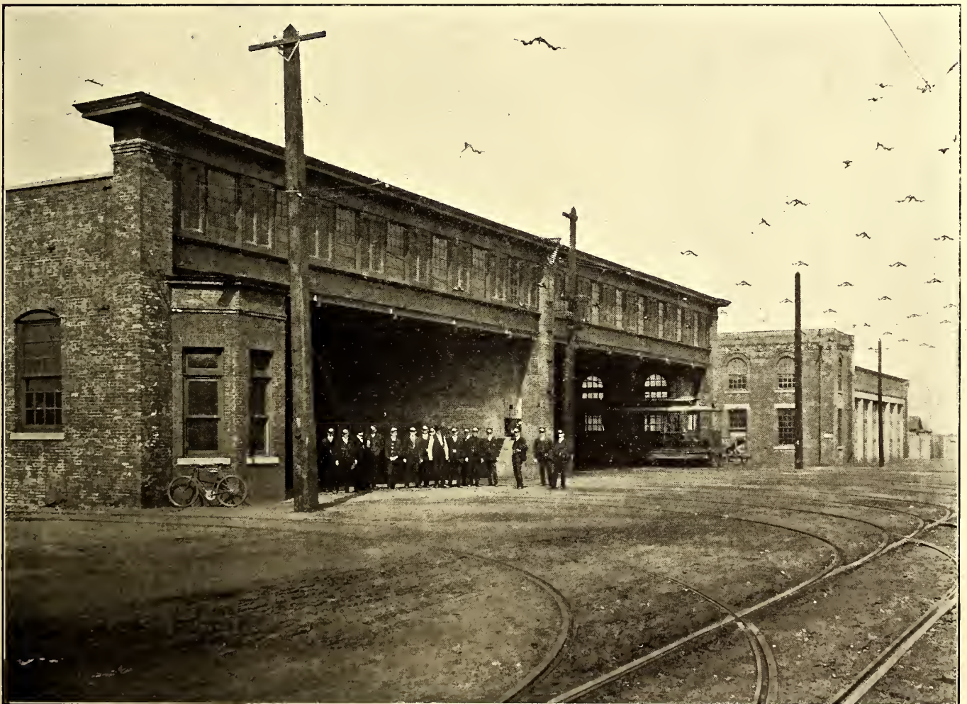
CAR HOUSE AND REPAIR SHOP AT BIRMINGHAM. THE BUILDING IN THE FOREGROUND IS THE CAR HOUSE, AND THE REPAIR SHOPS ARE SHOWN IN THE BACKGROUND
