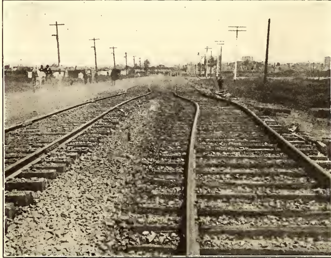
TRACK TWISTED IN OAKLAND BY THE EARTHQUAKE
