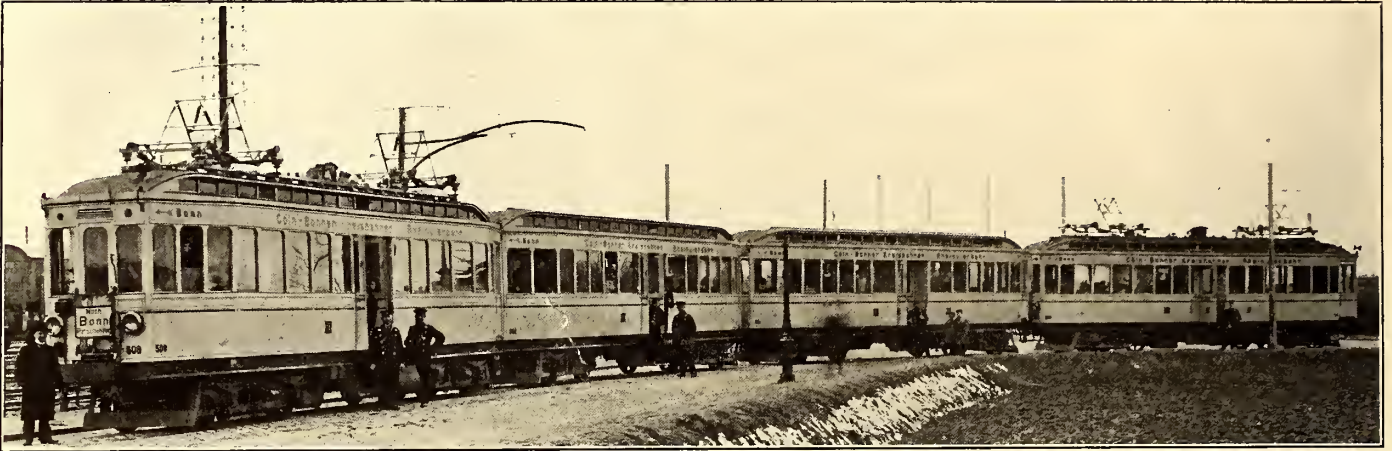
A TRAIN OF TWO MOTOR CARS AND TWO TRAILERS ON THE 990-VOLT DIRECT-CURRENT LINE BETWEEN COLOGNE AND BONN
