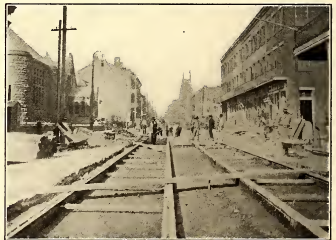
CONCRETED TRACK READY FOR PAVING, NEW ORLEANS
