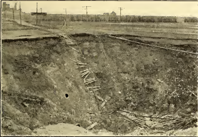
CAVE IN ON THE DUNENWEG LINE OF THE SOUTHWEST MISSOURI ELECTRIC RAILWAY COMPANY
