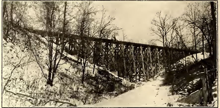
TRESTLE BRIDGE ON ST. MARY'S LINE
