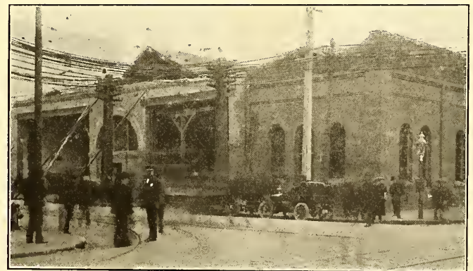
CAR HOUSE AT TURK AND FILLMORE STREETS, SLIGHTLY DAMAGED BY FIRE AND EARTHQUAKE, BUT NOW USED AS MAIN OFFICES BY THE UNITED RAILROADS, OF SAN FRANCISCO
