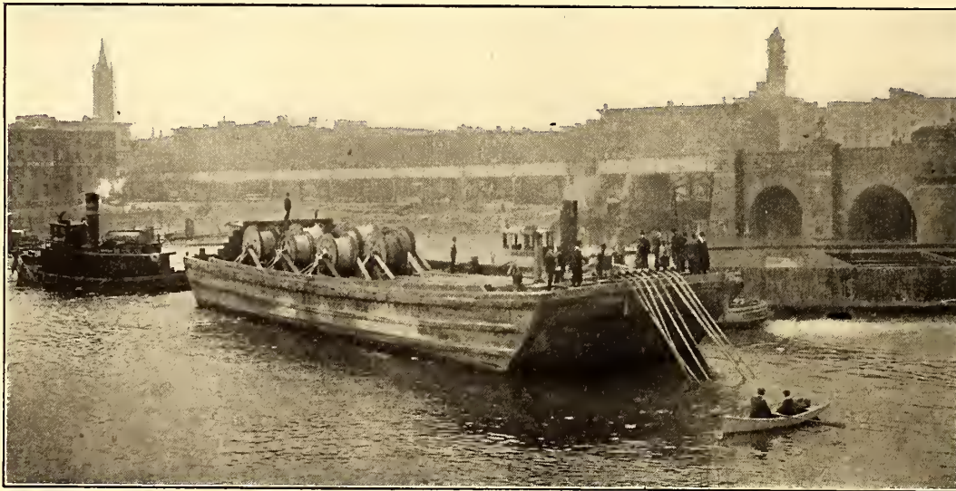
METHOD OF LAYING CABLE ACROSS THE HARLEM RIVER
