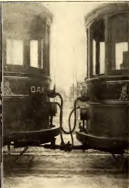
FIG. 5.—COUPLING BETWEEN TWO CARS
