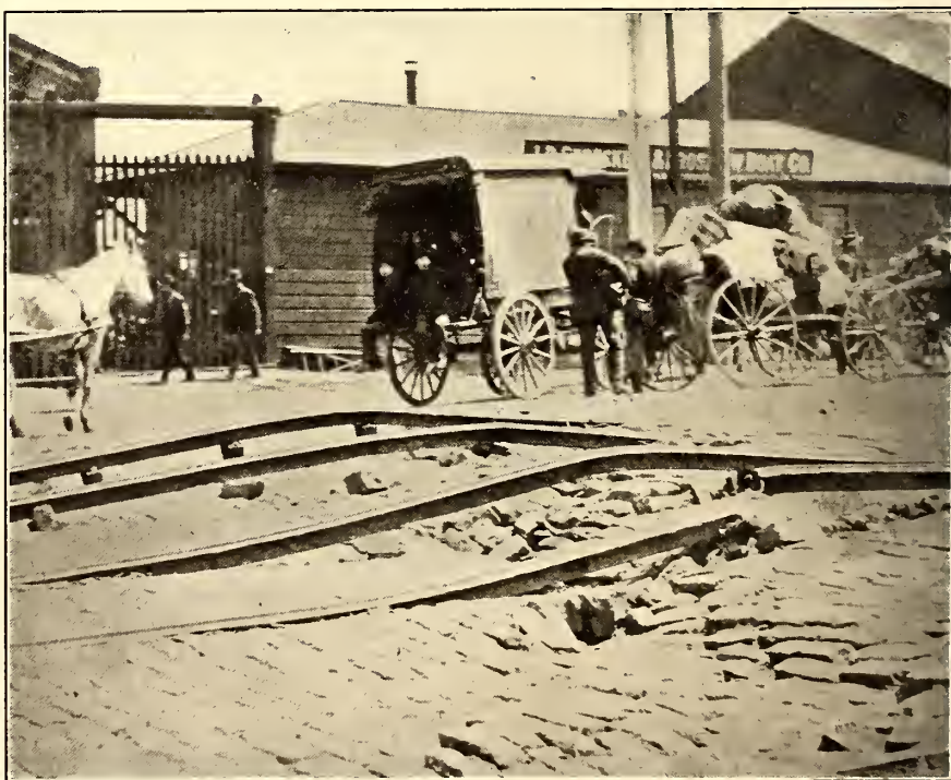
ANOTHER VIEW, SHOWING TRACKS TWISTED AND BROKEN BY THE EARTHQUAKE, AND WAGONS LOADED WITH REFUGEES, FURNITURE AND MERCHANDISE
