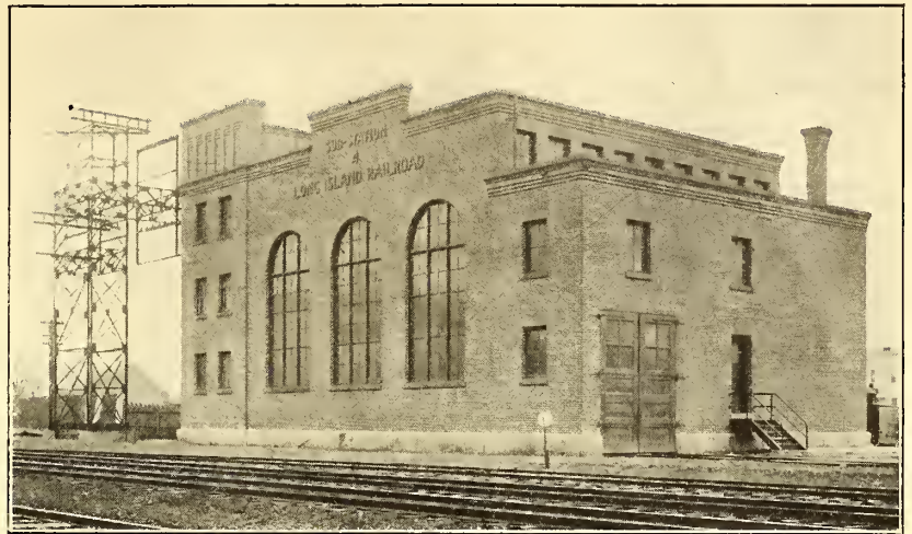
FIG. 9.—SUB-STATION AT ROCKAWAY JUNCTION
