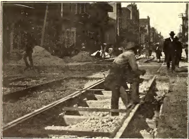
PUTTING IN CONCRETE IN TRACK WORK, NEW ORLEANS
