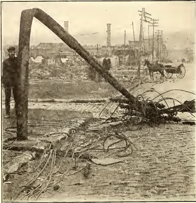
IRON TROLLEY POLE ON BRYANT STREET, BENT AS A RESULT OF THE INTENSE HEAT. THE VIEW, INCLUDING THE CHINAMAN REFUGEE ON THE LEFT AND THE DEAD DOG ON THE RIGHT, IS TYPICAL OF SCENES COMMON AFTER THE FIRE
