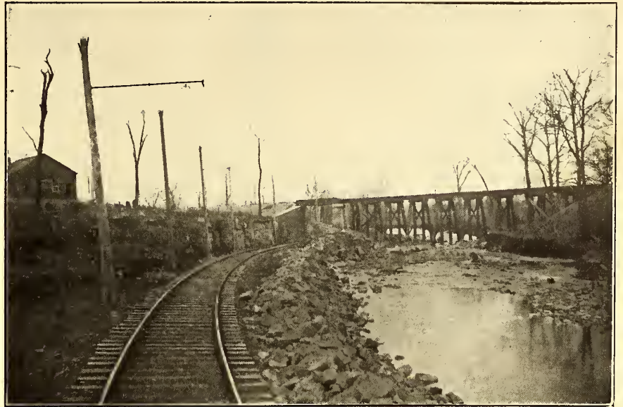
CROSSING UNDER THE ILLINOIS SOUTHERN RAILWAY
