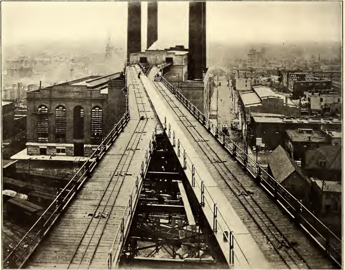
FIG. 3.—COAL BRIDGE, VIEWED FROM TOWER
