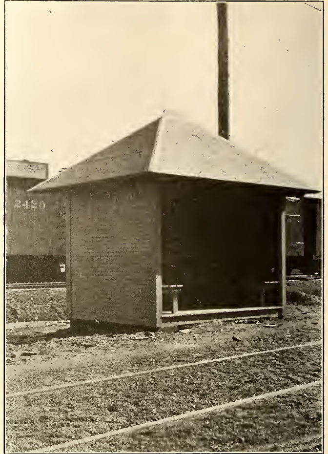
TYPE OF WAITING STATION ON SULLIVAN LINE
