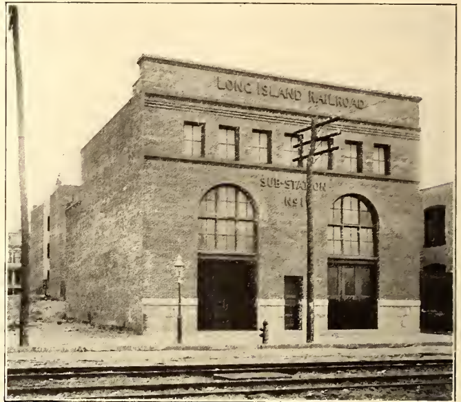
FIG. 4.—THE GRAND AVENUE SUB-STATION
