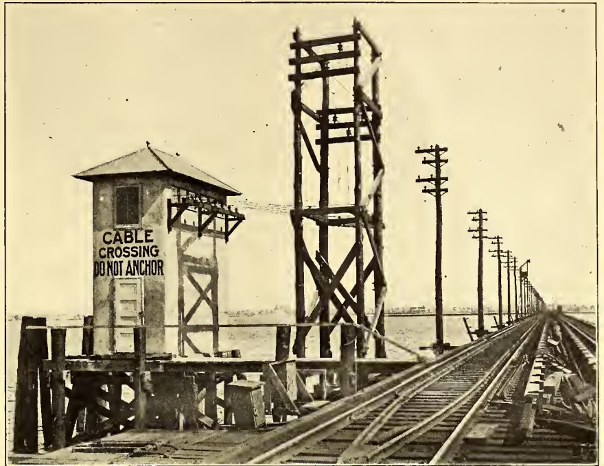
FIG. 8.—ARRESTER HOUSE AT BROAD CHANNEL DRAWBRIDGE
