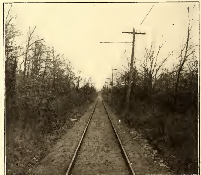
A TANGENT BETWEEN FARMINGTON AND FLAT RIVER, SHOWING HEAVY BALLAST
