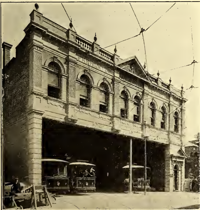
CAR HOUSE AND GENERAL OFFICES OF THE FREMANTLE MUNICIPAL TRAMWAYS
