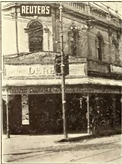
50-KW TRANSFORMER PLACED ON A TRAMWAY POLE IN FREMANTLE
