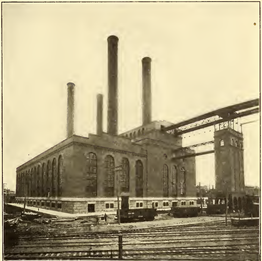
FIG. 2.—GENERAL VIEW OF POWER STATION AND ASH TOWER
