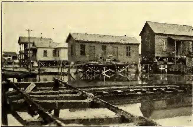
VIEW IN GALVESTON, SHOWING HOUSES AND TRACKS ON STILTS, READY FOR THE GRADE TO BE RAISED
