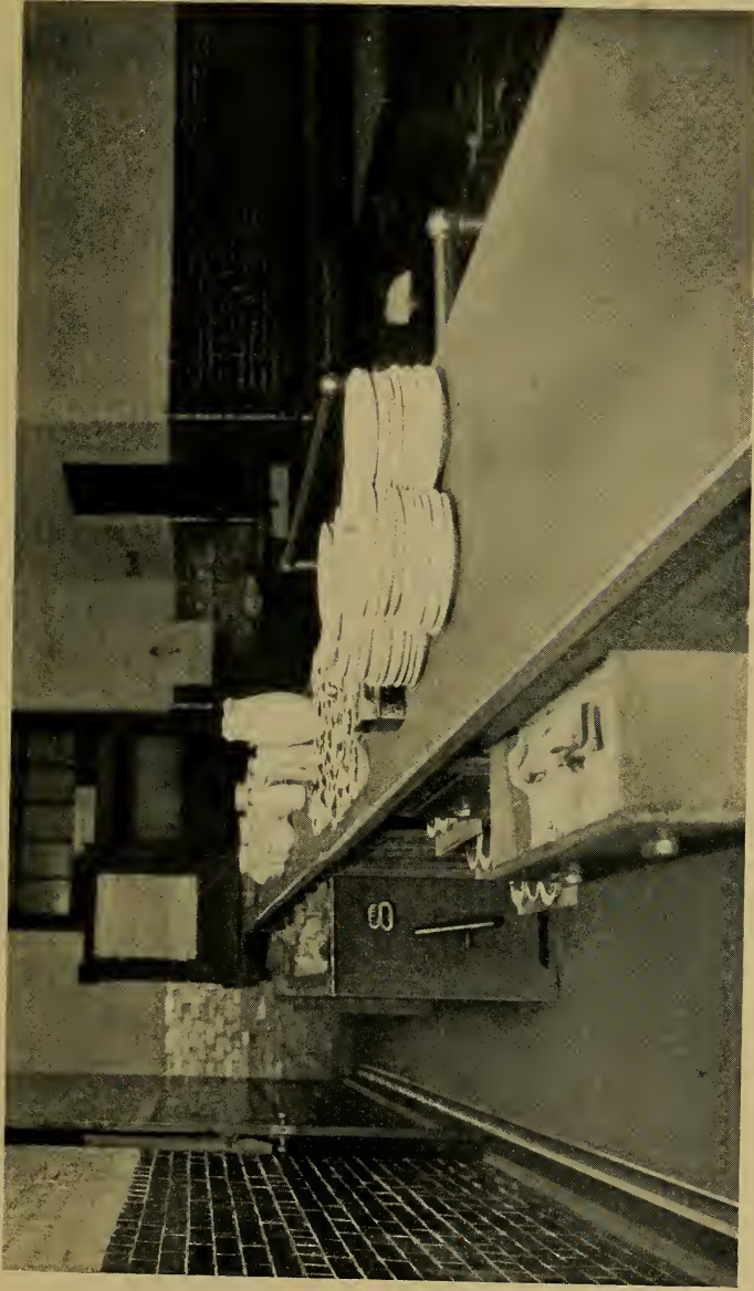
PLATE 9—SECTION OF COUNTER SHOWING SANDWICH DRAWER, DESSERT CLOSET WITH SHELVES DRAWN OUT AND ICE CREAM CABINET.
