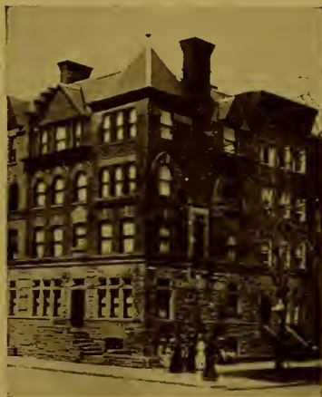
Houghton's City House
