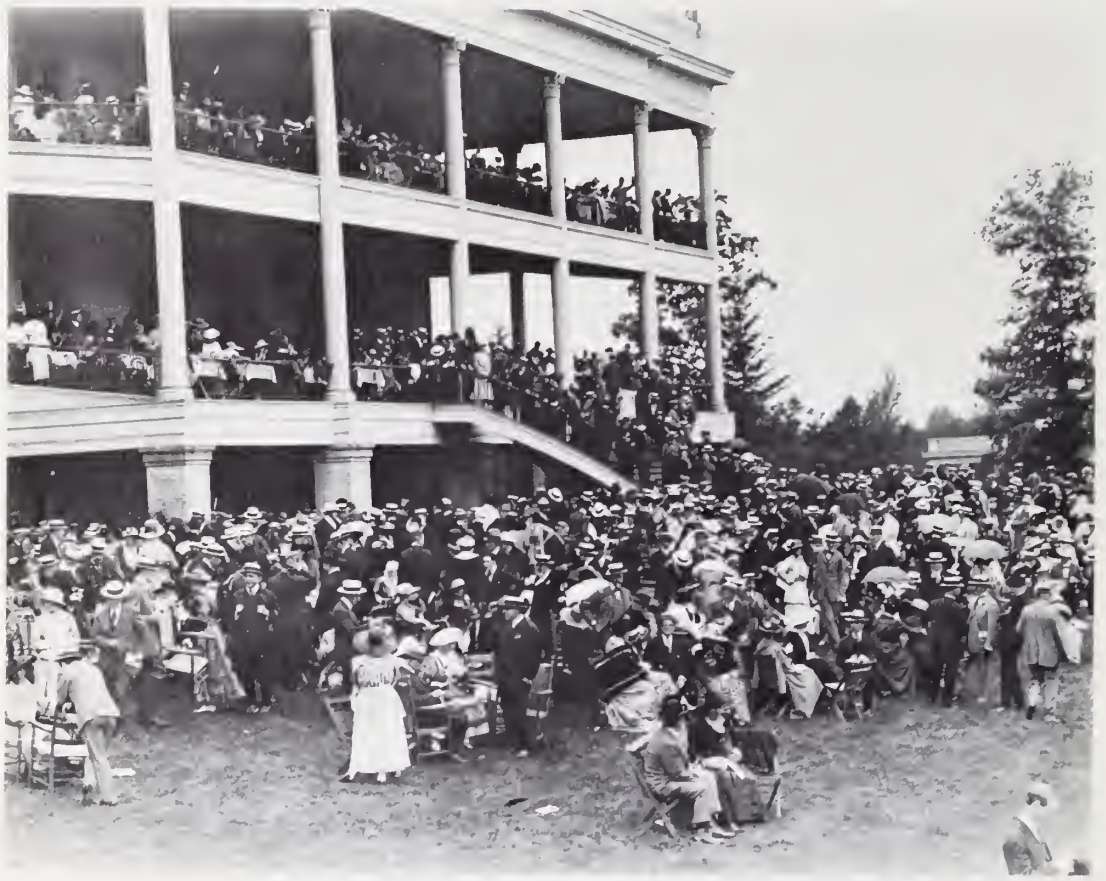
CLUBHOUSE SET: Belmont Park boasted a luxurious clubhouse with spacious private lawn. Here's balconied edifice, situated toward West end of track with finish line close by.
