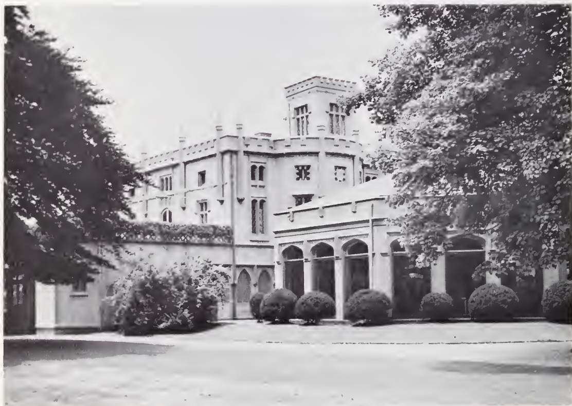
BEAUTY SPOT: Manice Mansion, bought at time parcel was assembled for building of original Belmont Park, became Turf and Field Club headquarters and flourished until mid-1950's.
