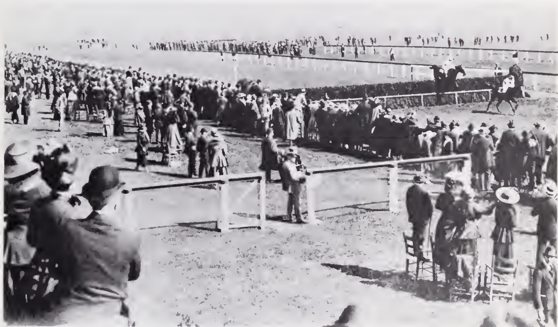
TERMINAL TRACK: 1916 scene at Belmont Park Terminal, steeplechase course used by United Hunts. Course was built at same time as Belmont Park main track across Hempstead Turnpike.
