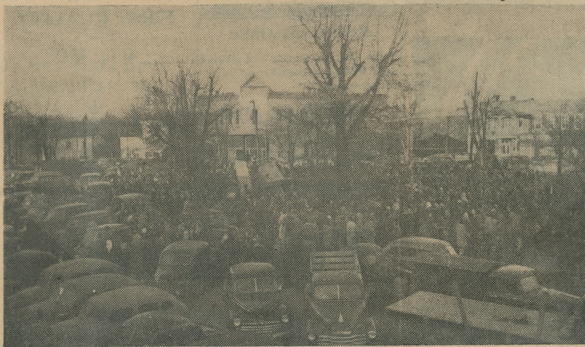
Photo taken from Reeves Building by Quality Photo Service
