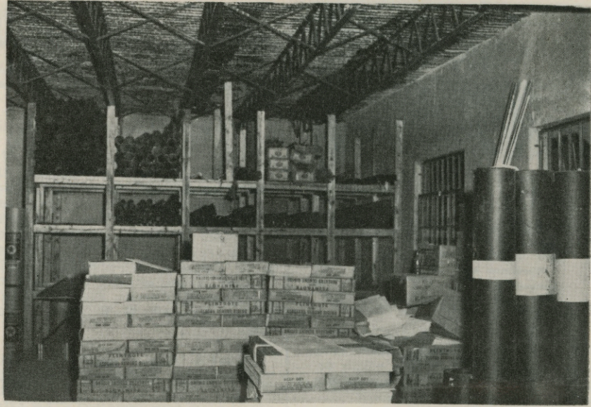
The new building that houses the Reeves Builders Supply Company in Clarkesville, Ga., is all of steel and masonry construction except for necessary displays and storage bins. The windows all have steel sash. Steel supports roof and second floor, as seen above. The building is 60 feet wide, the ground floor is 90 feet long, and the upper floor is 110 feet long. Built under Randolph Reeves' personal supervision and from his own plans, the building cost approximately $30,000.
