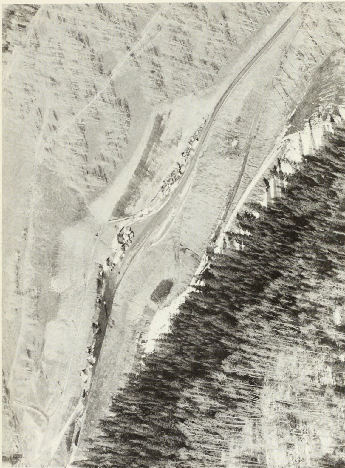
Figure 4.--Photograph showing Belina No. 1 portals and other surface facilities in Whiskey Gulch, Carbon County, Utah. Foreground is Conifer-Aspen type vegetation and background is Aspen type.
