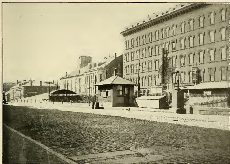
FIG. 32.—PRESENT SUBWAY OUTLET AT MAVERICK SQUARE.
