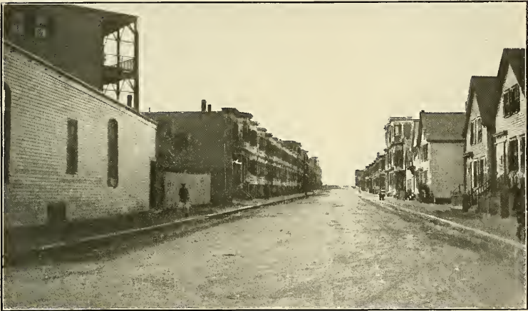
FIG. 7.— WORDSWORTH STREET, FROM SARATOGA STREET, LOOKING NORTH. Roadway little used; street treeless and desolate.
