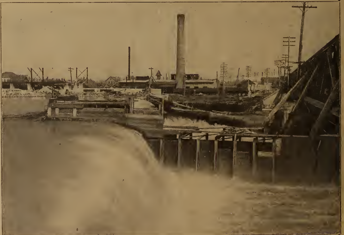
GREAT DAM OF CHICAGO SANITARY CANAL AT JOLIET
