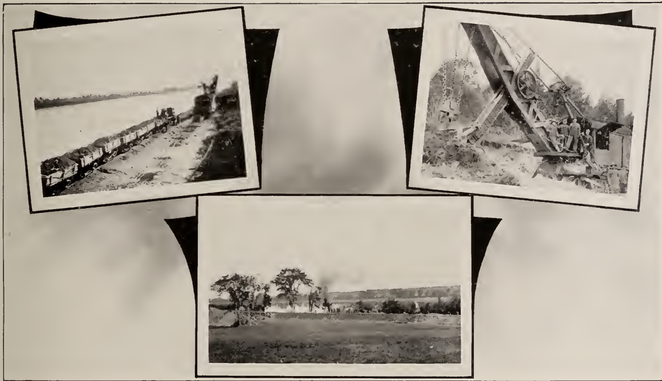
Construction Scenes near Fredericton on the St. John Valley Railway.
