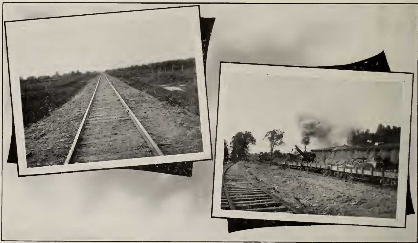
Construction Scenes on the Fredericton and Grand Lake Railway.
