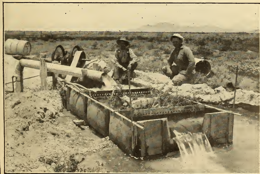
B. PORTABLE WEIR BOX IN USE.
