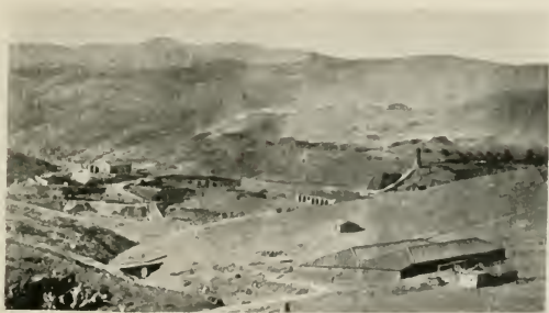
CEMENTATION VATS, HUELVA.
