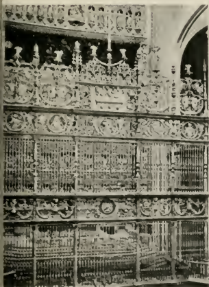
FIFTEENTH CENTURY GRATING, SEVILLE CATHEDRAL.
