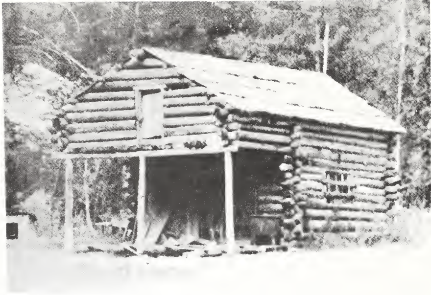
Fig. 15. Wyle's ranch, Payette National Forest, Idaho. Note 1\frac{1}{2} story height of cabin and stove under extension (from John Hartung).
