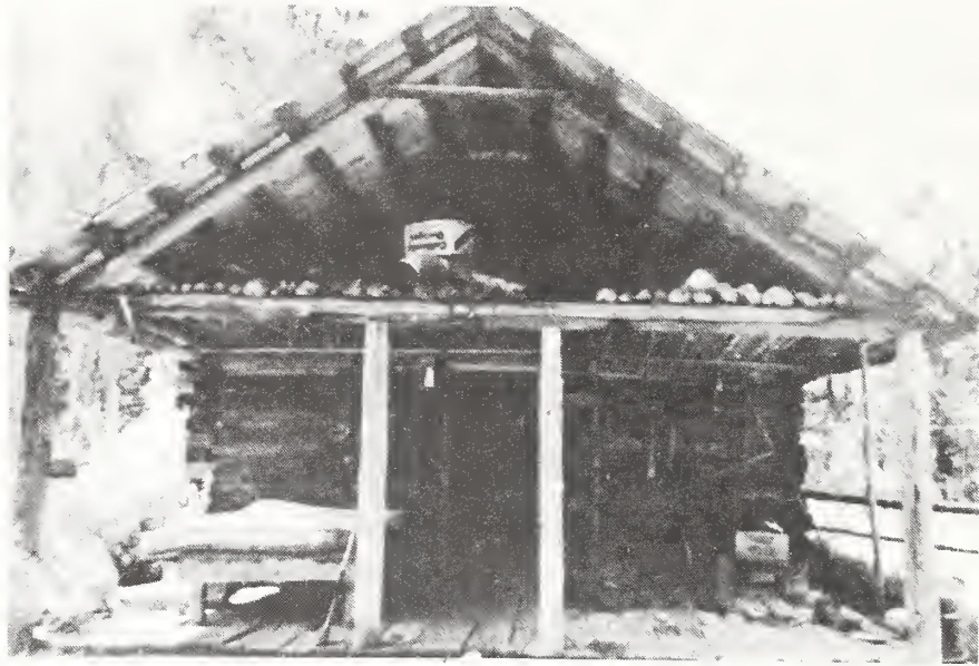
Fig. 10. Simond's cabin, Payette National Forest, Idaho. Note bed on porch and gable extension opening to the outside; typical of miner's cabin during summer occupation (from Hartung, 1978).
