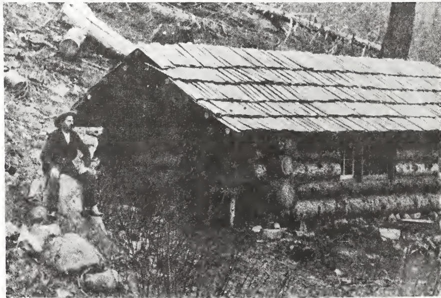
Fig. 31. Hopkin's cabin, Middle Fork of the Salmon River, Idaho. Photo taken ca. 1910, note large size of logs used in cabin's construction and small stool under gable extension (from Carrey and Conley, 1977).
