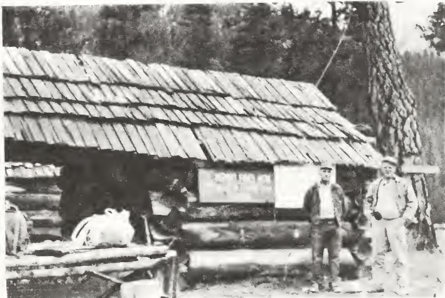
Fig. 7. Rocky Mountain Cabin with a gable extension nearing 100% the length of the actual cabin; a Forest Service structure from ca. 1930 (from Carrey and Conley 1977).
