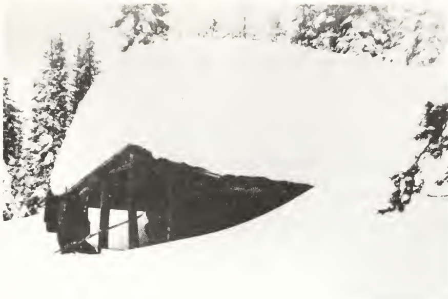
Fig. 12. 1880s miner's cabin, Boise National Forest, Idaho. Note accessibility provided by gable extension during heavy snowfall (from Jerry Wylie).
