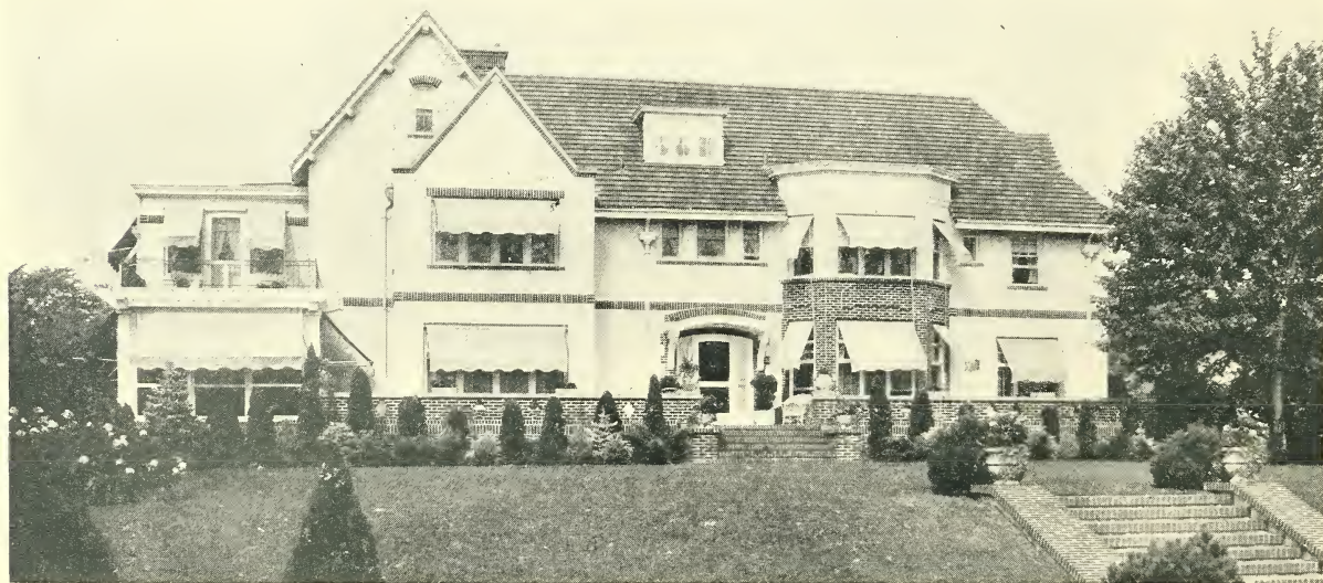
Effective planting is the result of careful planning. An example of some of the work we do.
