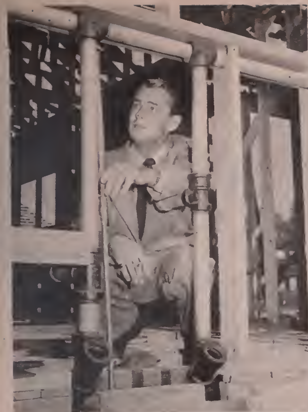
Copper pipes leading to the kitchen get Alan's close attention as do all other building details.
