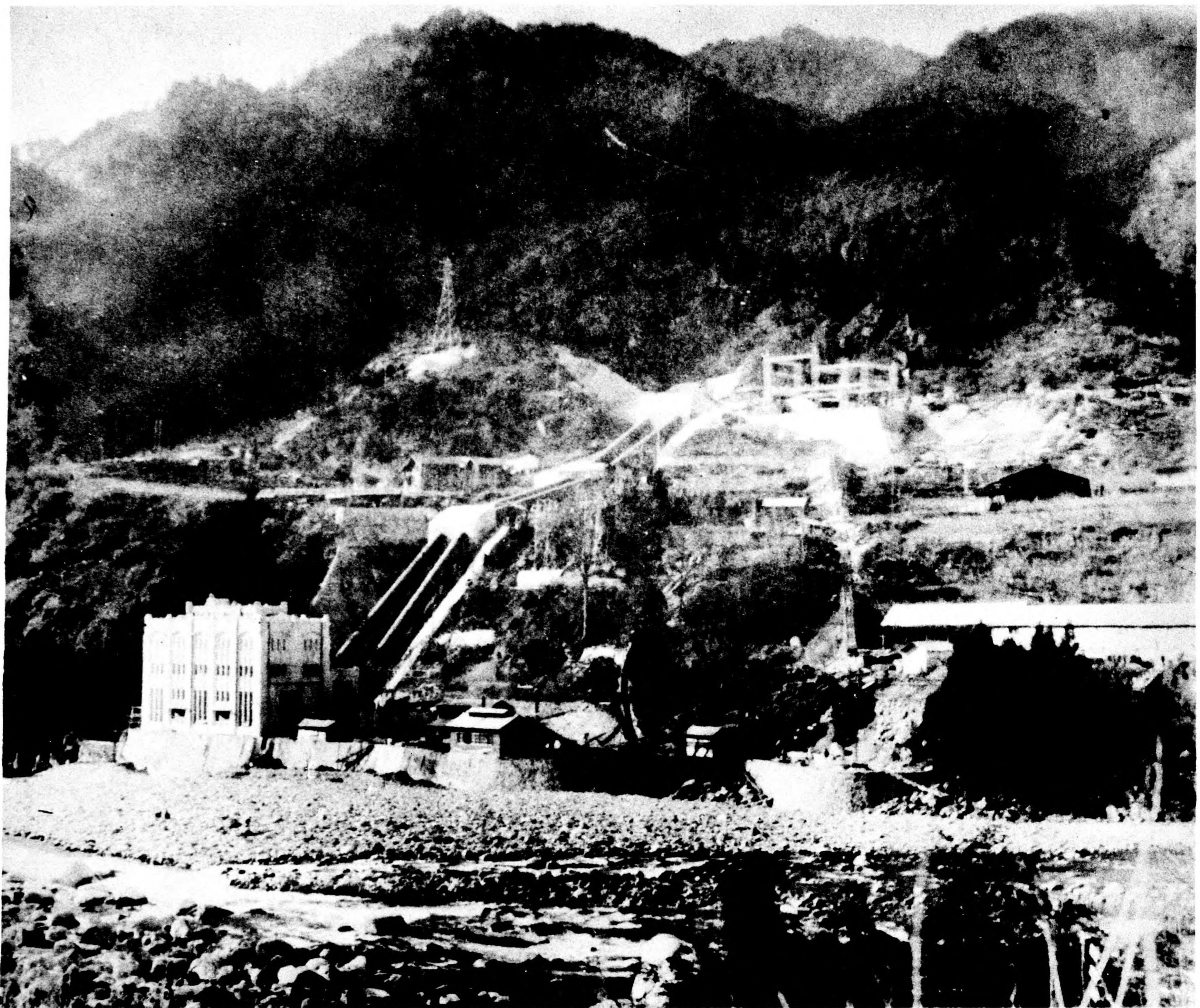
Photograph No. III-114, Momoyama Hydro Plant before construction of auxiliary building
