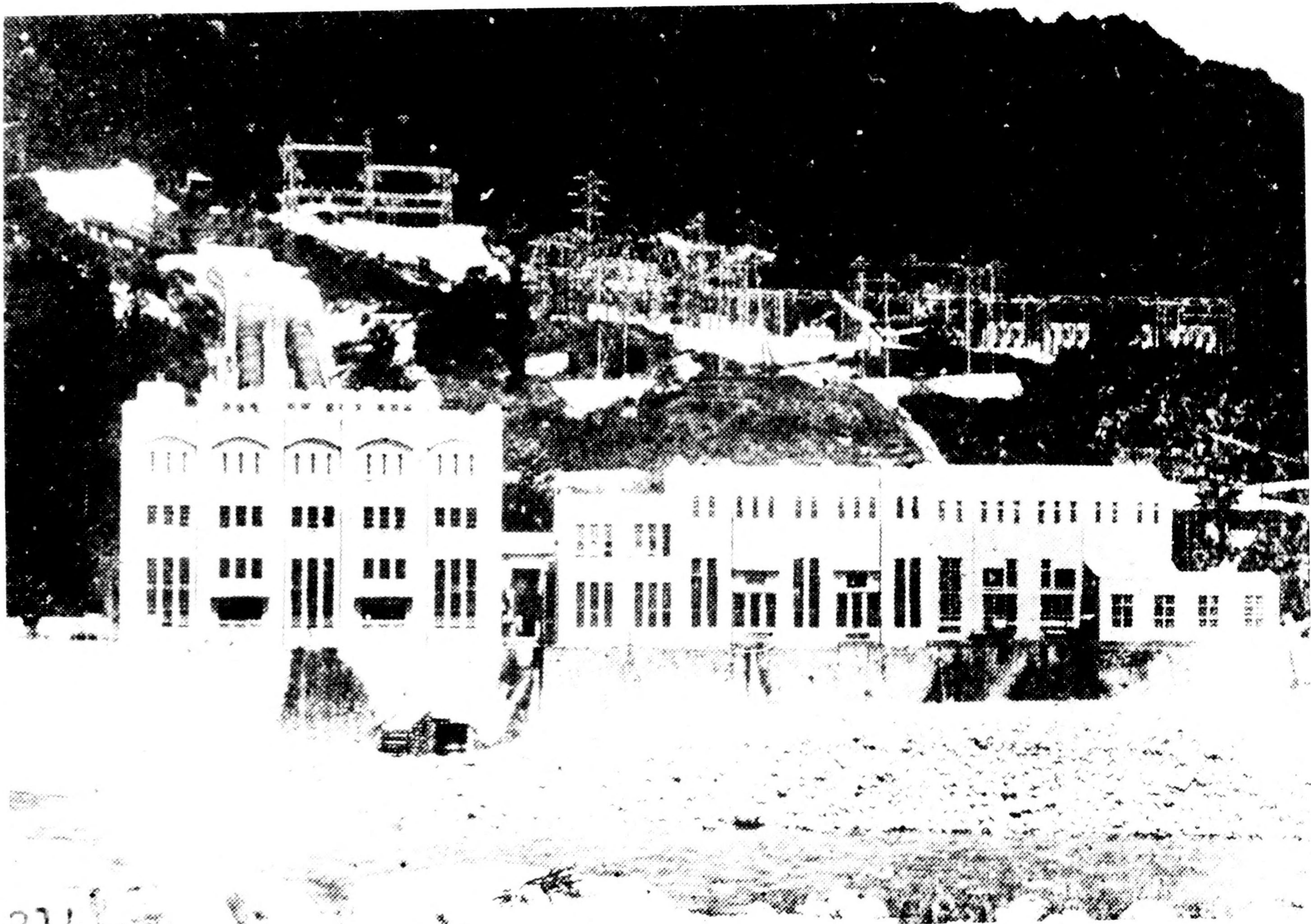
Photograph No. III-115 Momoyama Hydro Plant with auxiliary building
