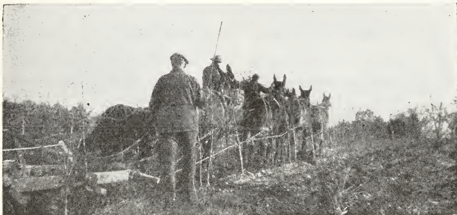
Tree Digger at Work
