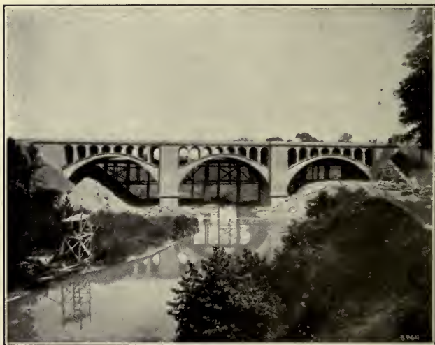
THE CONCRETE BRIDGE ON A LARGER SCALE
