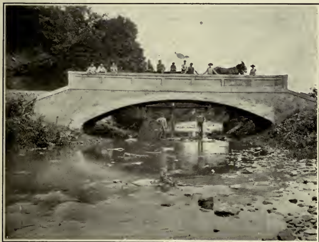
THE MODERN CEMENT BRIDGE ON COUNTRY ROAD
