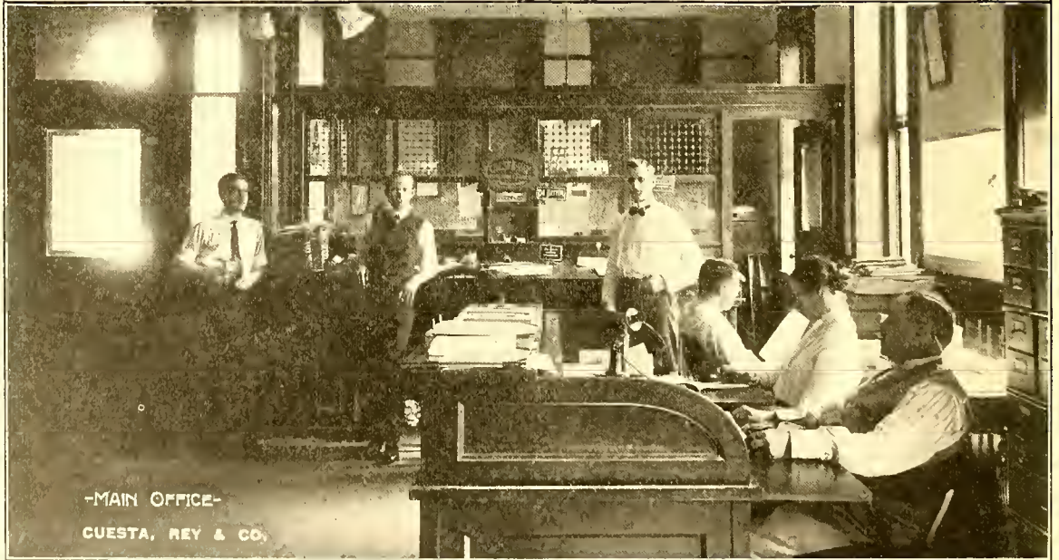
OFFICE AND EXTERIOR VIEW OF FACTORY
