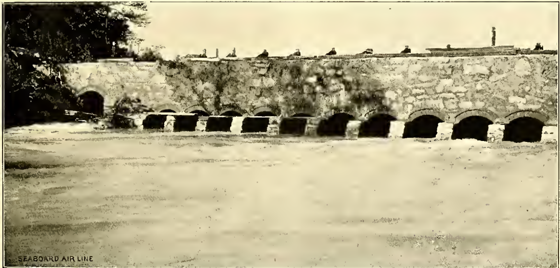
BULKHEAD ENTRANCE OF WATER FROM DAM INTO ROANOKE RAPIDS CANAL ON S. A. L. RAILWAY.
