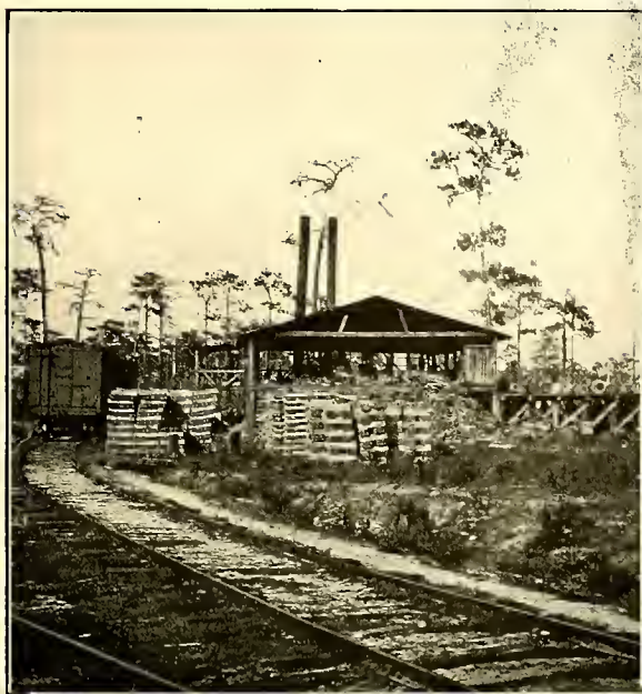
TYPICAL SHINGLE MILL IN THE RURAL DISTRICTS OF FLORIDA, S. A. L. RY.
