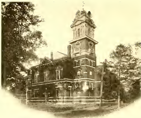
GWINNETT COUNTY COURT HOUSE, LAWRENCEVILLE, GA., S. A. L. RY.
