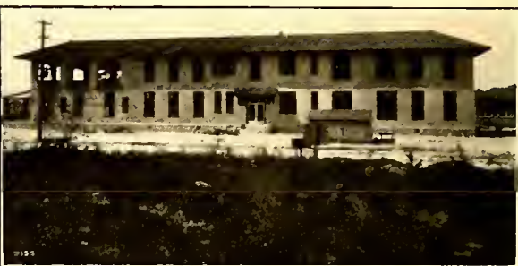
ST. LUKE'S HOSPITAL JACKSONVILLE, FLORIDA Edward F. Stevens Mellen C. Greeley Associate Architects
