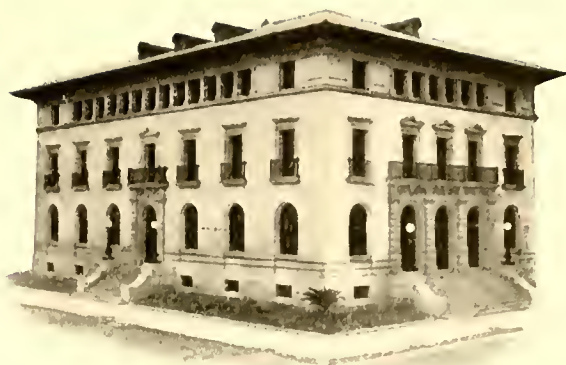
ONE OF FERNANDINA'S MANY ADORNMENTS. THIS COMMODIOUS STRUCTURE, WHICH IS THE NASSAU COUNTY COURT HOUSE, UNITED STATES CUSTOM HOUSE AND POST OFFICE, IS ONE OF THE MANY ATTRACTIONS AT FERNANDINA, FLA., ON THE S. A. L. RY.
