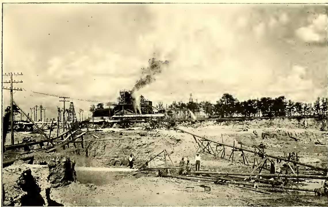
HYDRAULIC PHOSPHATE MINING IN FLORIDA ON S. A. L. RY.
