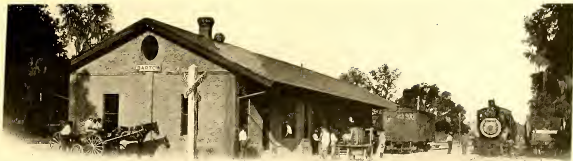
THE NEW S. A. L. RY. PASSENGER DEPOT, BARTOW, FLA. THE POINT TO WHICH THIS SYSTEM WAS RECENTLY EXTENDED.
