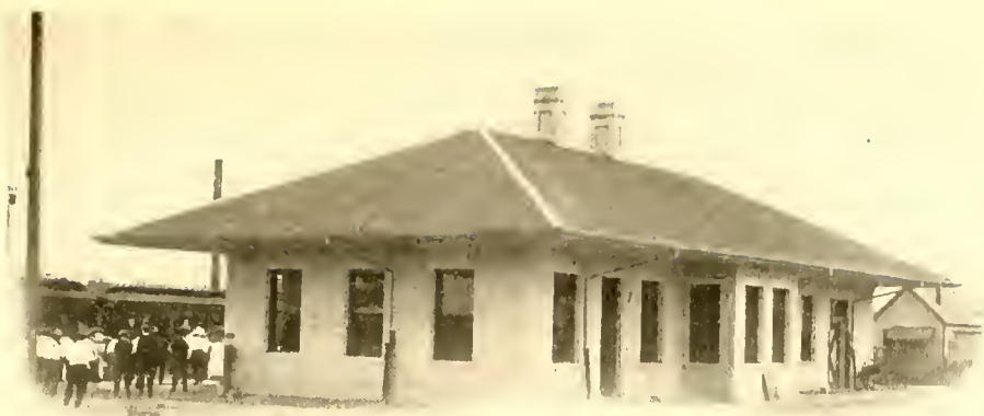
NEW UNION PASSENGER STATION AT OCILLA, GA., ON THE S. A. L. RY.
