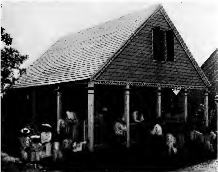
FIG. 2.—TEMPORARY DISPENSARY AT CURRENT SETTLEMENT, ELEUTHERA
