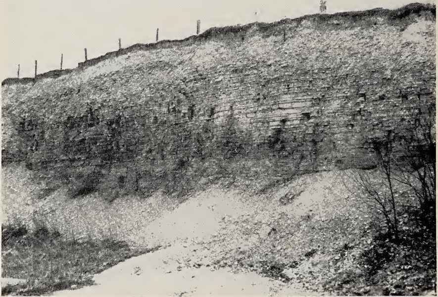
FIGURE 1. Road cut showing acid shale with overlying siltstone and capped by eolian material. (Pierce County, Wisconsin)
