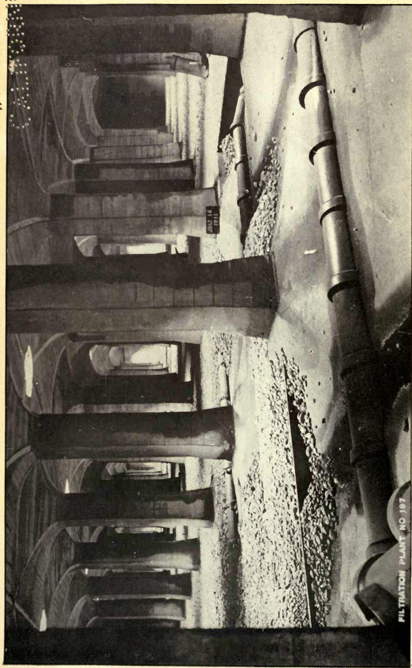
TORONTO FILTRATION PLANT.—INTERIOR OF FILTER, SHOWING UNDER-DRAINS AND FIRST GRAVEL LAYER.
