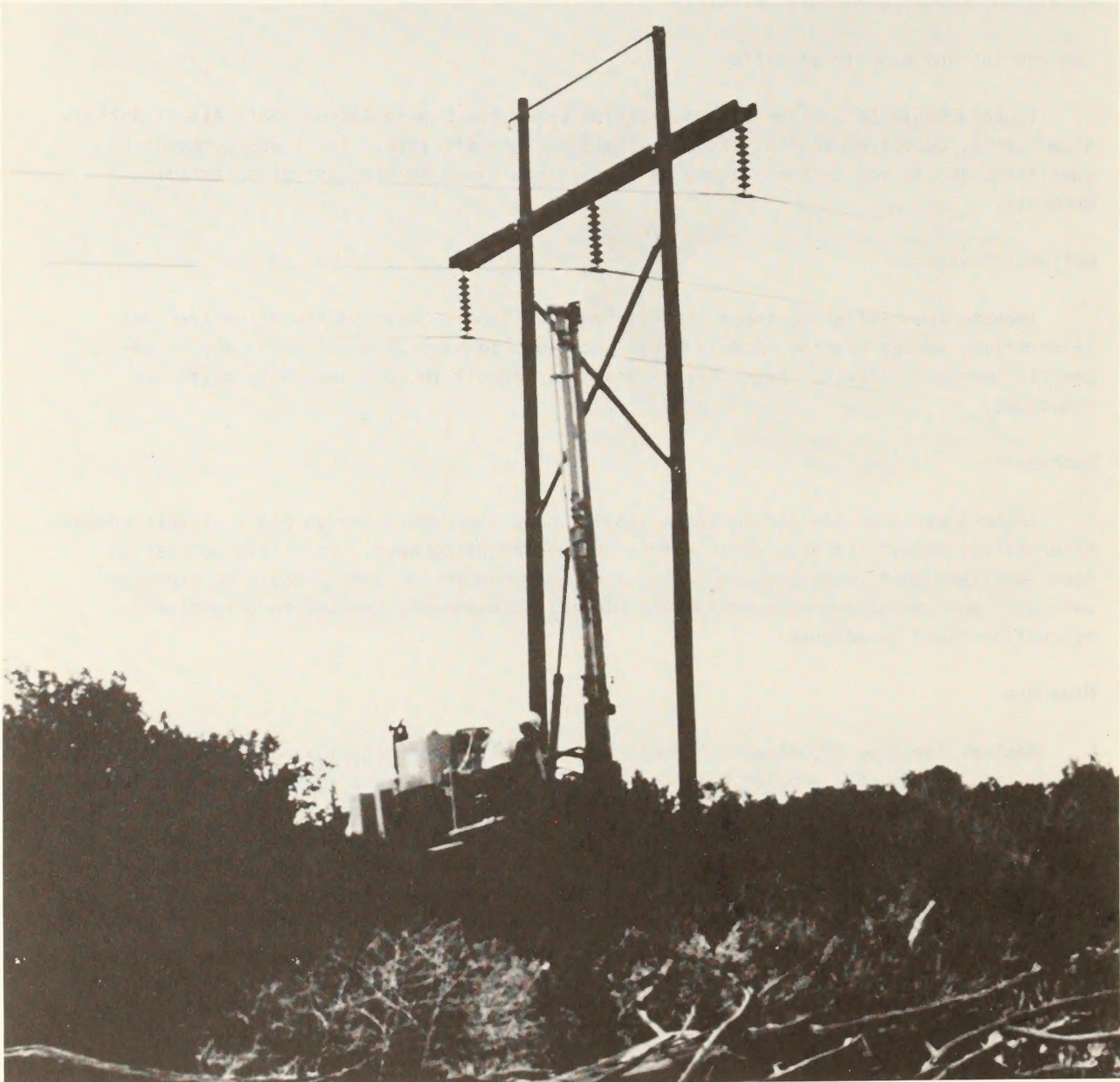
TYPICAL 115-KV POWERLINE.
