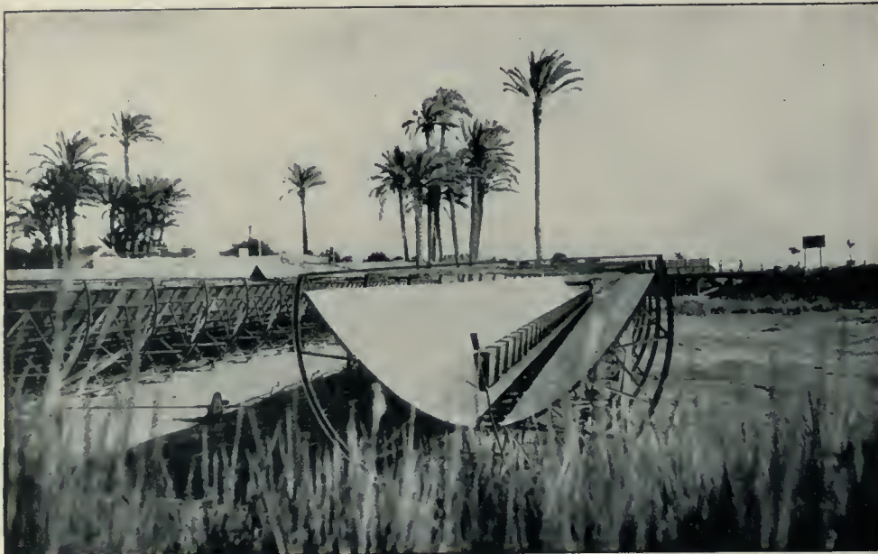
FIG. 47.—SHUMAN-BOYS ABSORBER, MEADI, 1913. ONE SECTION OF THE ABSORBER FROM THE NORTH.
