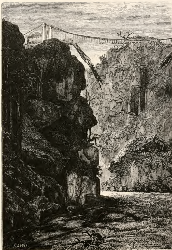
THE BRIDGE, COMPLETELY RUINED, FELL WITH A CRASH.
